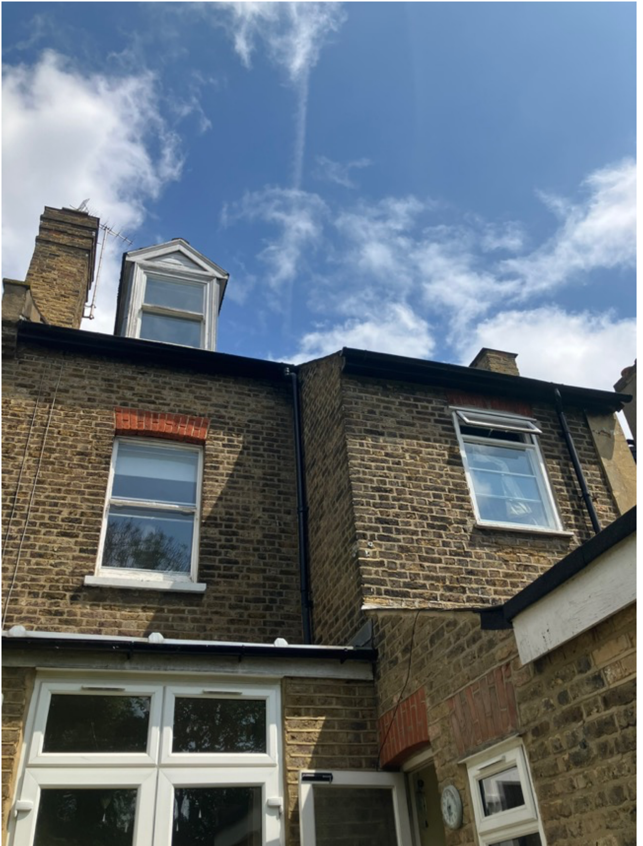
No.13 Western Road Rear Elevation
