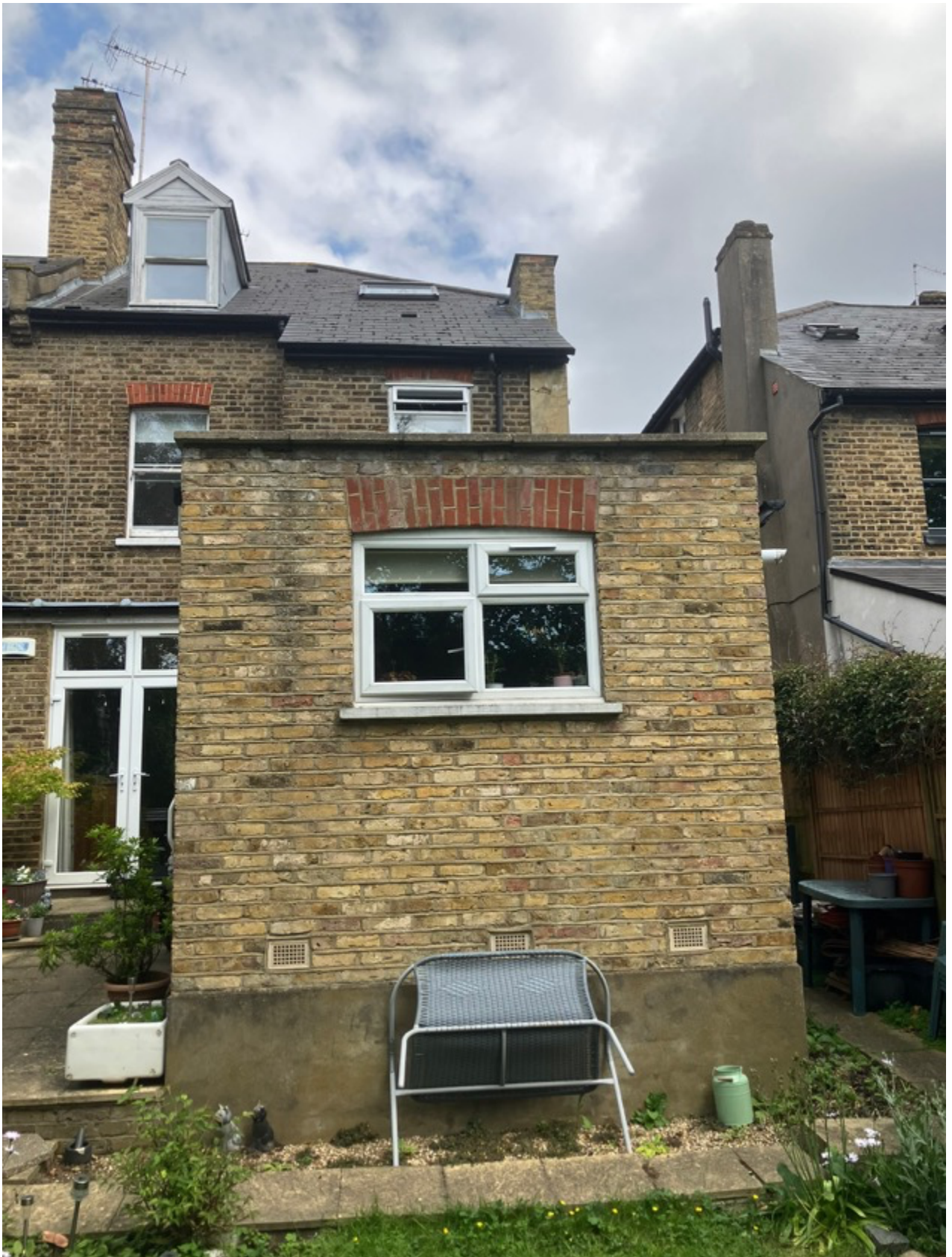
No.13 Western Road Rear Elevation
