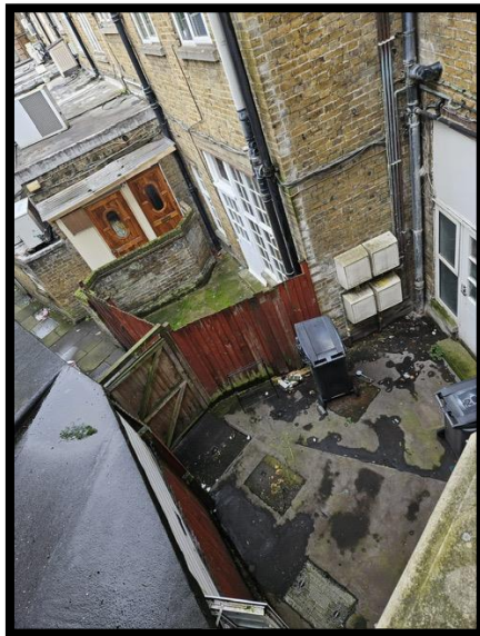
Figure 1 Yard to rear of Application site providing safe storage for refuse and recycling bins
