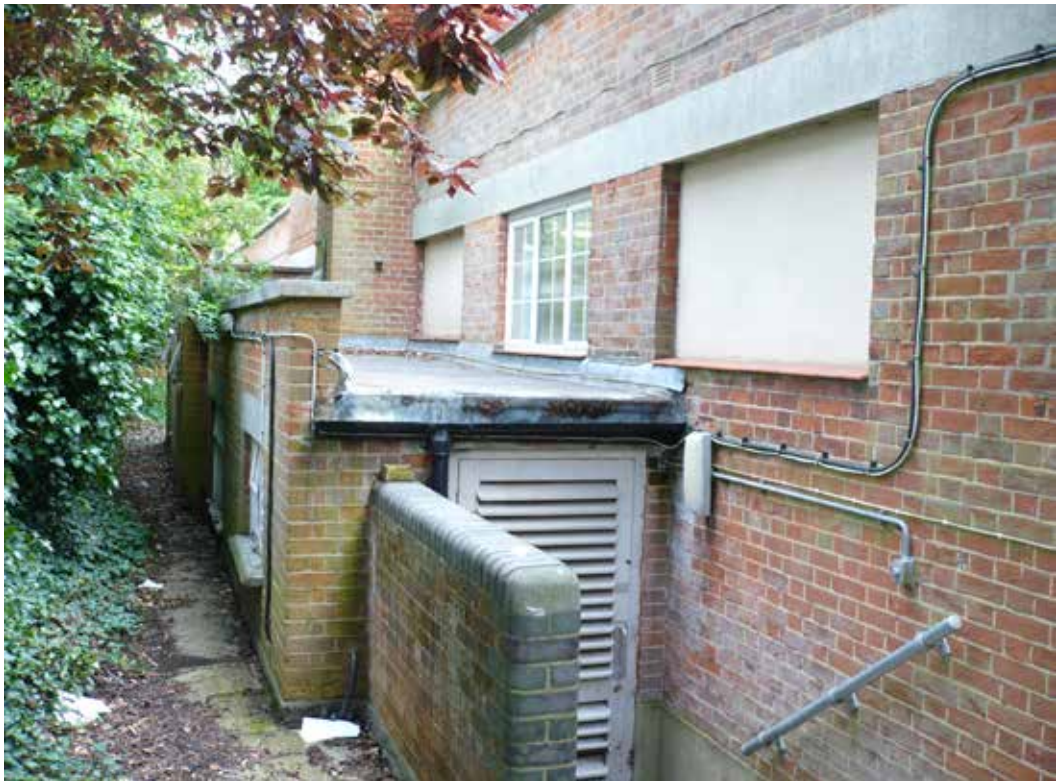
4. Stairs into the plant area at the rear
