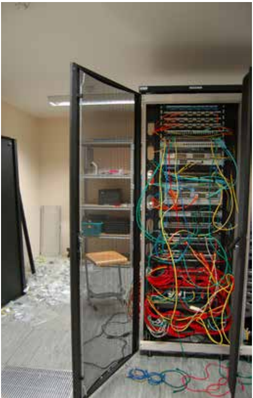
Existing IT Hub
