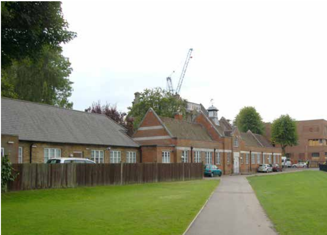
1. Approach via pedestrian path from Senior School to RMC building
