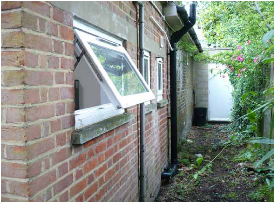
3. Service area to the rear
