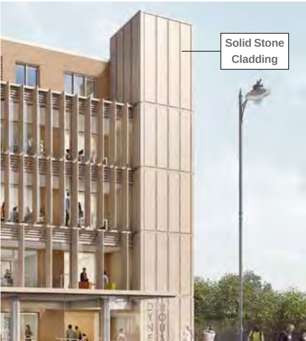
Stone Cladding on Lift Shaft
