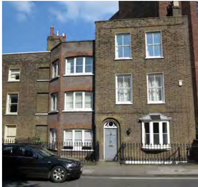
5. No.16 Southwood Lane
