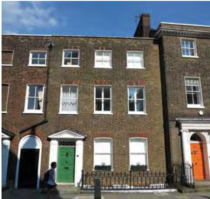
6. No.8 Southwood Lane
