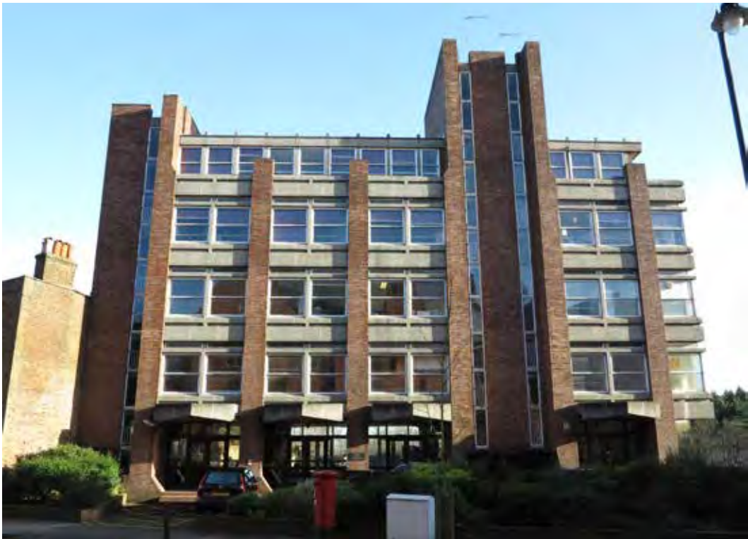
1. Southwood Lane entrance to Dyne House
