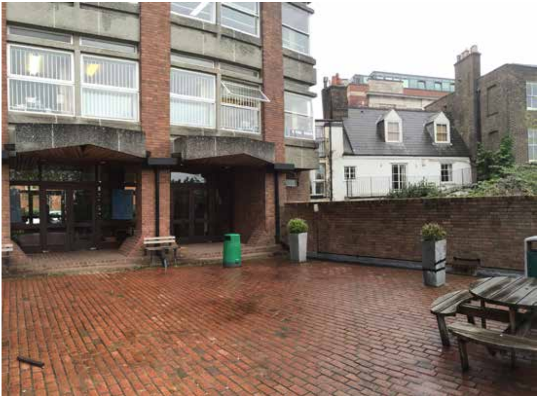
3. External Seating Area at the rear of Dyne House
