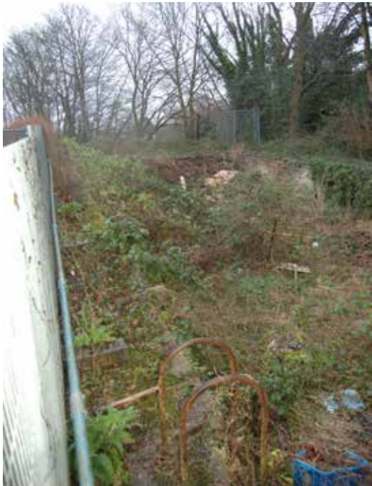
2. The redundant open air swimming pool
