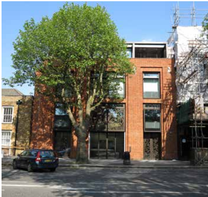
3. The New Teaching Building 2012
