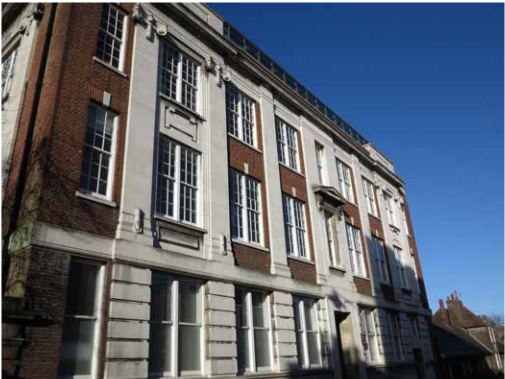
Stone & Brick Facade
