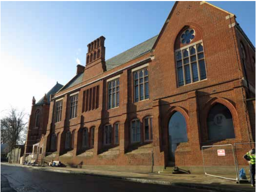
Relief and depth within the brick facade
