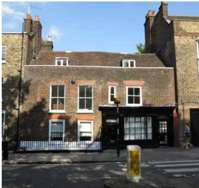
4. No. 2 Southwood Lane
