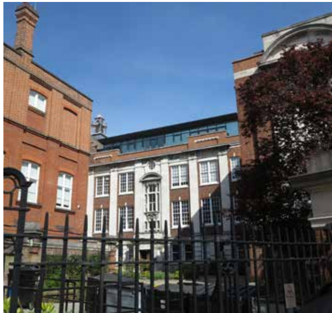
2. The Science Building 1928
