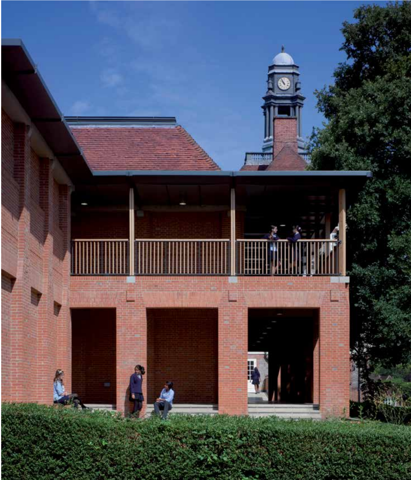
The Henrietta Barnett School, London, Hopkins Architects
