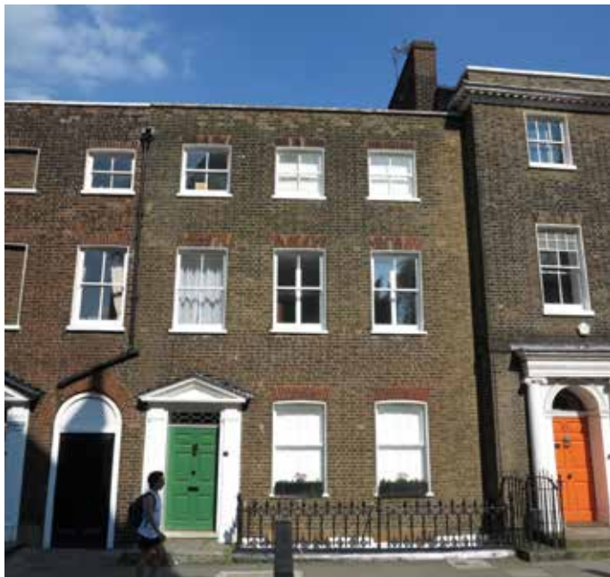
6. No. 8 Southwood Lane
