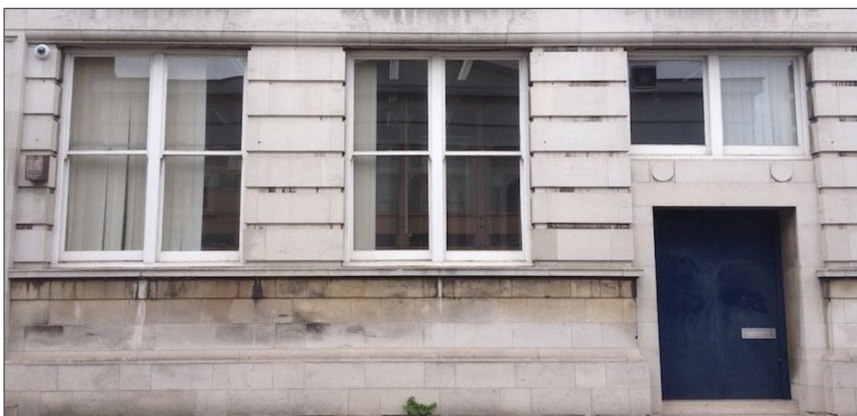
Detail view of the east elevation of East Wing from Southwood Lane
