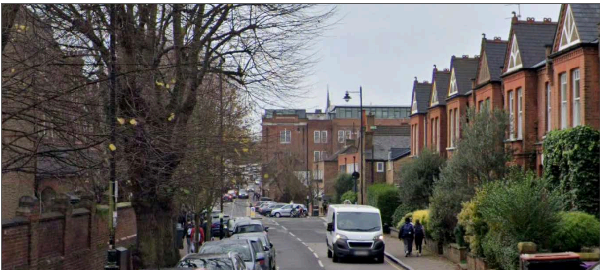
Existing view of Science building from Southwood Lane - from north
