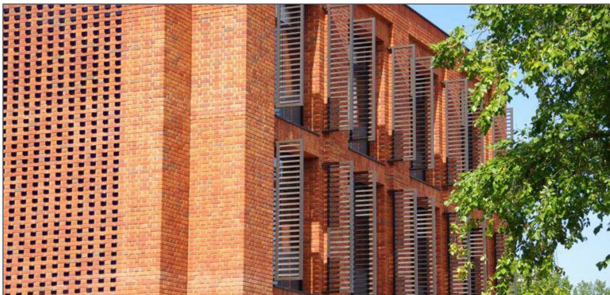
Photograph of existing Charter building rear privacy screens
