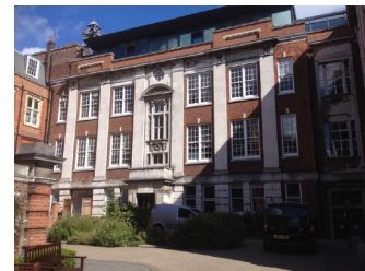
Exterior view of the south elevation in Science Quad
