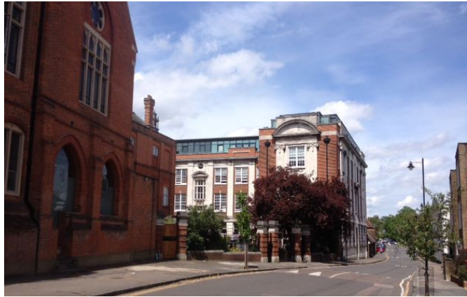
Street context: view of the Science Building from the south along Southwood Lane
