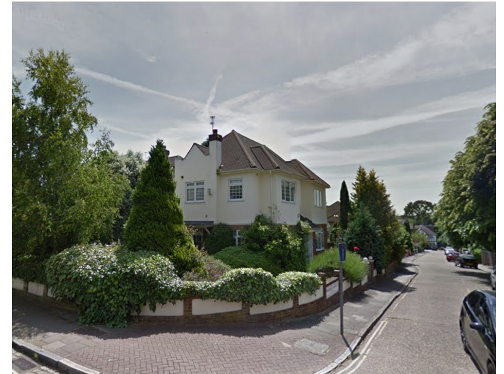
Existing Site Image 2
