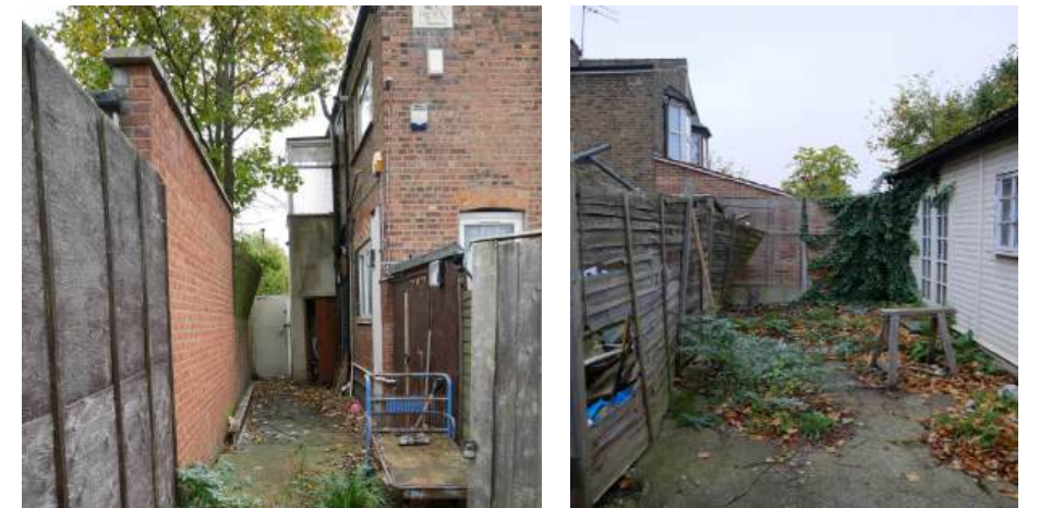
15. View showing side of site and east boundary and View of rear building and garden
