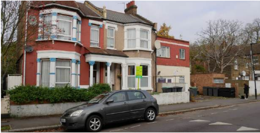
9. View from Raleigh Road including adjacent semi-detached houses
