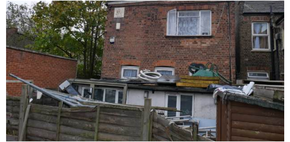
13. View of rear of main building
