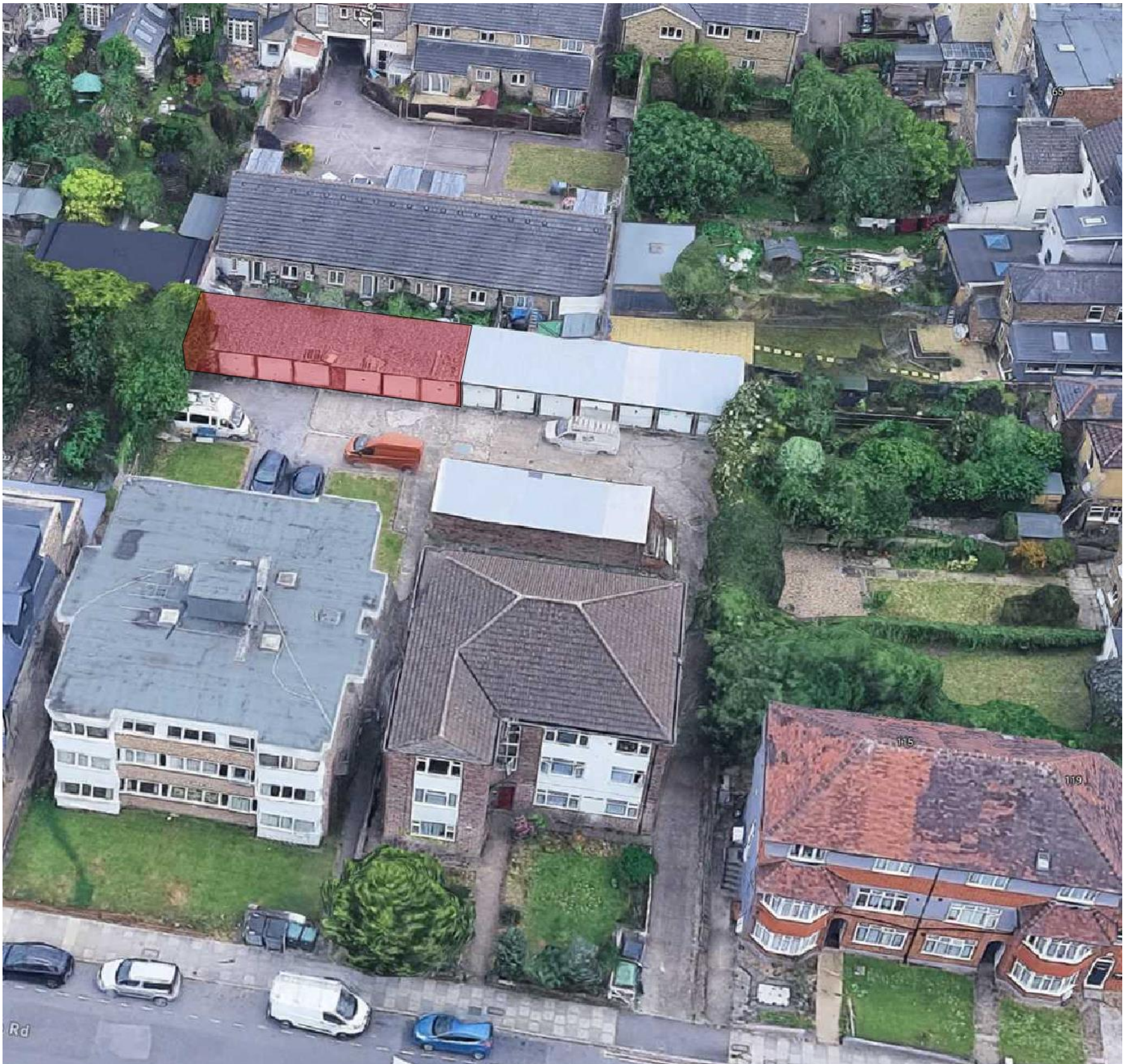
Aerial photo of site with private side access road and Avondale & Richard Courts adjacent.
