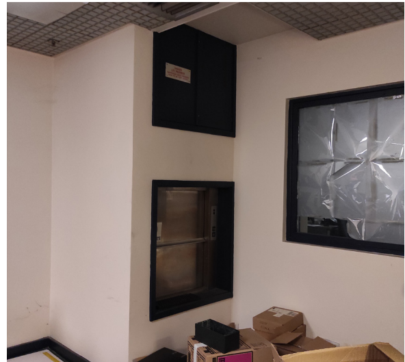
Figure 2: Dumbwaiter in Old Cash Office
