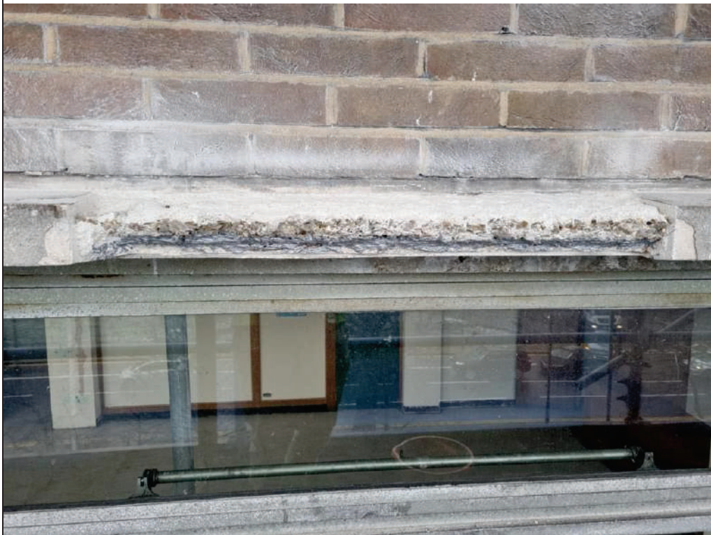
Pre-cast Window Head Repair – Defective Rebar rubbed back by mechanical means and treated with Fosroc Galvafruid
