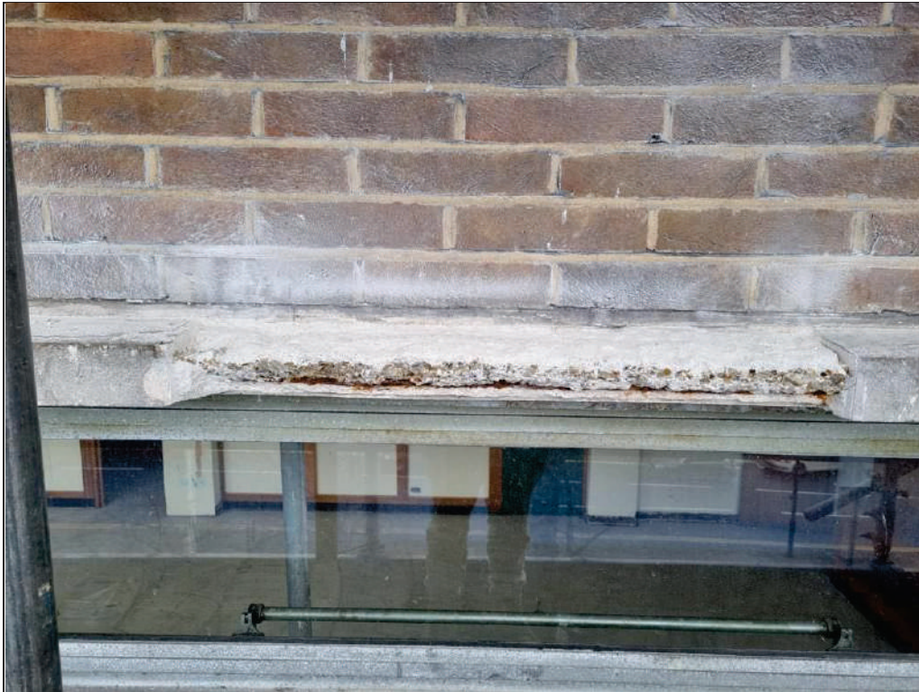
Pre-cast Window Head Repair – Defective pre-cast Removed
