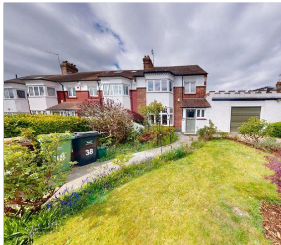
Existing Front facade
