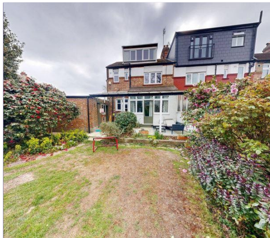
Existing Rear facade
