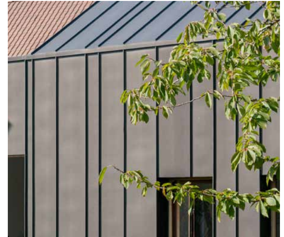
Fig.38- Pre-patinated zinc cladding to dormer wall and GFL extension roofing
