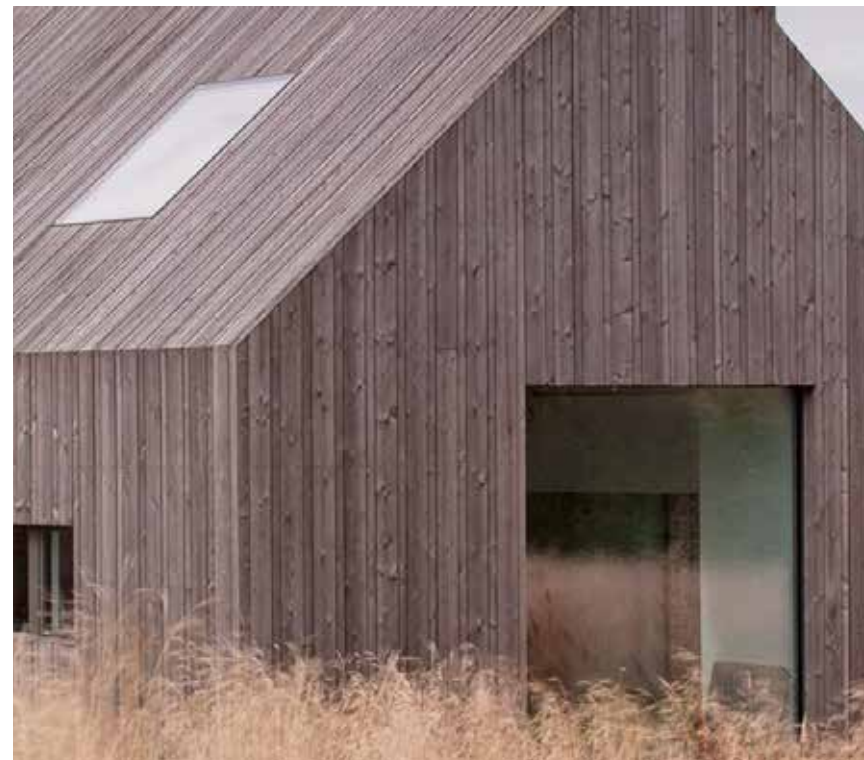
Fig.39- Timber cladding to wall and roof, flush glazing and gutters, weathered finish
