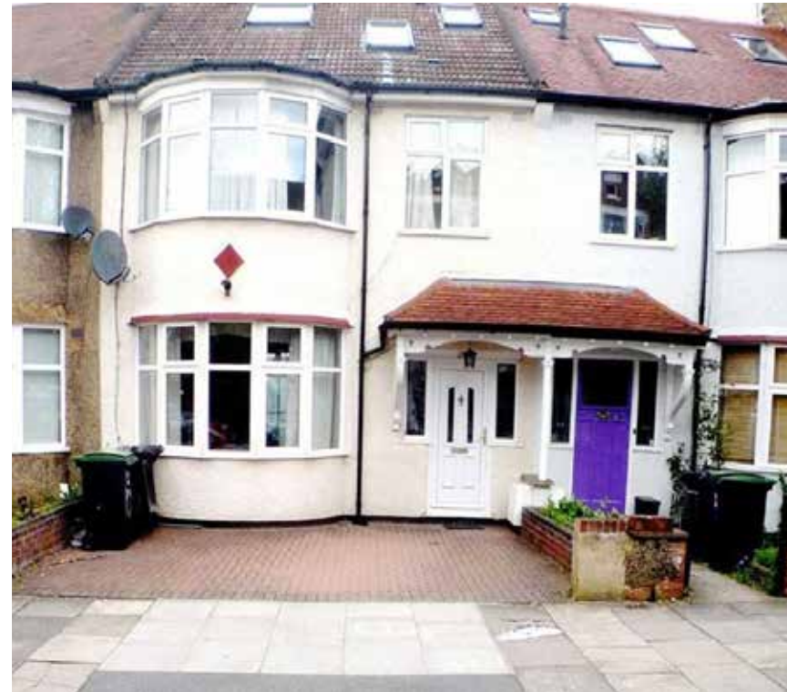
Fig.14- Street Elevation with Pebbledash painted render characteristic of 1930's dwellings
