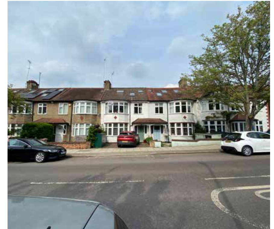
Fig.15- Front elevation is consistent with adjacent terraced houses also in 1930's style
