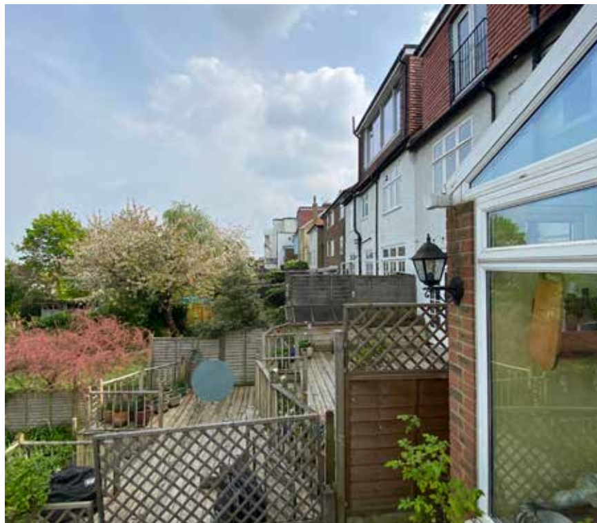
Fig.10- Adjacent terraces from rear, looking East
