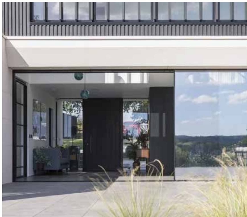
Fig.41- Powder coated Sliding door with slim profile frame
