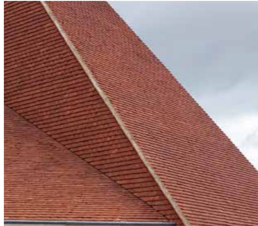
Fig.37- Existing original roof tiles to be maintained when roof upgraded and new tiles to align.
