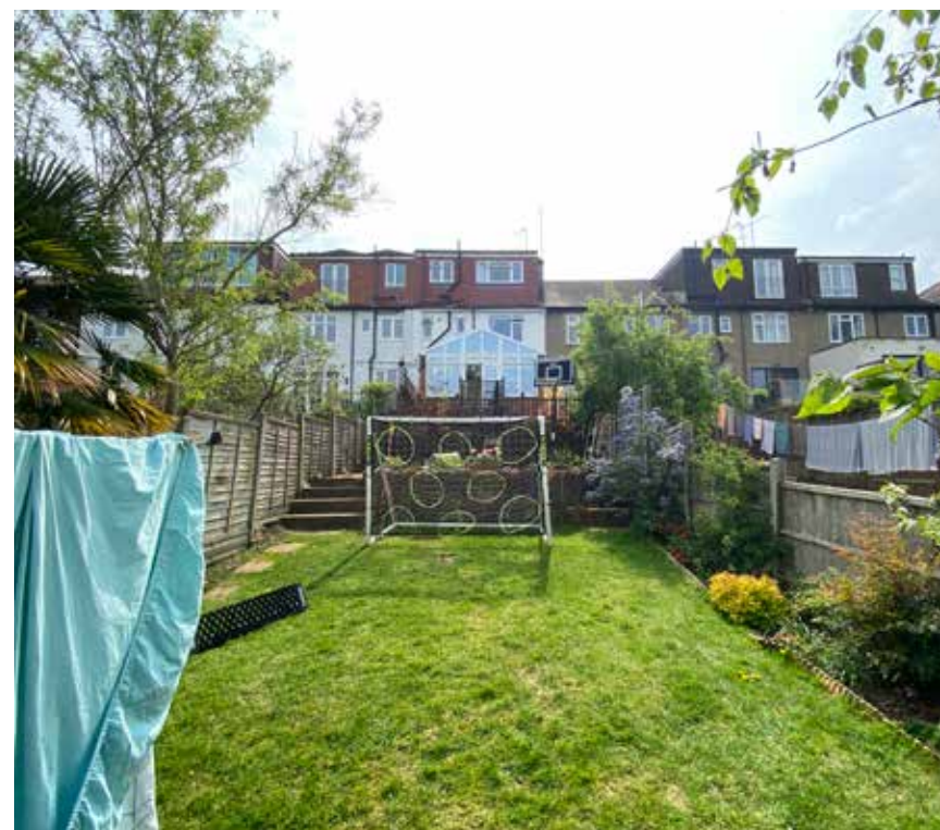
Fig.20- Overview of rear elevation of wider terrace, with flat roof dormers at 2FL level
