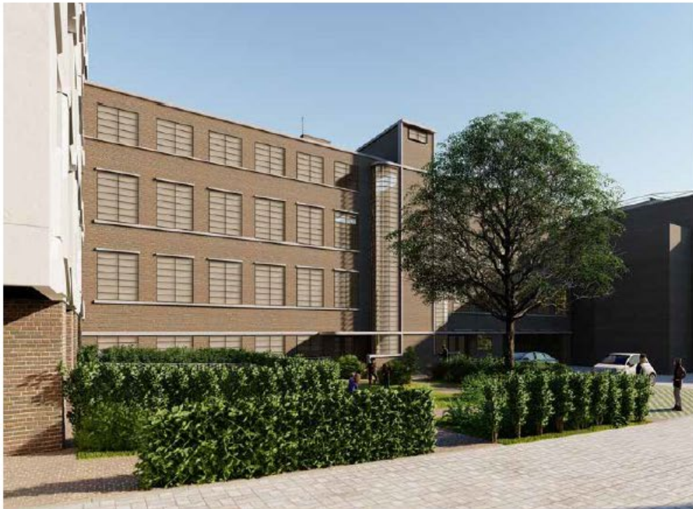
The plant equipment located on the East Wing is not visible from the public realm.
