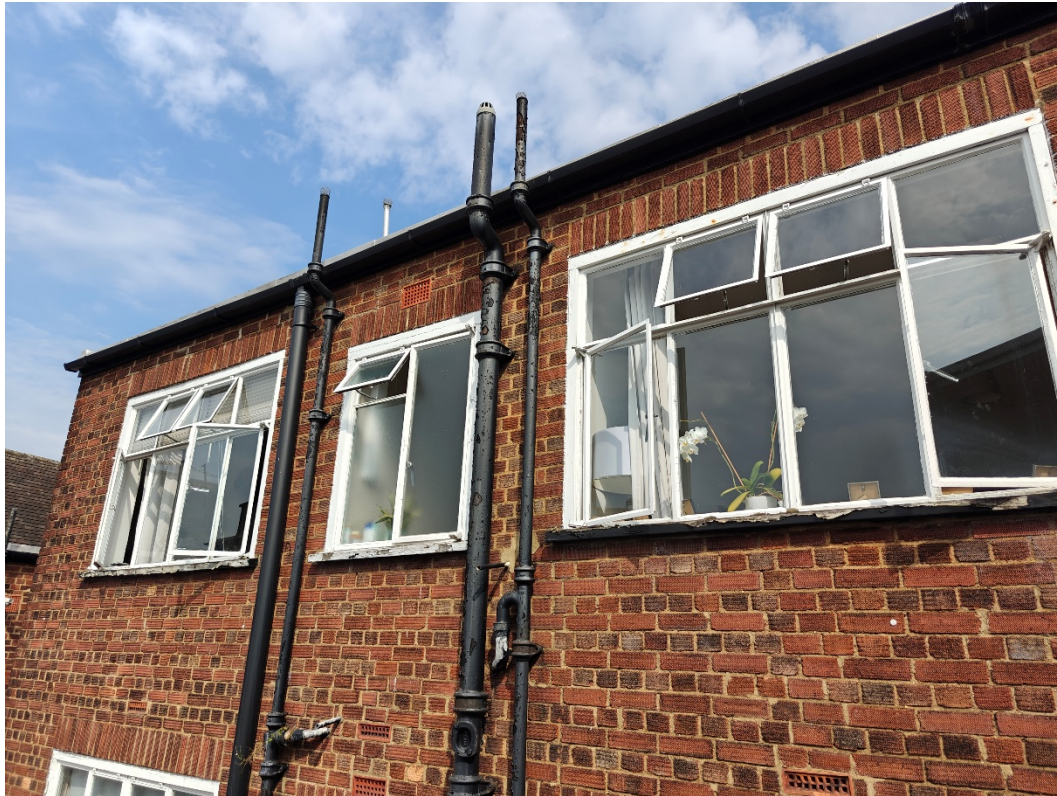
Figure 3 External view of the windows
