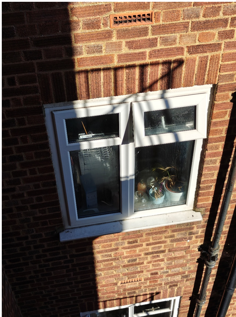
Figure 6 uPVC window installed in the block
