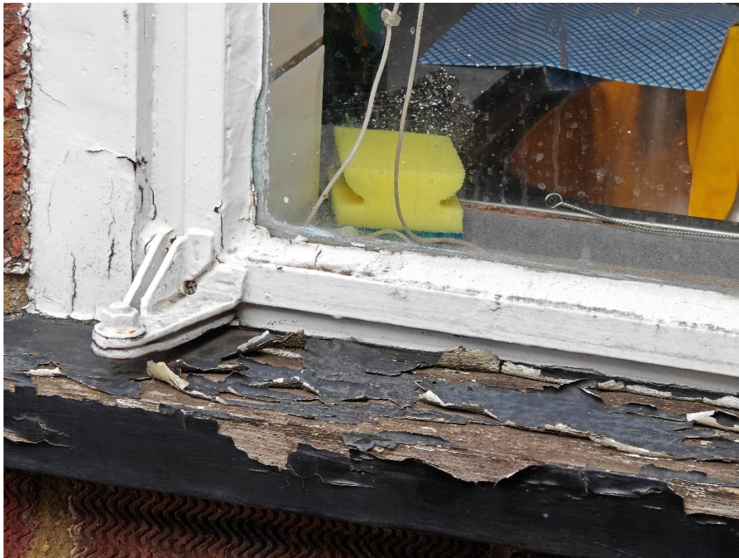
Figure 5 External detail with projecting hinge
