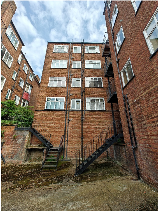
Figure 2 View of the South Elevation
