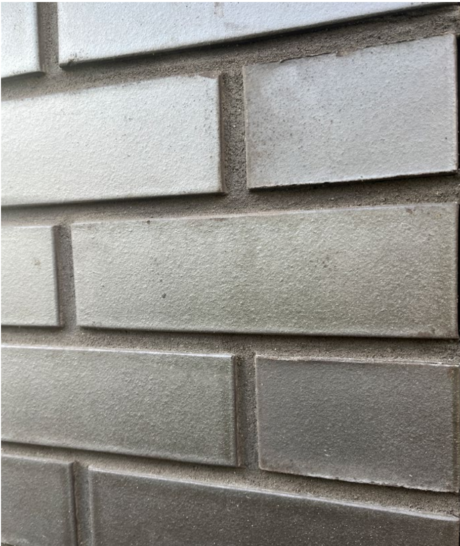
FIGURE 10. Brick Plinth - Approved Sample Panel
