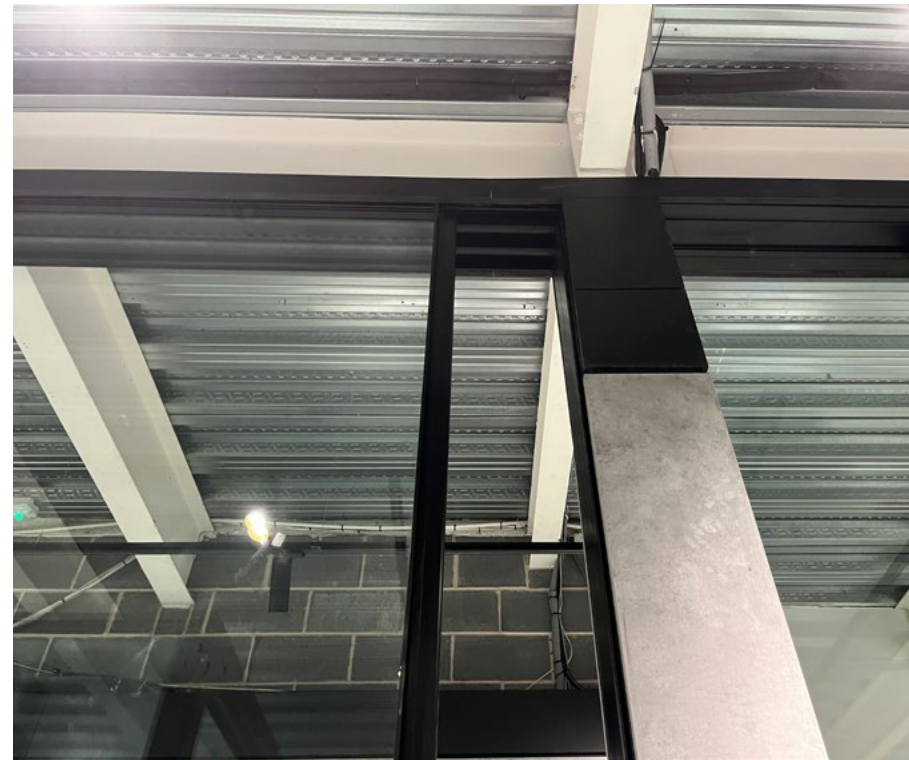
FIGURE 6. Fluid Glass - Sliding Door System - Head Detail
