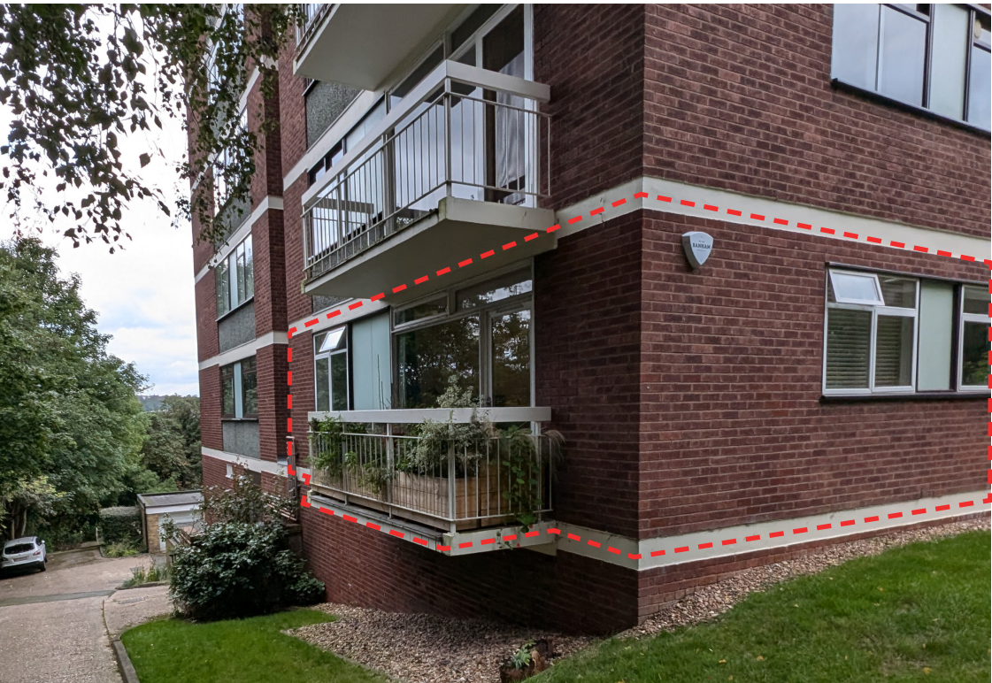
Photos of the building's façades Flat no.1 highlighted in red
