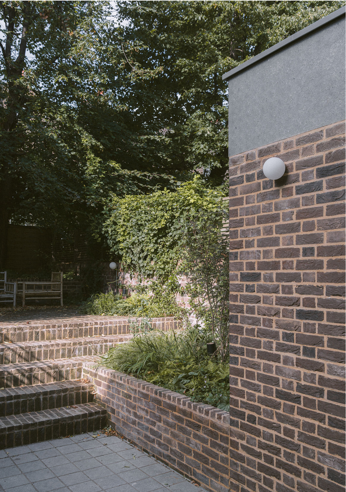
House in Islington, by Architecture for London/AFL Build
