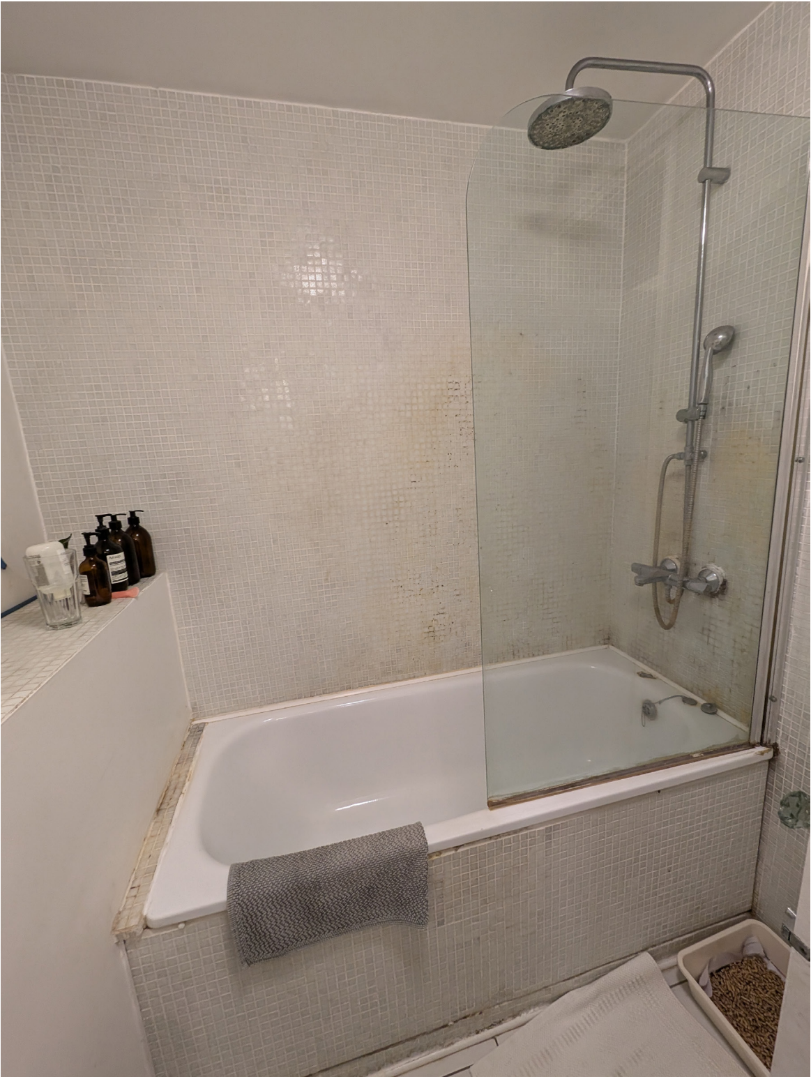
Photo of the existing bathroom
