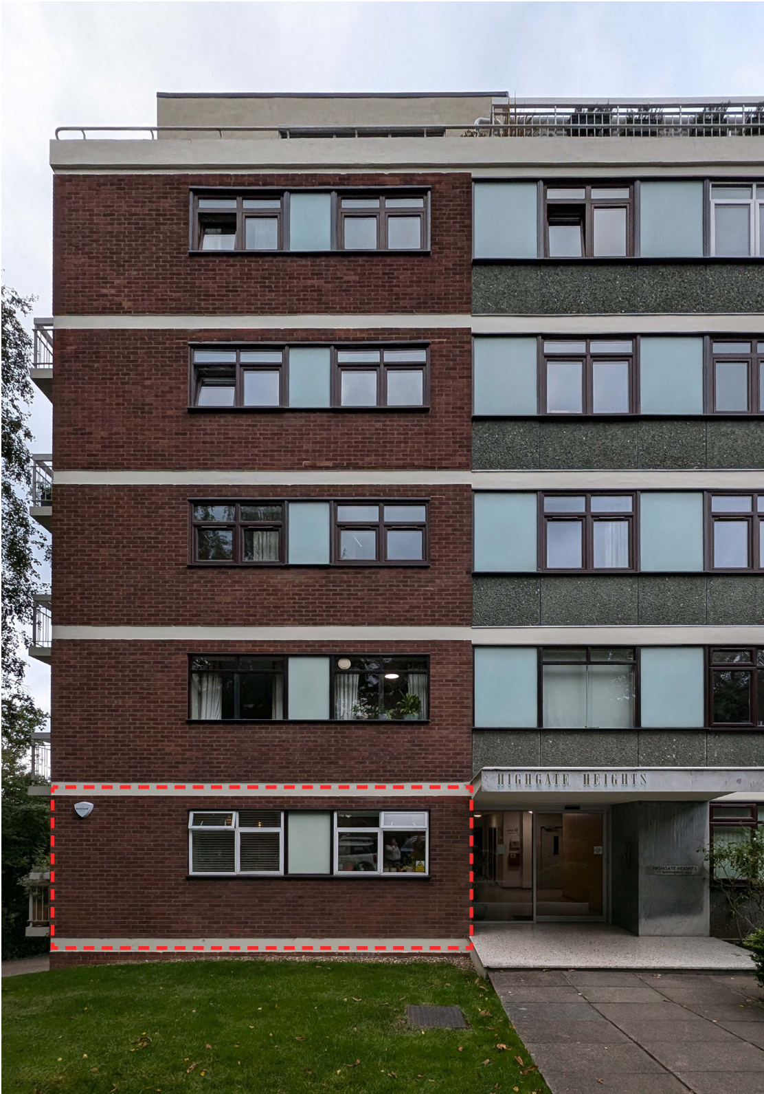
Front elevation showing inconsistency in the window frames within the same building
