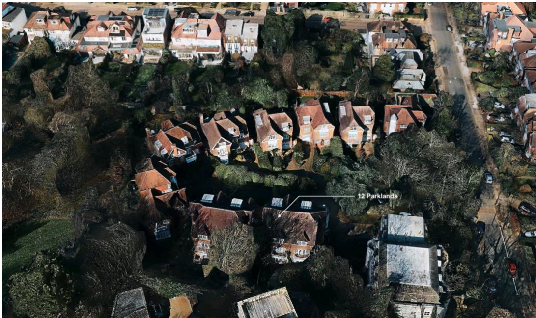
Application site looking north
