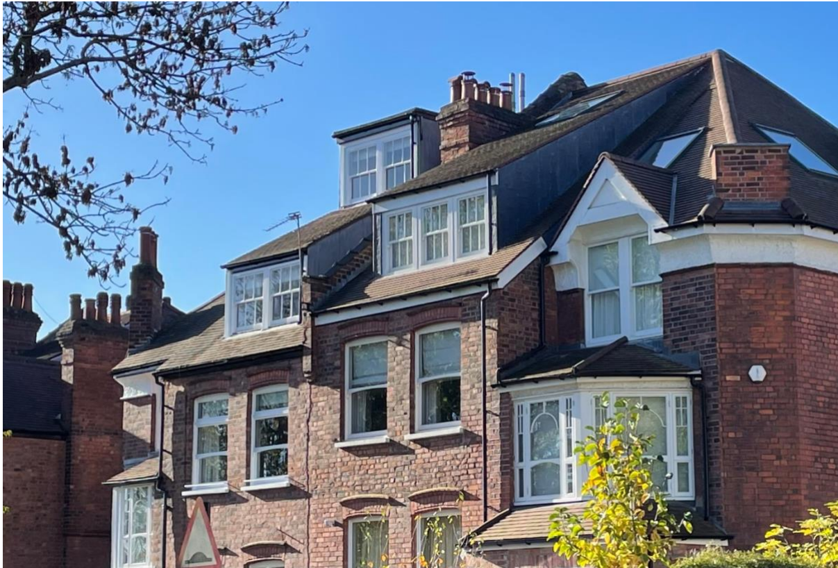
Rear roof dormers - Stanhope Road N6 within the HCA
