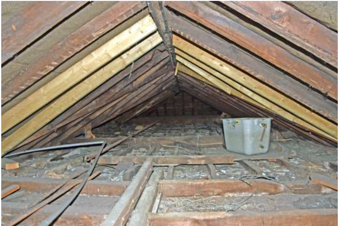
Figure 191: Overview photograph of loft for main residence, facing east. Taken 22.10.24.
