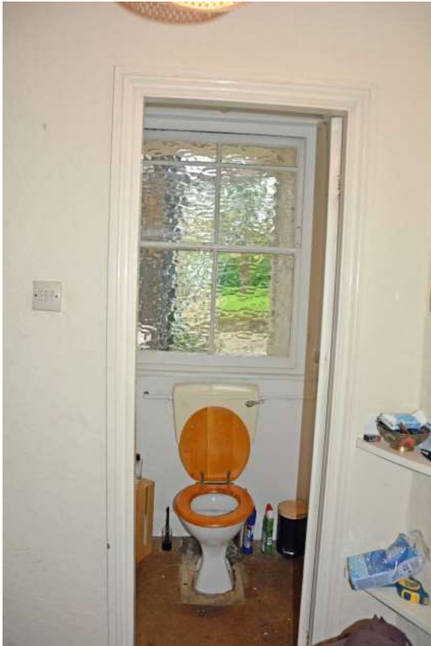
Figure 148a: Overview photograph of Area F. Taken 01.11.24
