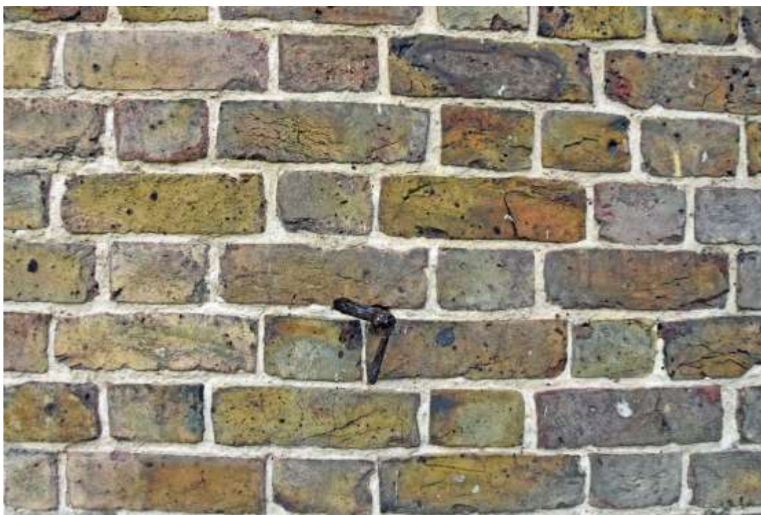
Figure 84: Detail Photograph of metal feature within the brickwork of the rear elevation. Taken 22.10.24.
