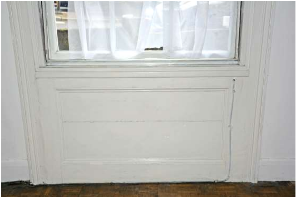
Figure 152: Detail Photograph of sash window shutter box on the eastern wall of Area G. Taken 01.11.24.
