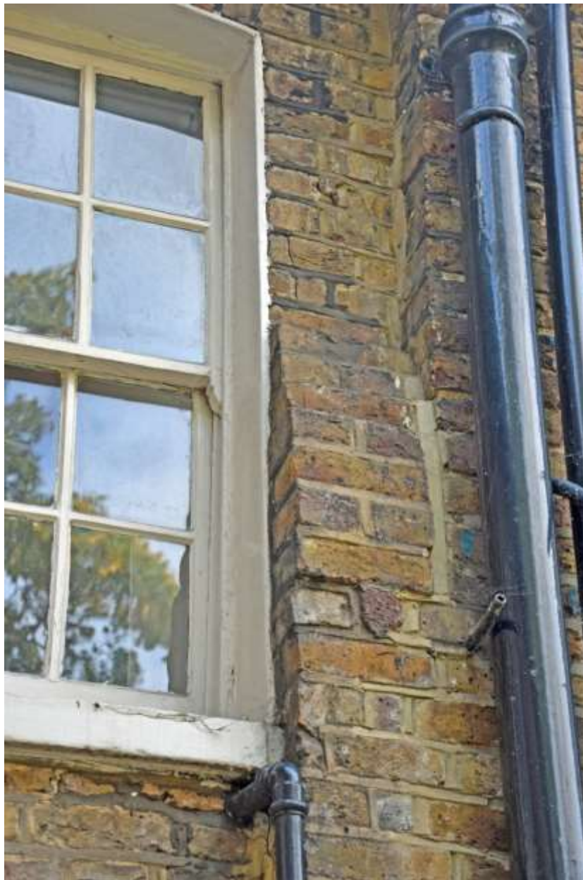
Figure 55: Detail photograph of stepped-out brickwork adjacent to the upper left window on the northern side elevation. Taken 22.10.24.
