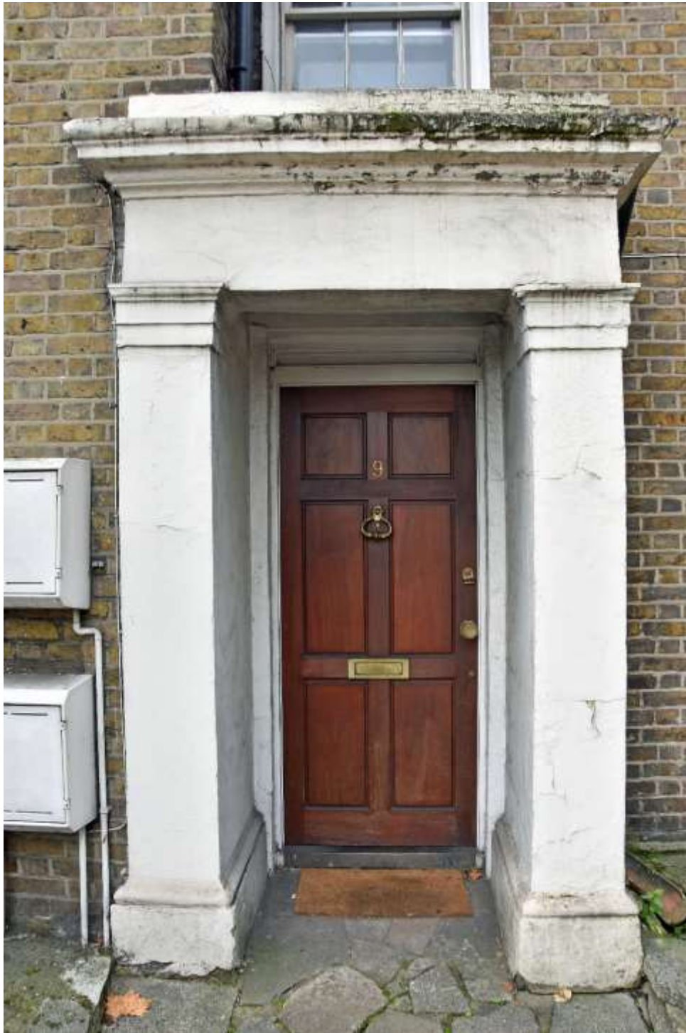
Figure 34: Photograph of the front door (principle entrance) and porch. Taken 22.10.24.
