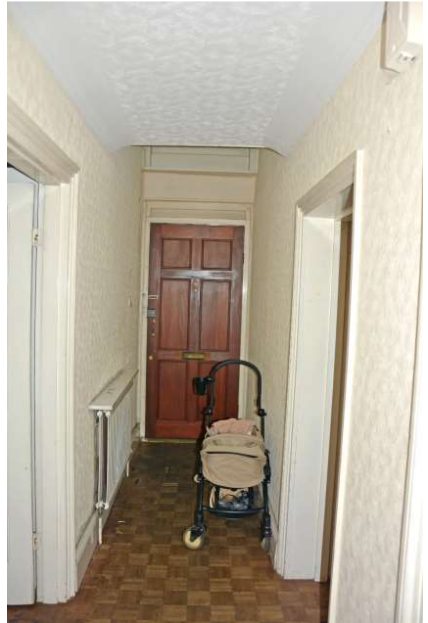
Figure 125: Overview of hallway (Area B) facing east. Taken 01.11.24.
