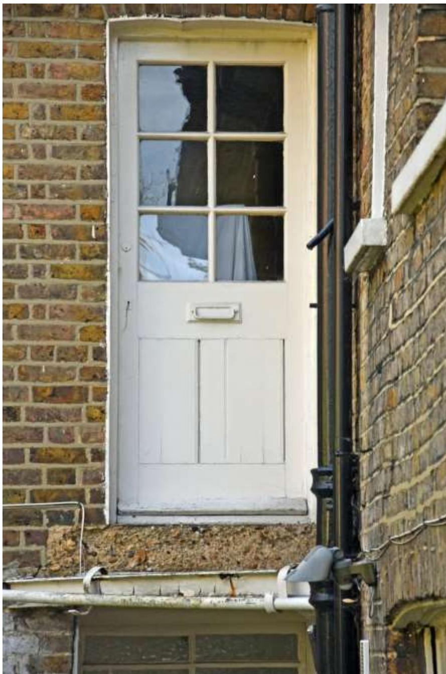
Figure 72: Photograph of first floor flat door on rear elevation. Taken 22.10.24.
