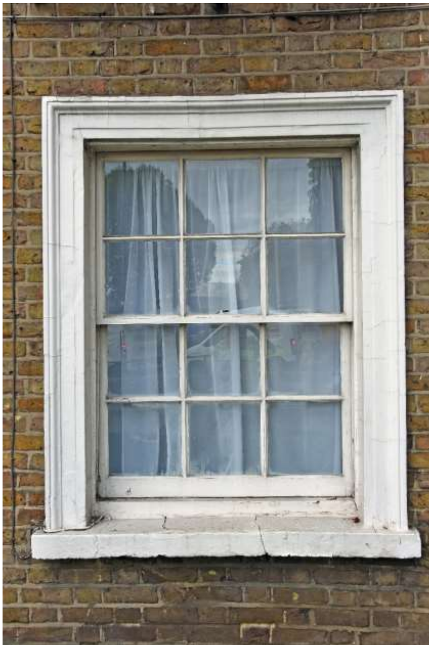
Figure 31: Photograph of the ground floor right window on the front façade. Taken 22.10.24.
