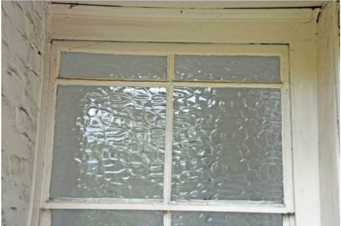
Figure 78: Detail Photograph of the lower central window of the rear elevation. Taken 22.10.24.
