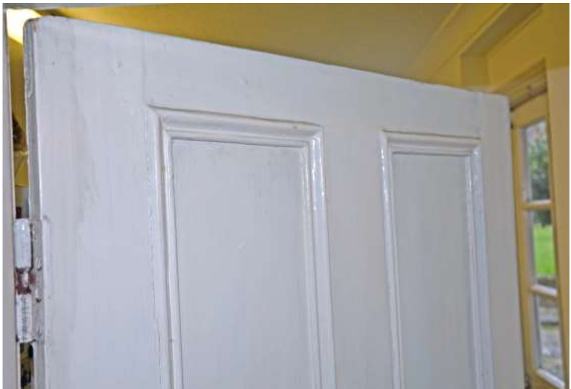
Figure 143: Detail photograph of door providing access to Area E. Taken 11.12.24.
