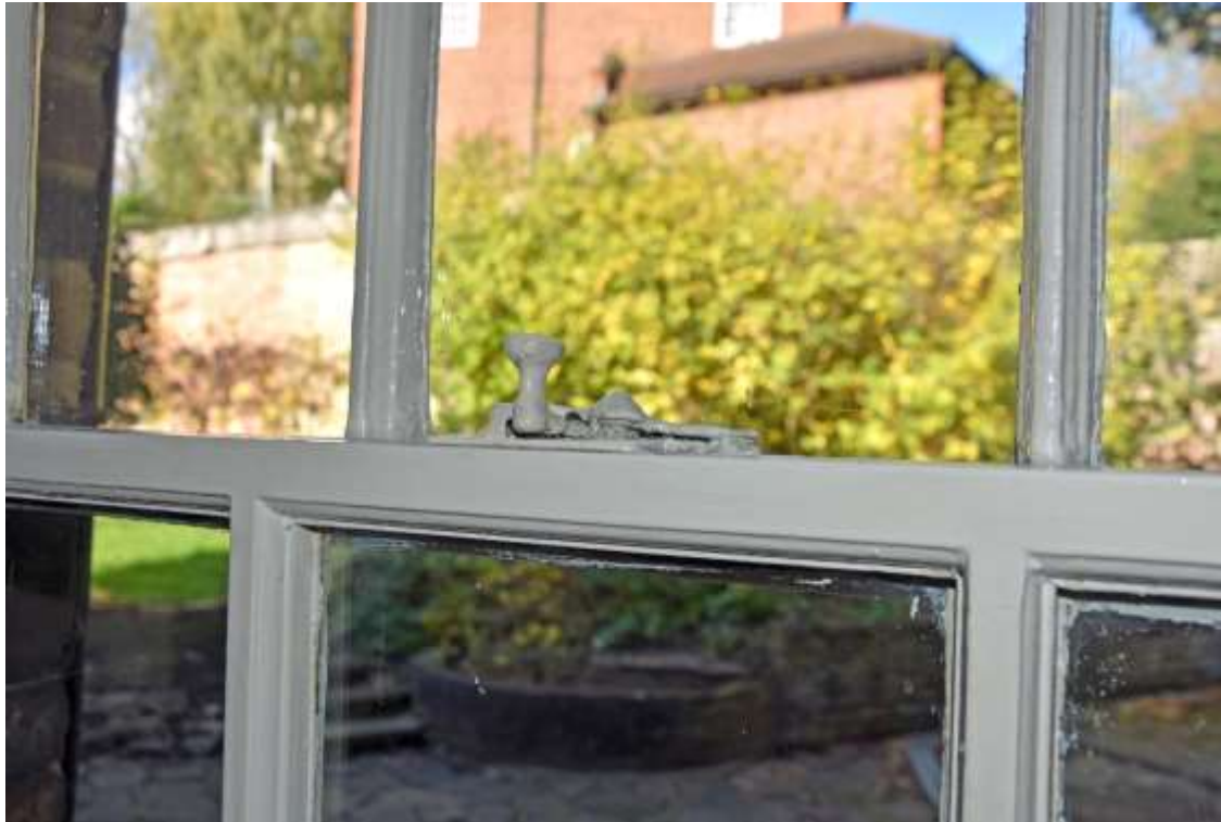
Figure 144: Detail photograph of window in Area E. Taken 22.10.24.
