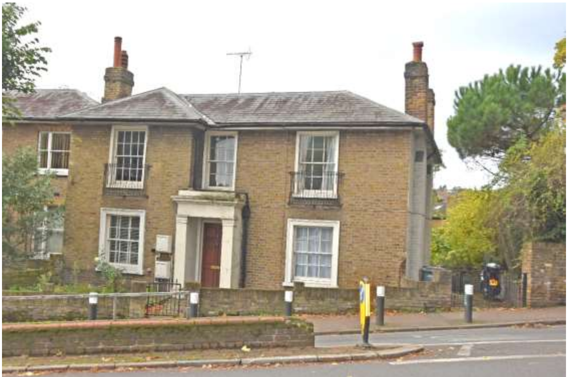
Figure 14: Photograph of Front Elevation of 9 Muswell Hill. Taken 22.10.24. Facing SW.
