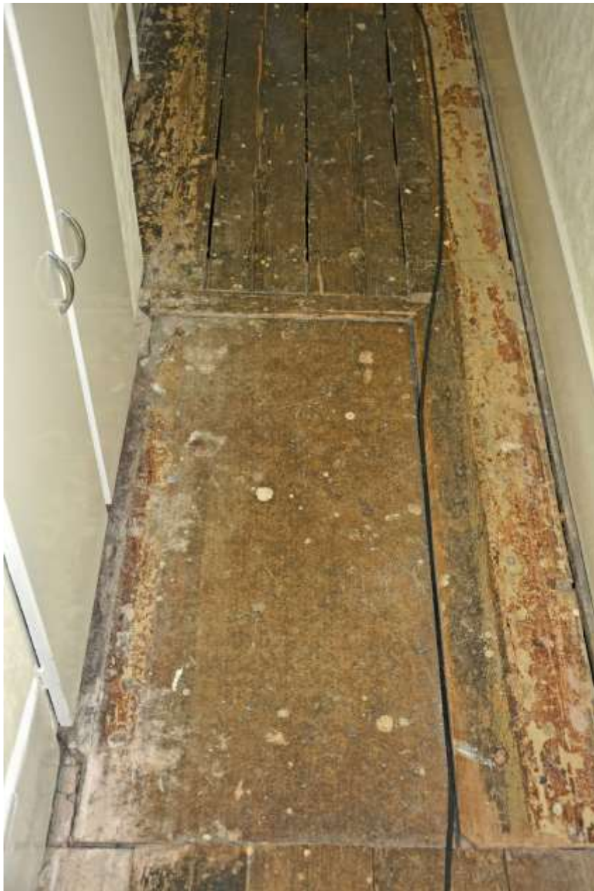
Figure 165: Detail Photograph of hallway flooring around former fireplace/hearth. Taken 01.11.24.
