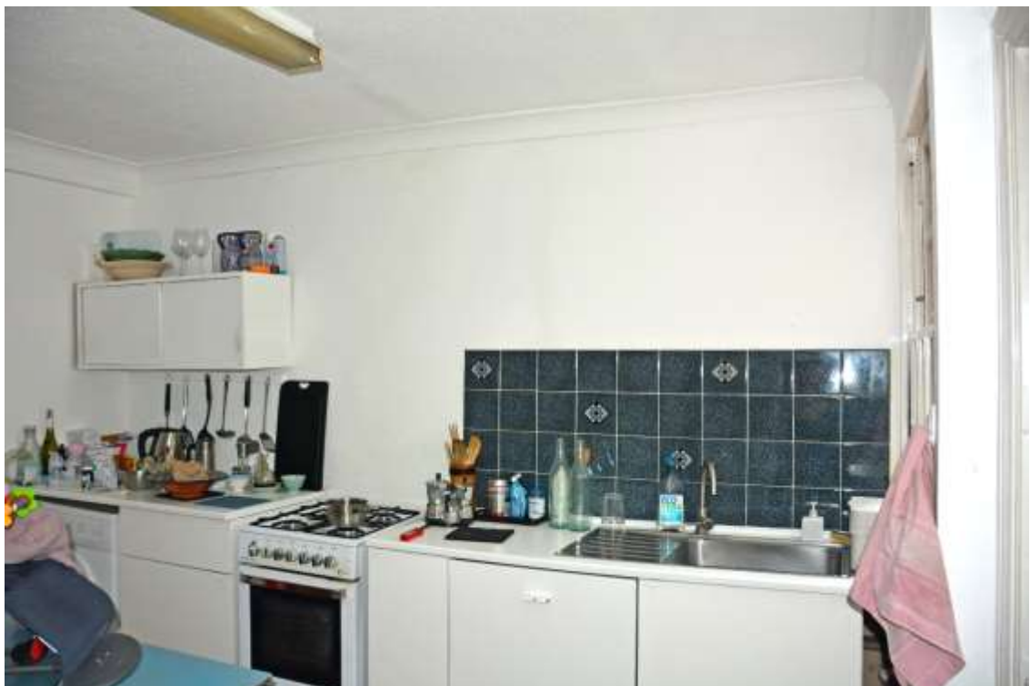
Figure 141: Overview photograph of Area E (kitchen), as viewed from doorway in Area D. Taken 01.11.24.
