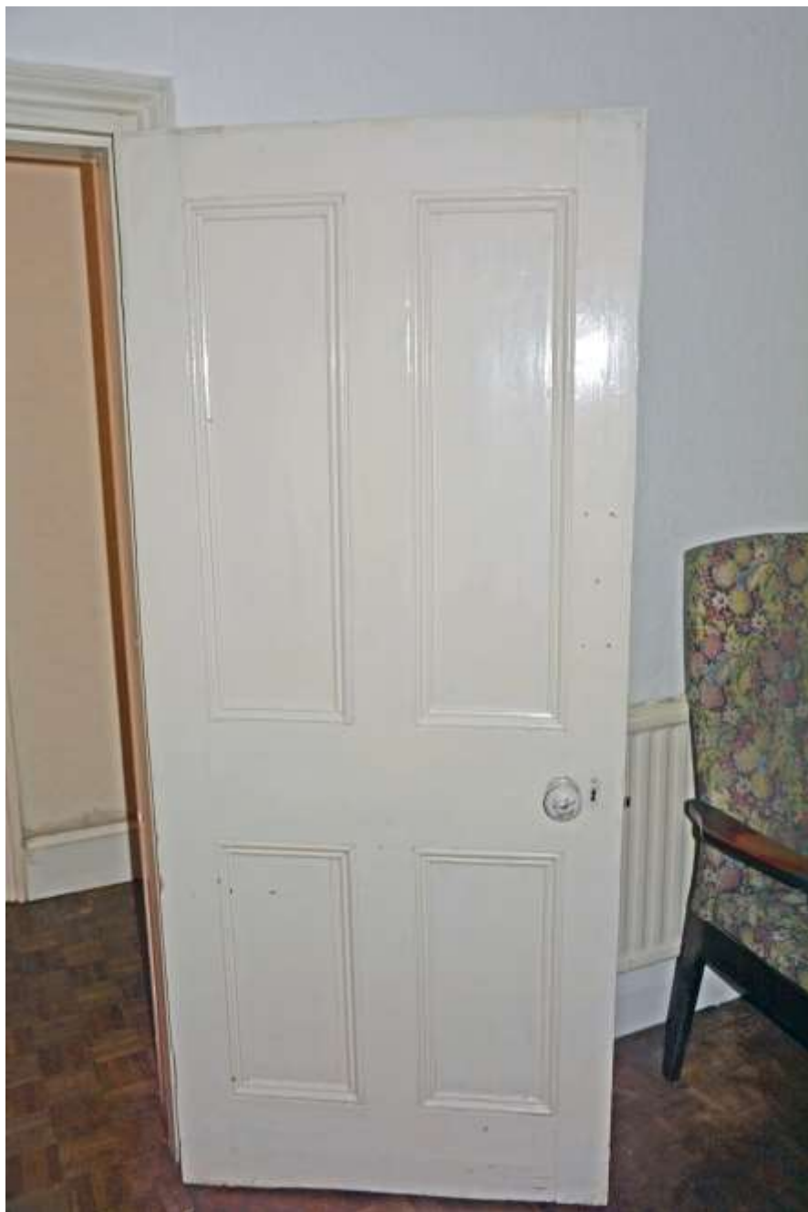
Figure 127: Door between Area B and Area C. Taken 01.11.24.
