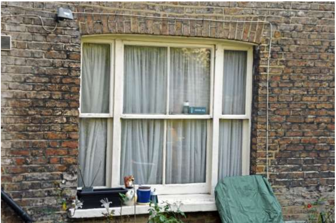
Figure 63: Photograph of lower central window on the northern side elevation. Taken 22.10.24.
