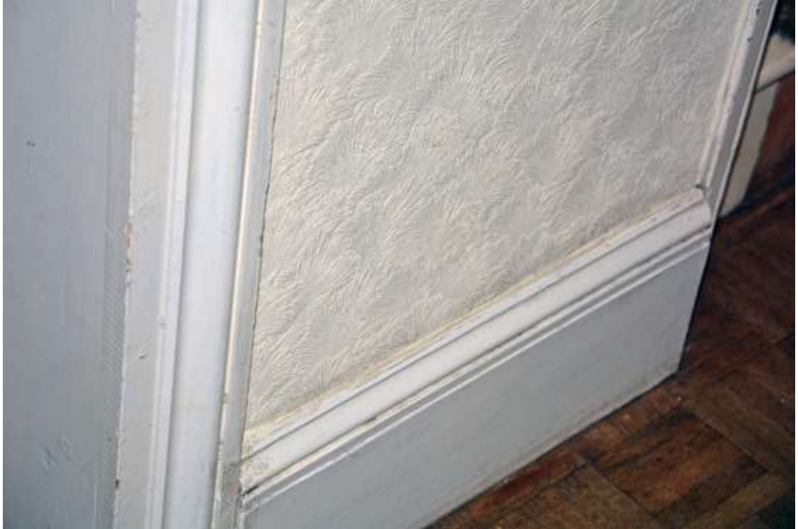
Figure 120: Detail Photograph of hallway skirting board on southern side. Taken 01.11.24.
