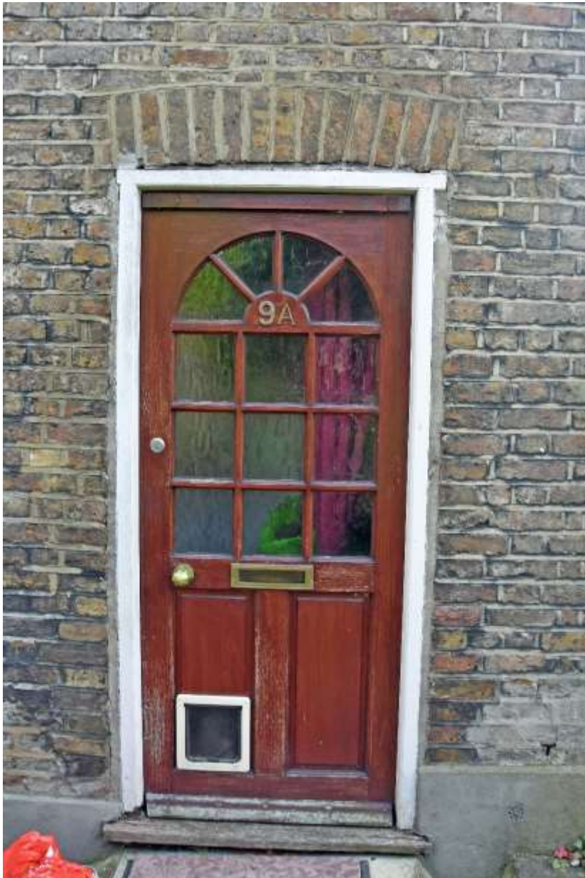
Figure 60: Overview Photograph of Front Door to rear property (9a Muswell Hill). Taken 22.10.24.
