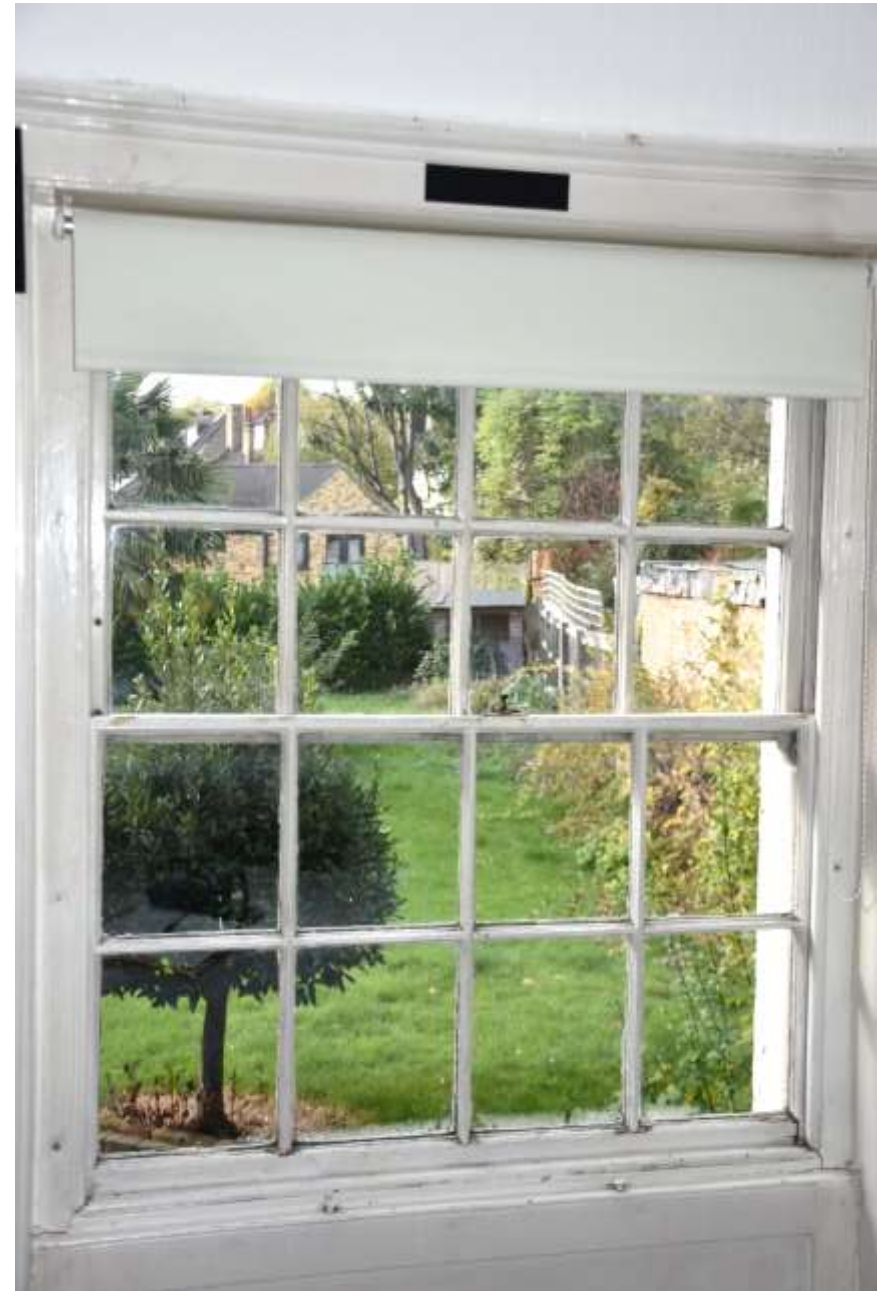
Figure 184: Detail of window within Area P. Taken 01.11.24.
