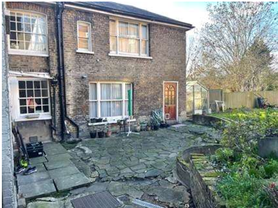
Figure 108: Overview of the rear patio area. January 2026.
