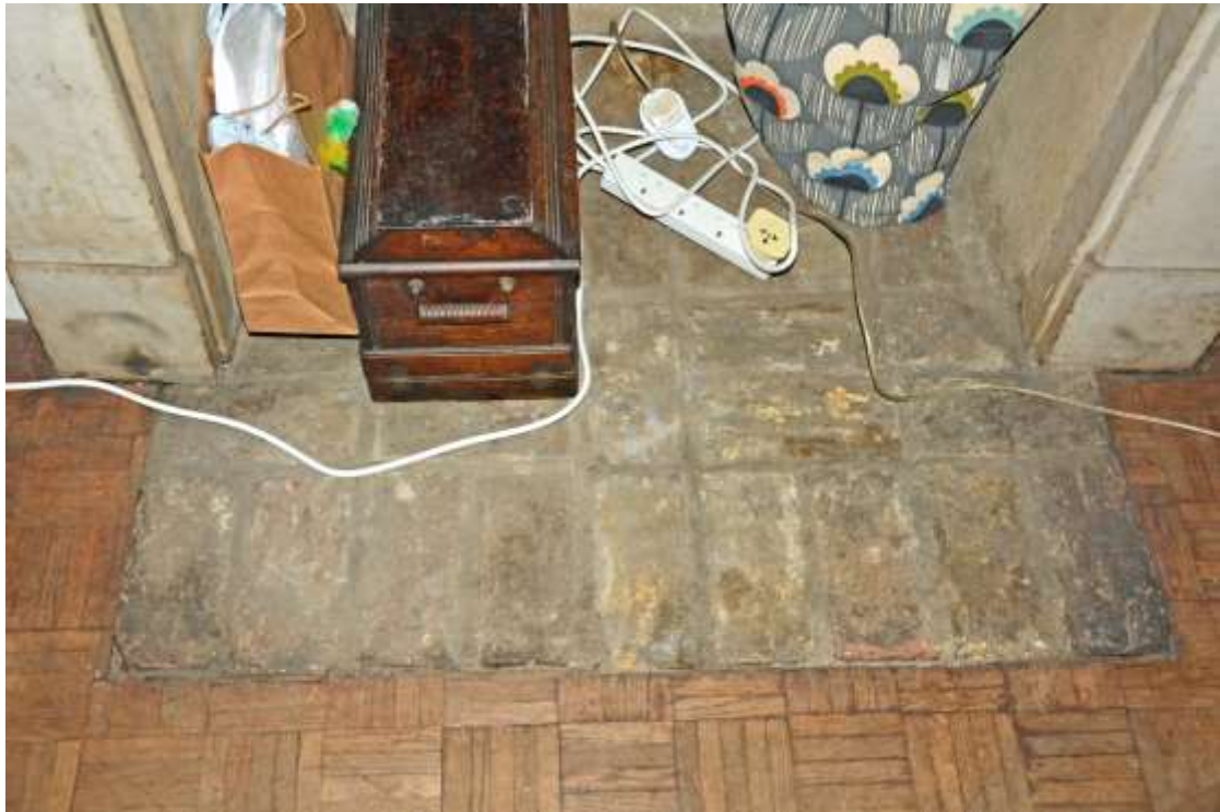
Figure 134: Detail Photograph of Fireplace base in Area C. Taken 01.11.24.
