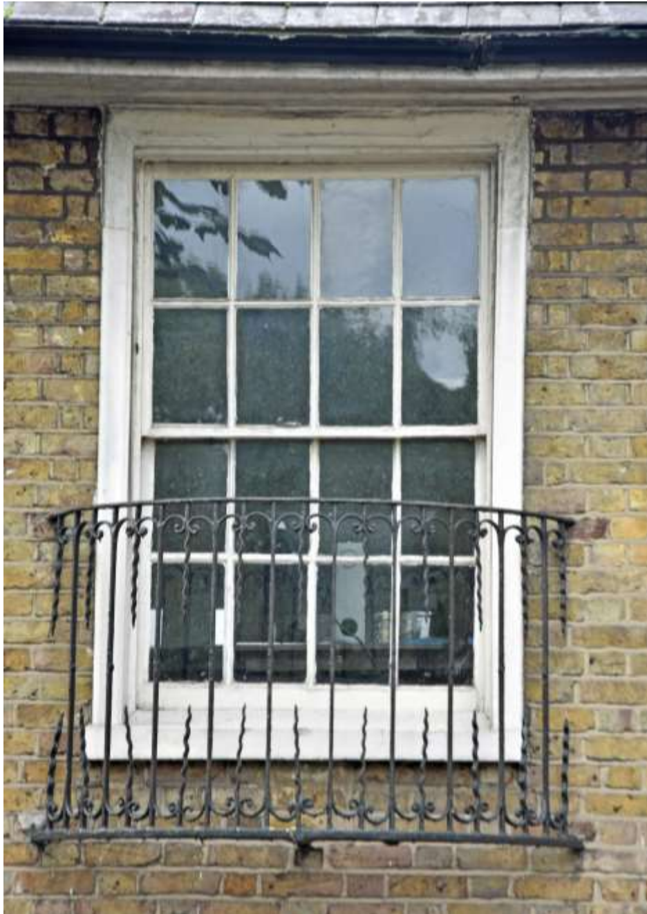
Figure 22: Photograph of the first floor left window on the front façade. Taken 22.10.24.
