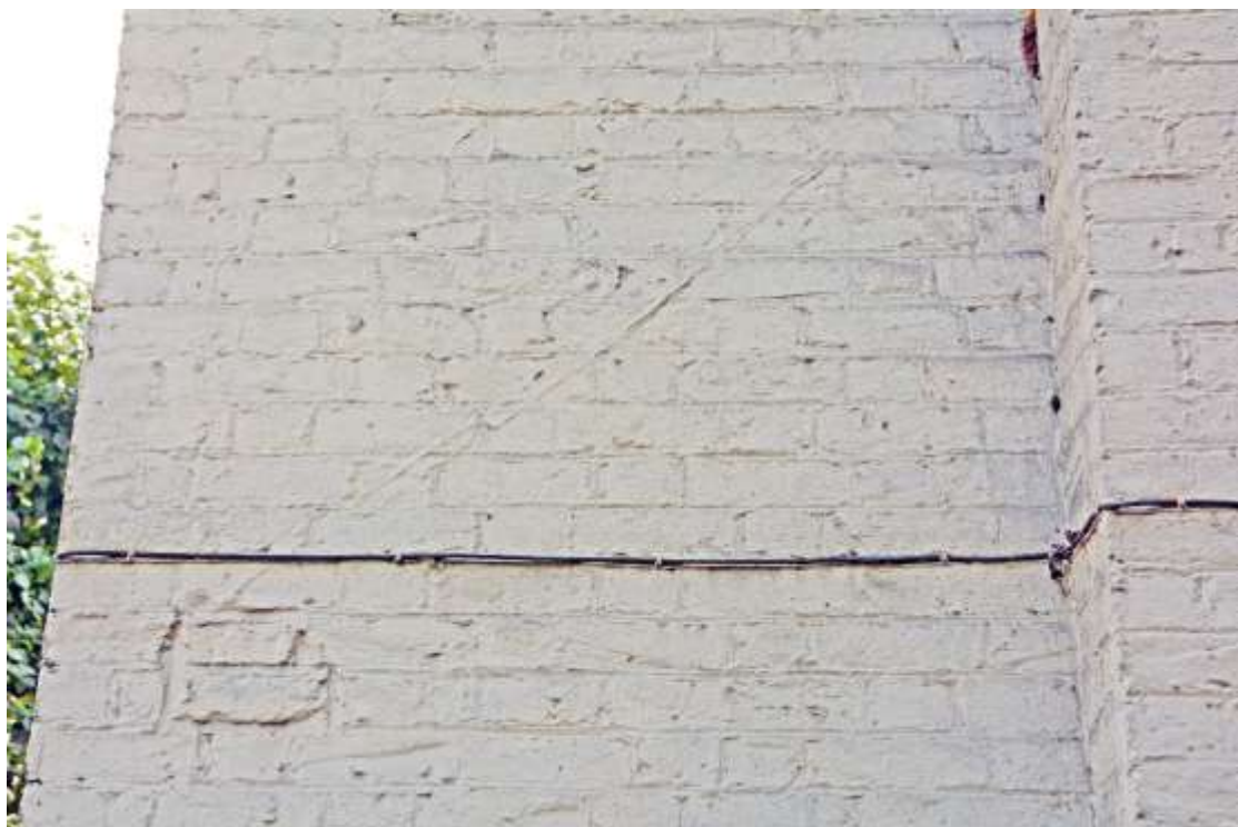
Figure 45: Detail of whitewashed wall, with diagonal slope of the formerly adjoining roof visible.
