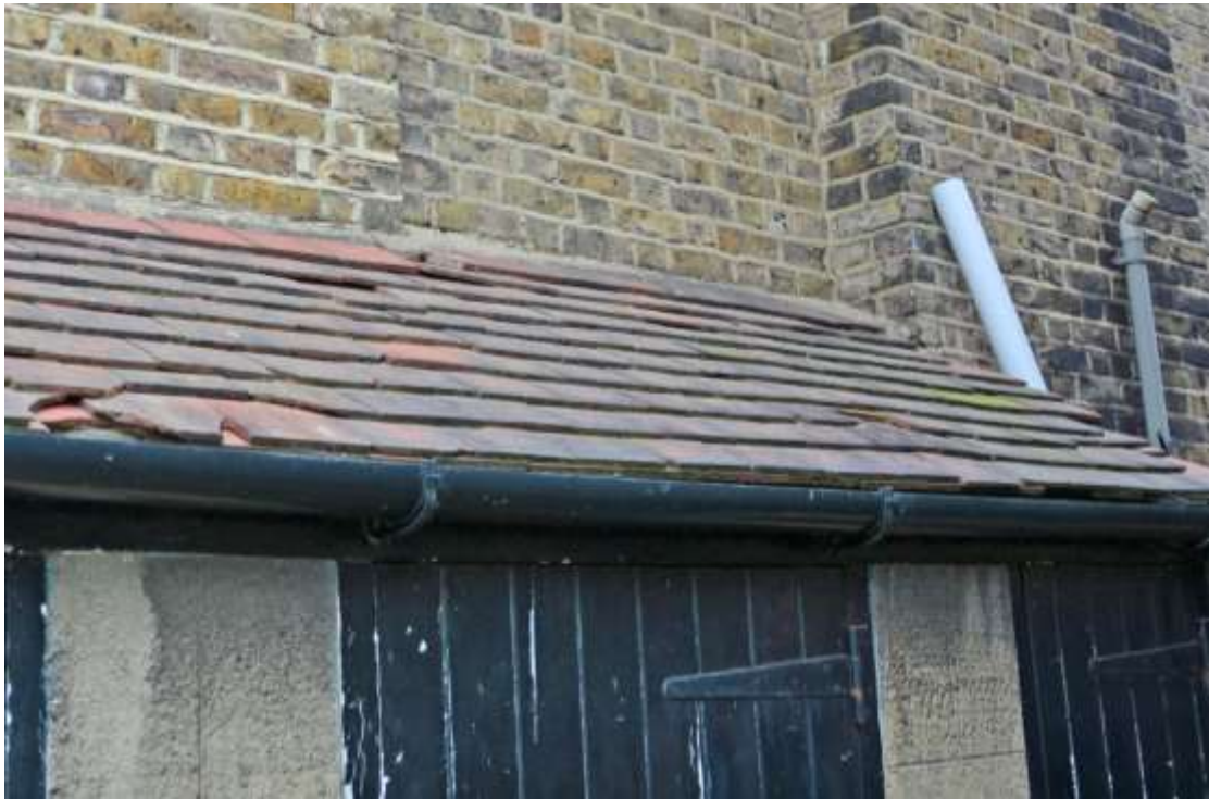
Figure 90: Detail photograph of 7 Muswell Hill shed feature and its attachment to the side wall of no. 9 Taken 01.11.24.
