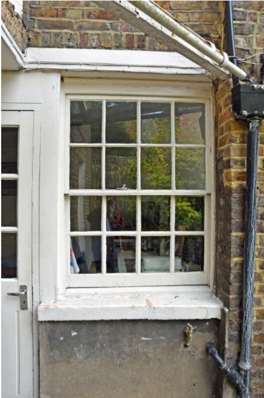
Figure 51: Photograph of ground floor far left window on the rear north side elevation. Taken 22.10.24.
