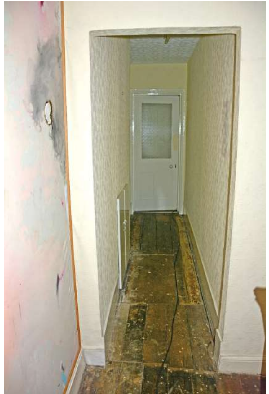
Figure 166: Overview Photograph of southern hallway section, original fireplace to the left. Taken 01.11.24.
