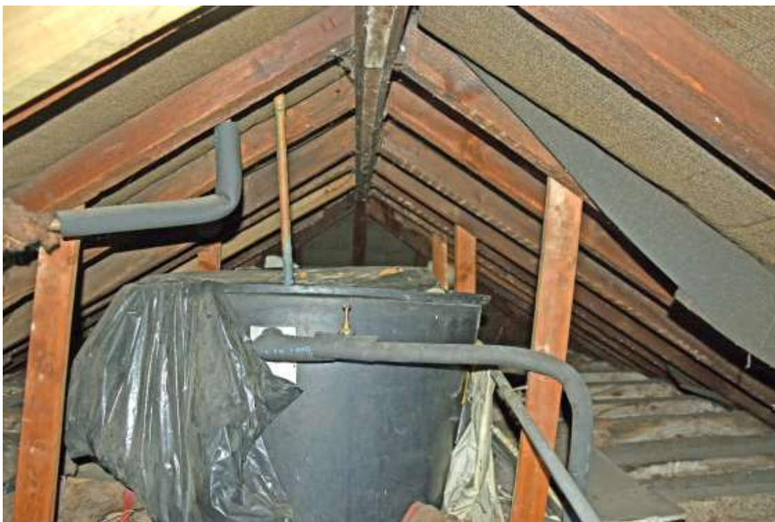
Figure 189: Overview of loft overlying 9a Muswell Hill, looking west. Taken 22.10.24.
