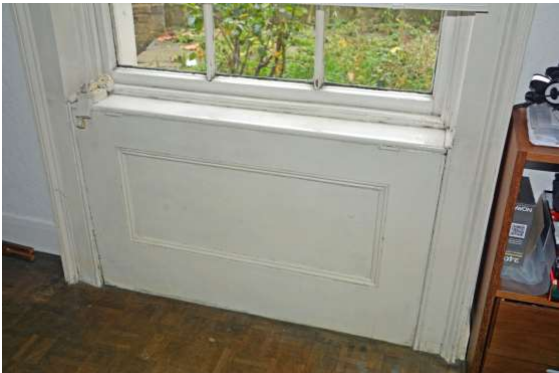
Figure 137: Shutter Box feature underlying window in Area C. Taken 01.11.24.
