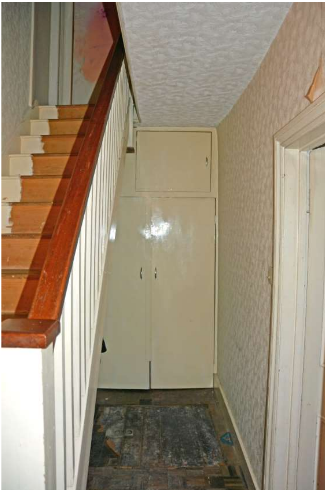
Figure 139: Overview of Area D – hallway and staircase. Taken 01.11.24.
