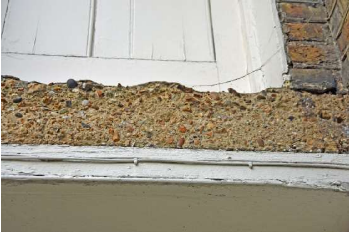
Figure 73: Detail Photograph of modern concrete slab for stair base – rear elevation. Taken 22.10.24.
