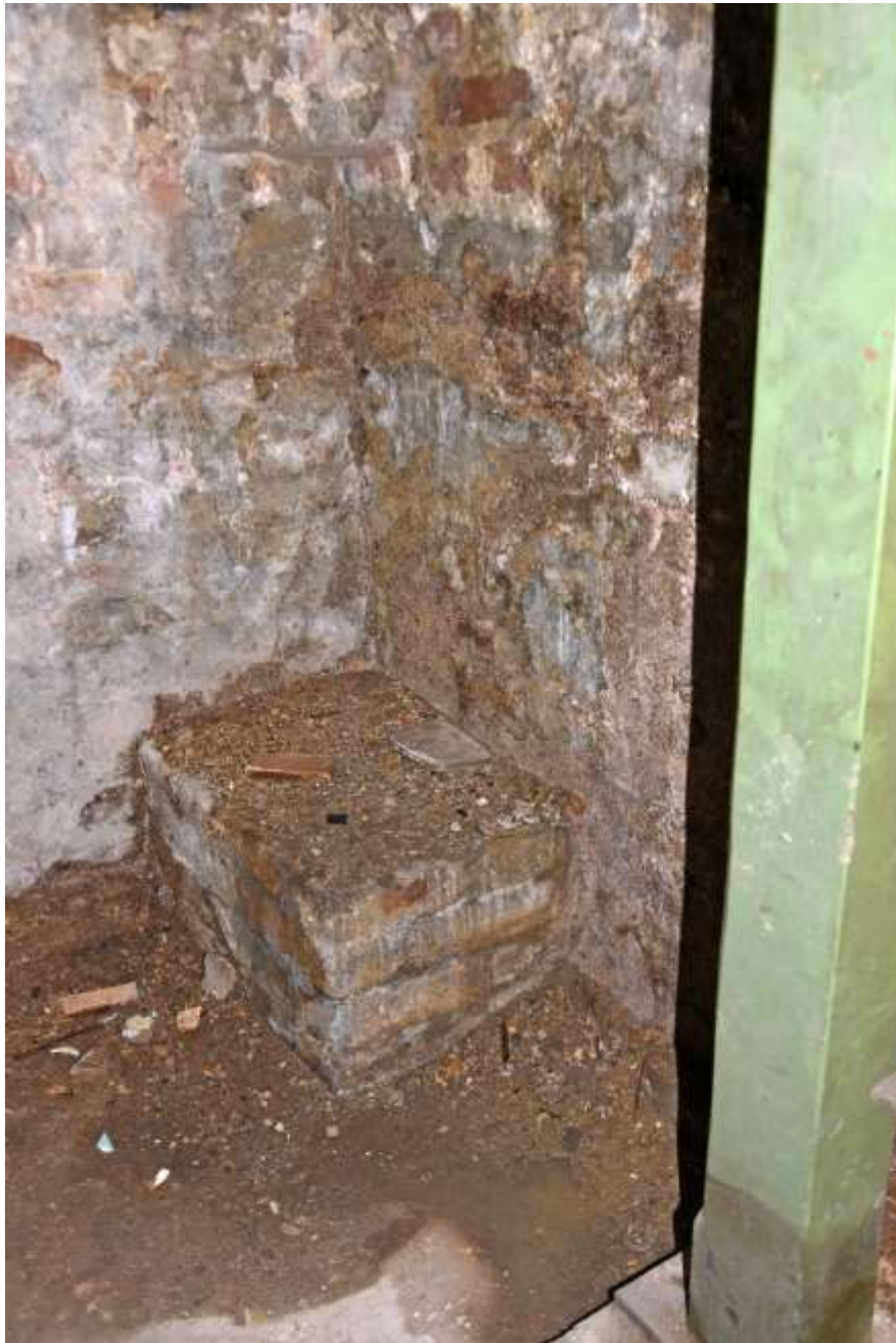
Figure 114: Stepped brick feature in northwest basement corner. Taken 22.10.24.
