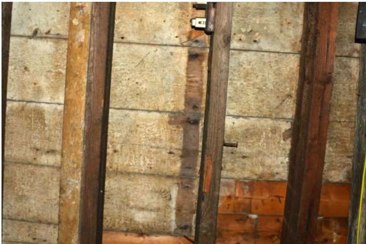
Figure 118: Detail, underside of floorboards as viewed from the basement & just in front of the lightwell. Newer, thin boards visible in the lower right (NE) corner. The older/wider boards have been painted, as have some of the original supporting joists. Taken 11.12.24.
