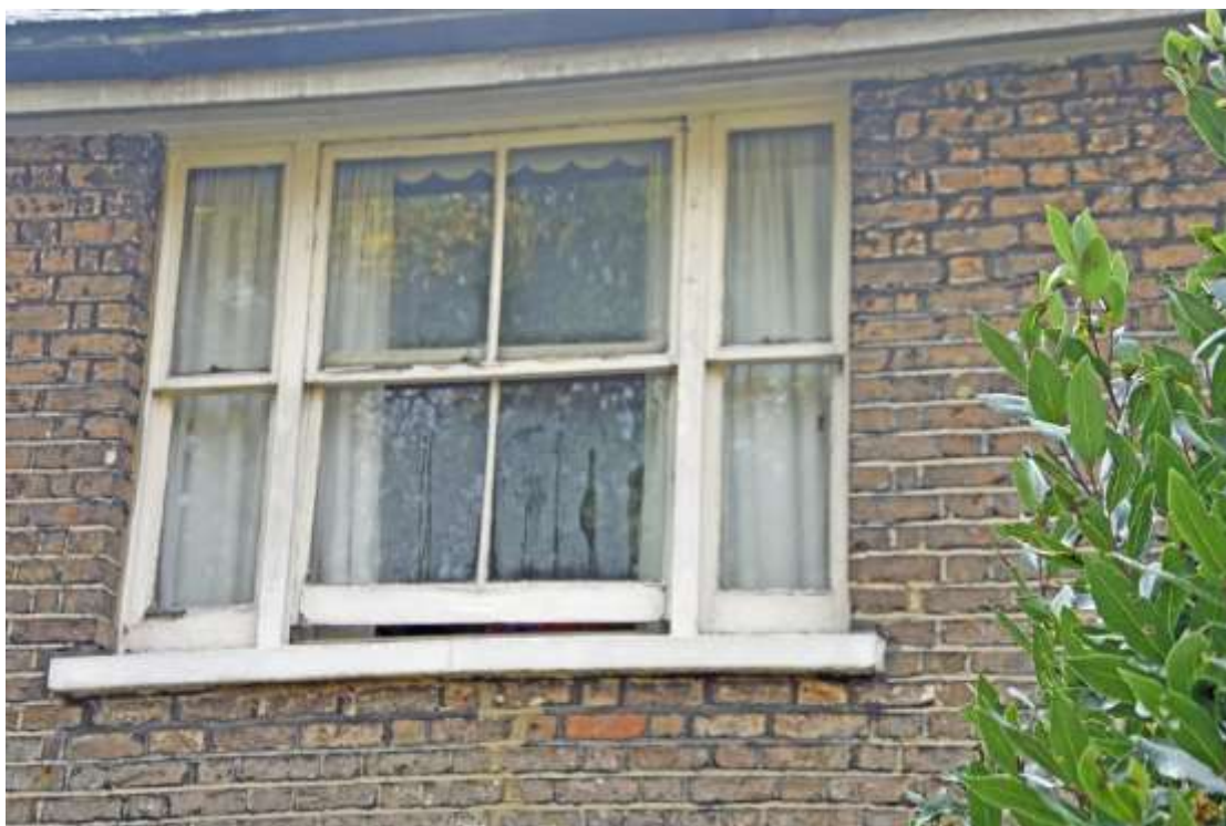
Figure 59: Photograph of the upper right window on the northern side elevation. Taken 22.10.24.
