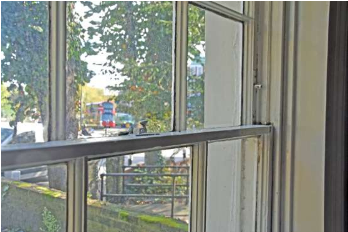
Figure 136: Detailing of window interior within Area C. Taken 22.10.24.
