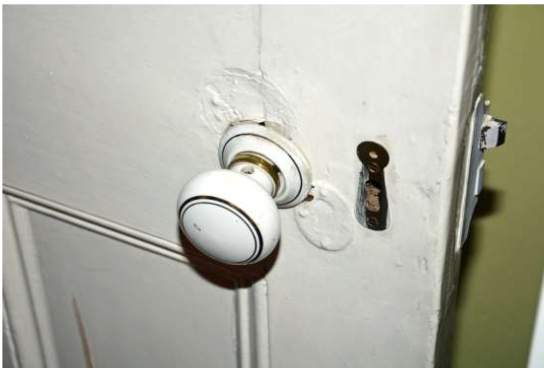
Figure 188: Detail of Area Q door, with old hardware positioning visible. Taken 11.12.24.
