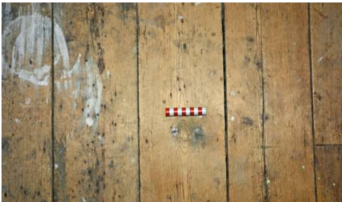
Figure 177: Detail Photograph of wide floor boards in Area O. 10cm scale Taken 11.12.24.
