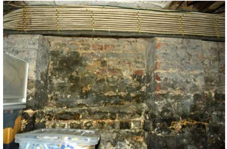
Figure 115: Brickwork quality, southern basement wall. Taken 22.10.24.
