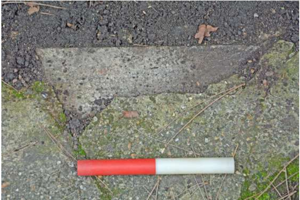
Figure 46: Detail of original floor from the coal shed or wood store feature, overlain by modern concrete (0.2m scale).
