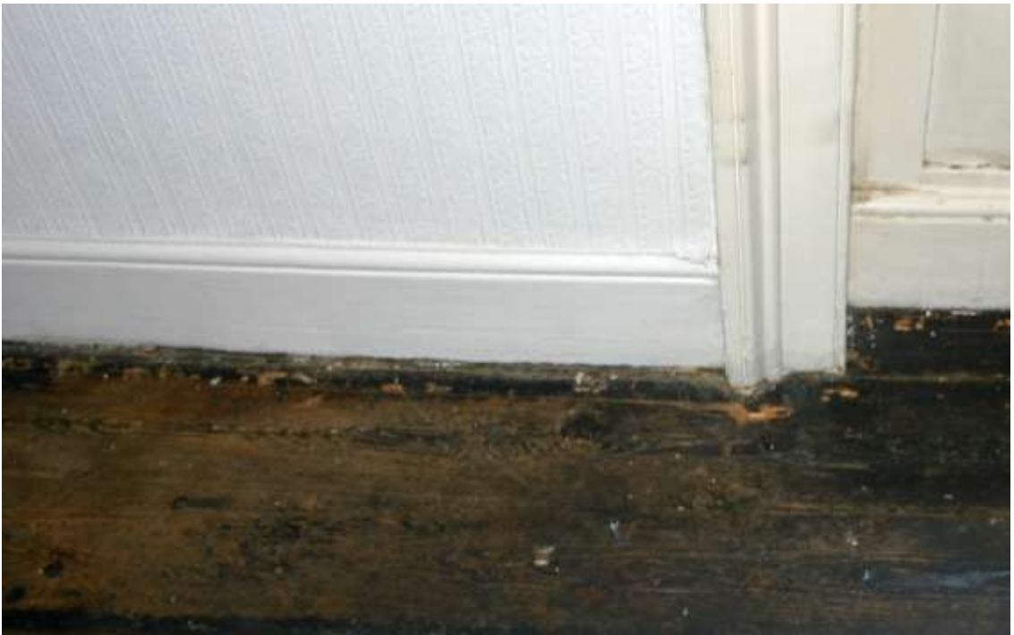
Figure 182: Detail Photograph of skirting boards in Area P. Taken 11.12.24.
