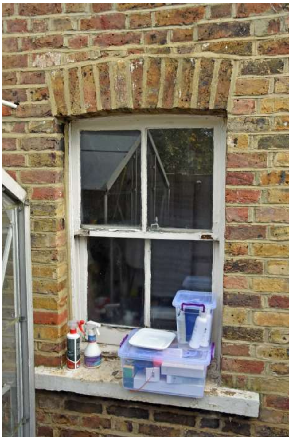
Figure 81: Photograph of the lower right window (9a) of the rear elevation. Taken 22.10.24.
