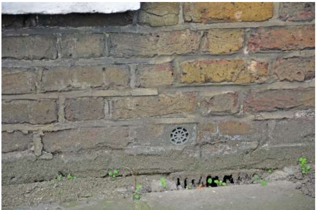
Figure 38: Detail of airbricks on the front of the residence, example taken from below lower right window.
