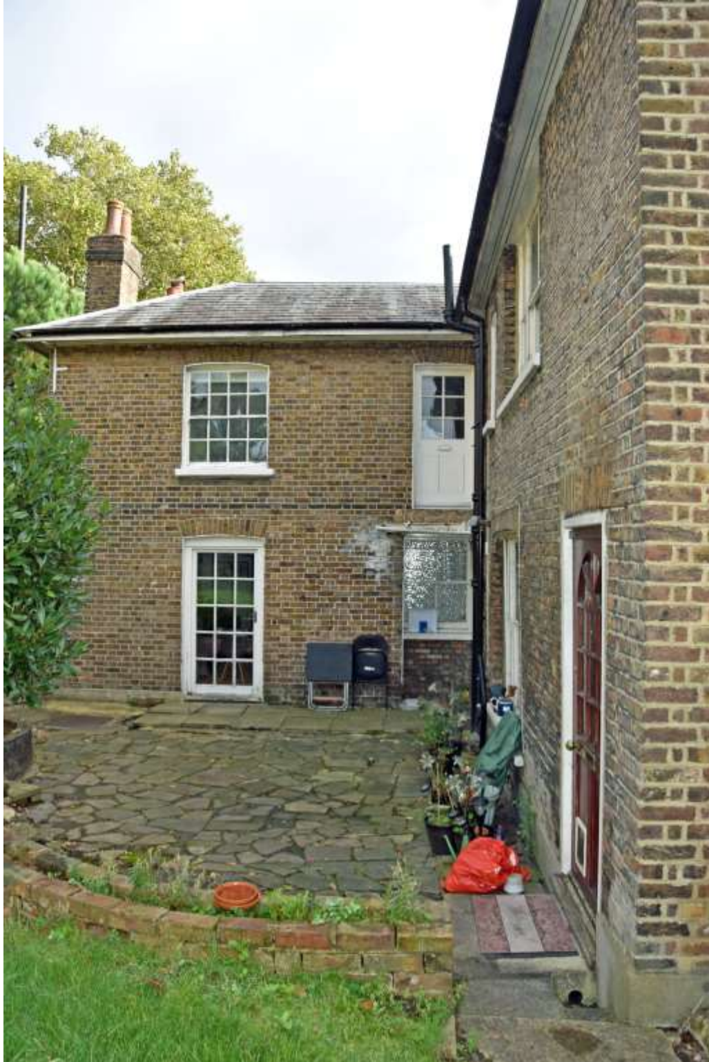
Figure 66: Overview Photograph of Rear Elevation (northern side). Taken 22.10.24.
