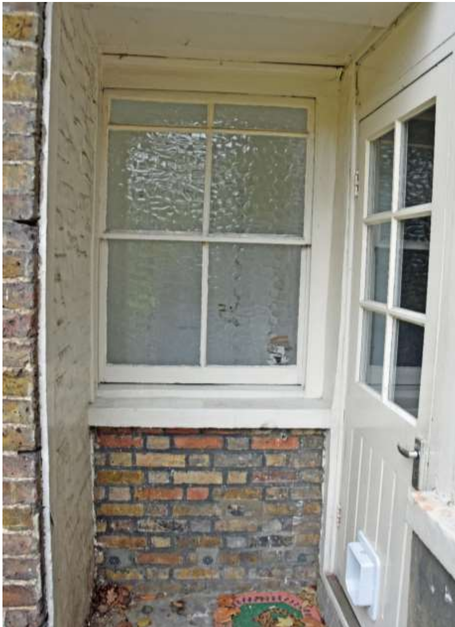
Figure 77: Overview Photograph of lower central window of rear elevation. Taken 22.10.24.
