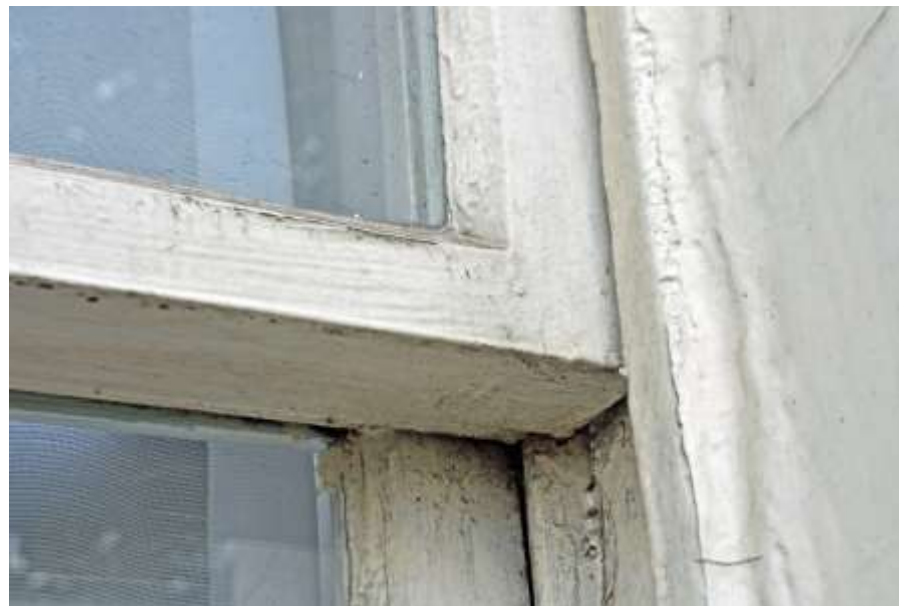
Figure 32: Detail of lower right window; areas of thickened paint visible.
