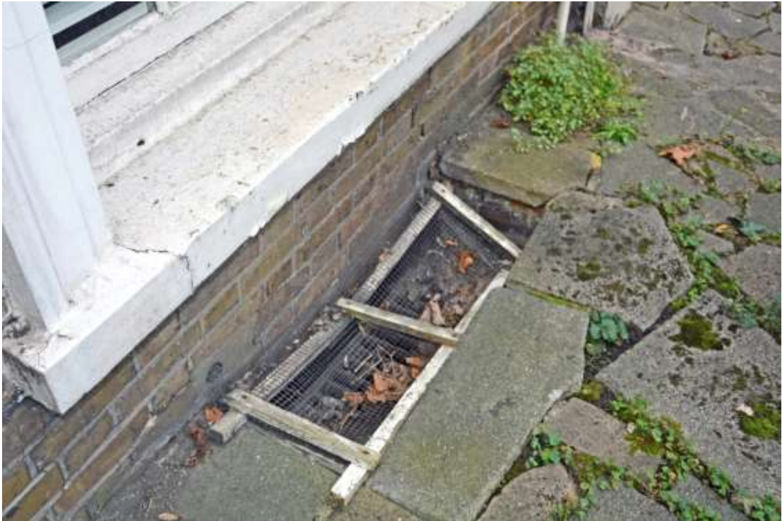
Figure 100: Photograph of lightwell feature within the front garden. Taken 01.11.24.
