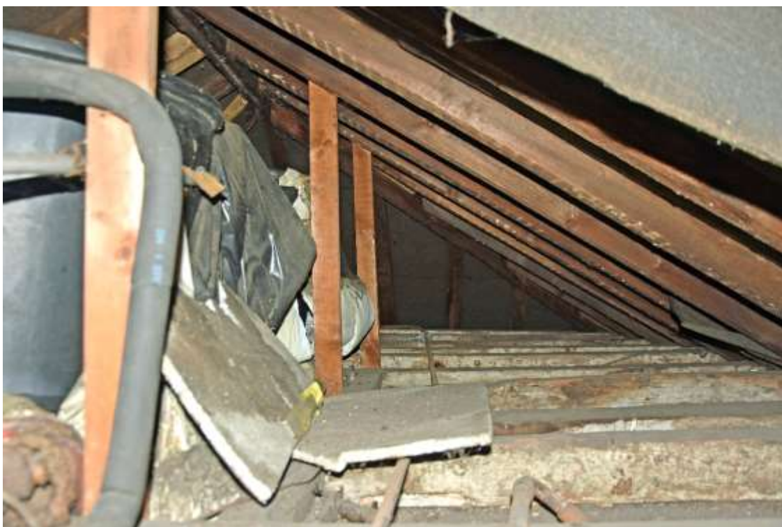
Figure 190: Detail of loft overlying 9a Muswell Hill, looking west. Taken 22.10.24.
