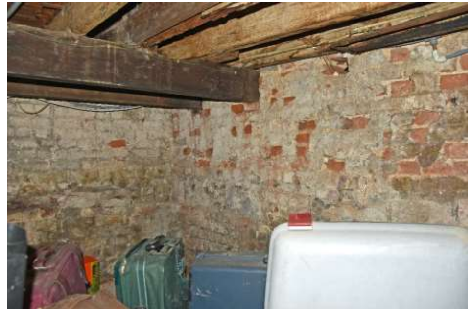
Figure 116: Overview of northwest basement corner. Taken 22.10.24.
