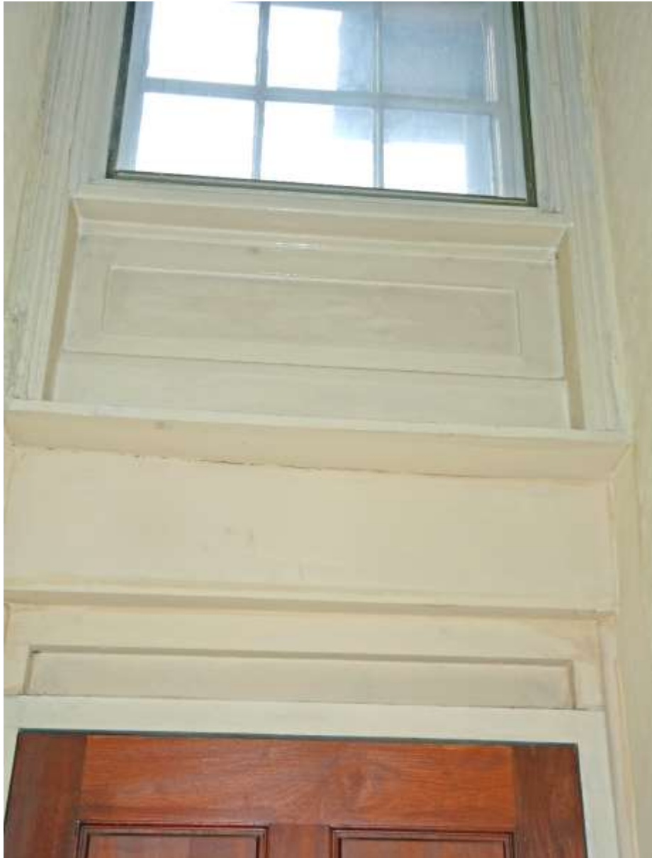
Figure 156: Photograph of panelling within the double height void in the eastern section of Area K.
