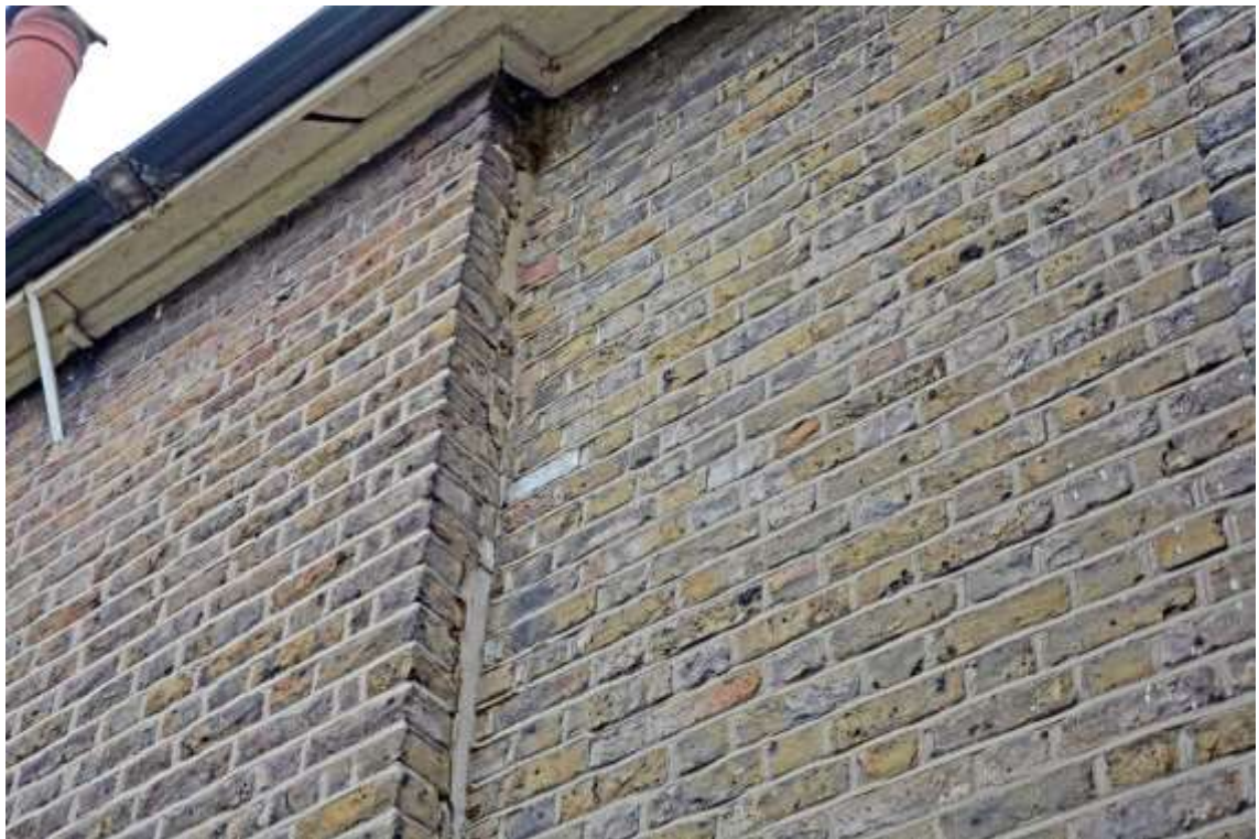
Figure 91: Detail Photograph of boundary between 9a and 9 Muswell Hill on the southern side elevation. Taken 01.11.24.
