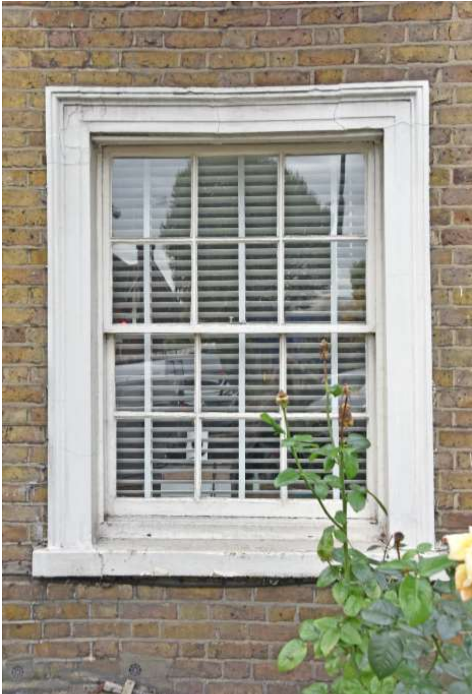
Figure 17: Photograph of the ground floor left window on the front façade. Taken 22.10.24.
