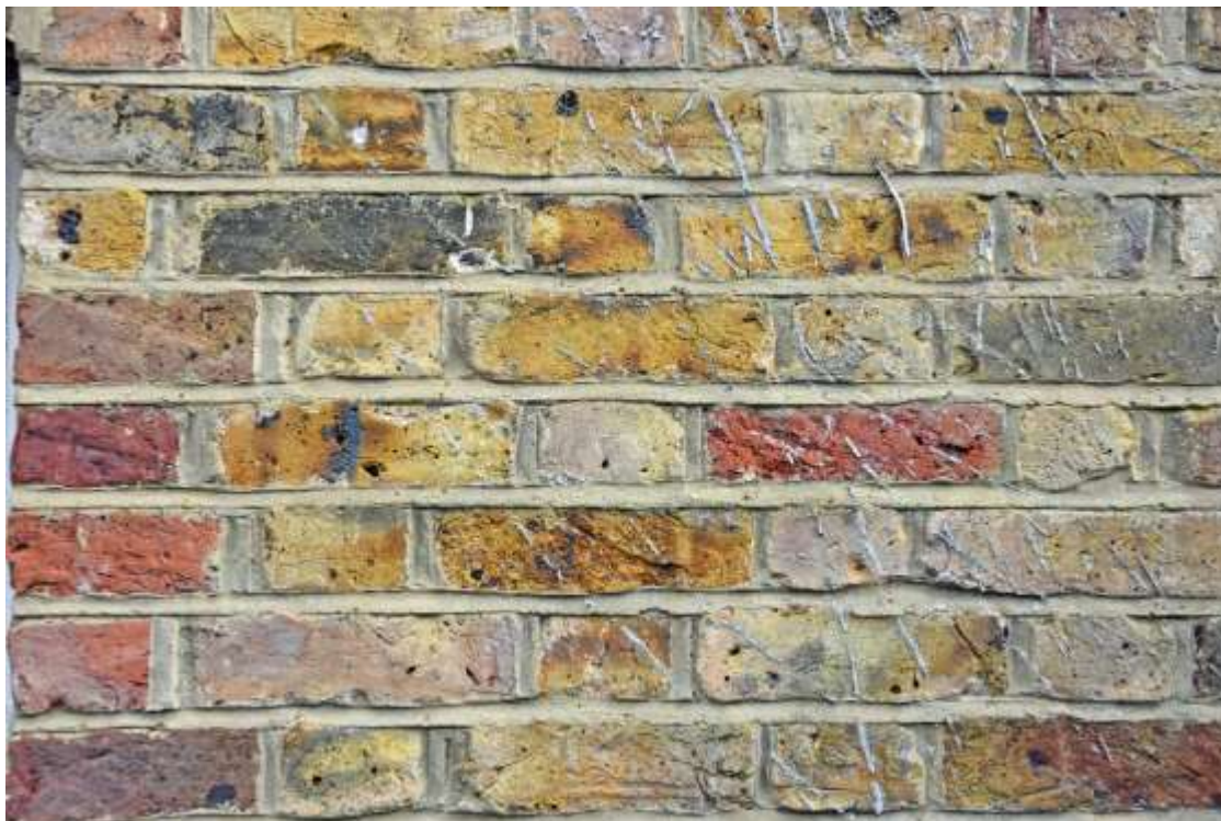
Figure 82: Detail Photograph of the brickwork to the right corner of the rear elevation, attachments from previously existing ivy observable. Taken 22.10.24.
