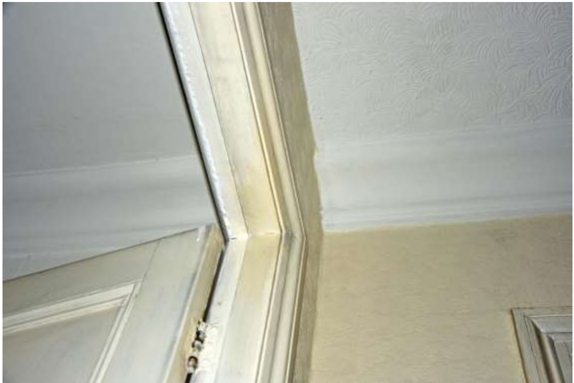
Figure 146: Detail photograph showing the continuation of the coving on the northern wall from Area B (right) into Area F (left). Taken 22.10.24.
