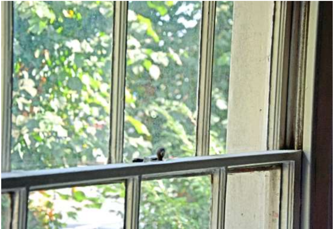
Figure 164: Detail photograph of window in Area L. Taken 22.10.24.
