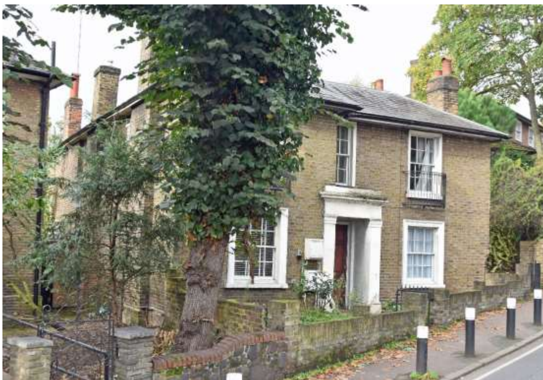
Figure 96: Overview Photograph of 9 Muswell Hill, with partial view of the front and side (south) elevations. Taken 22.10.24.
