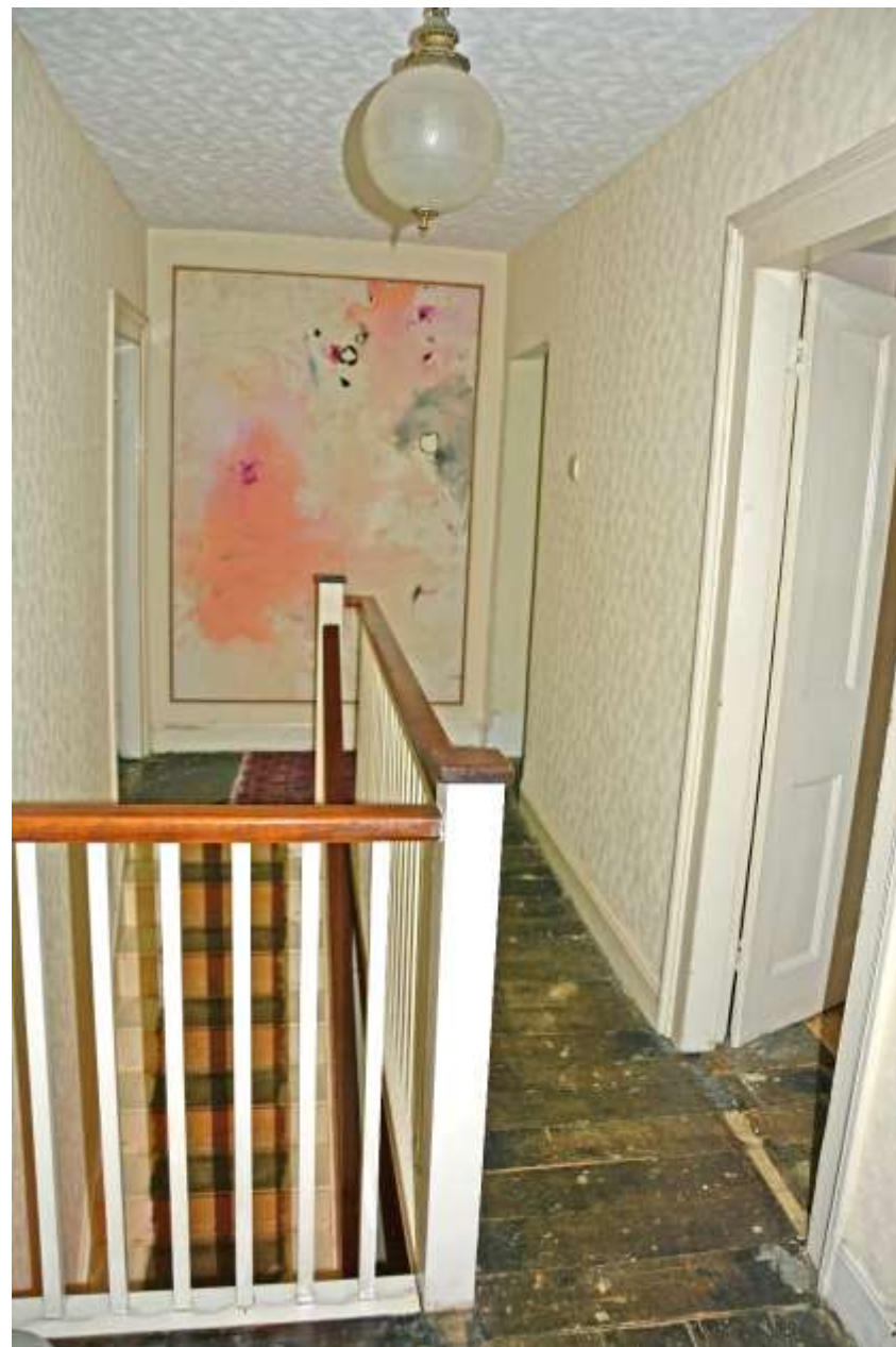
Figure 168: Overview of middle section of hallway. Taken 01.11.24.
