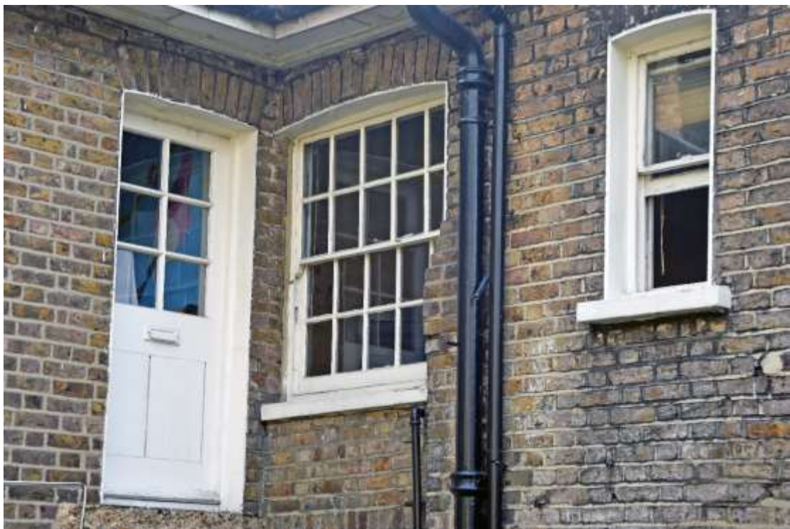
Figure 54: Overview Photograph of upper left window (centre) on the northern side elevation. Taken 22.10.24.
