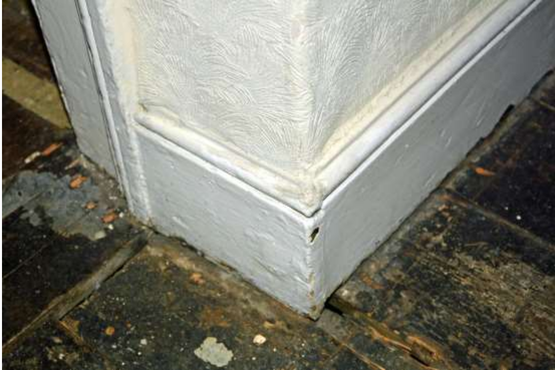
Figure 171: Detail Photograph of skirting boards in Area M. Taken 11.12.24.
