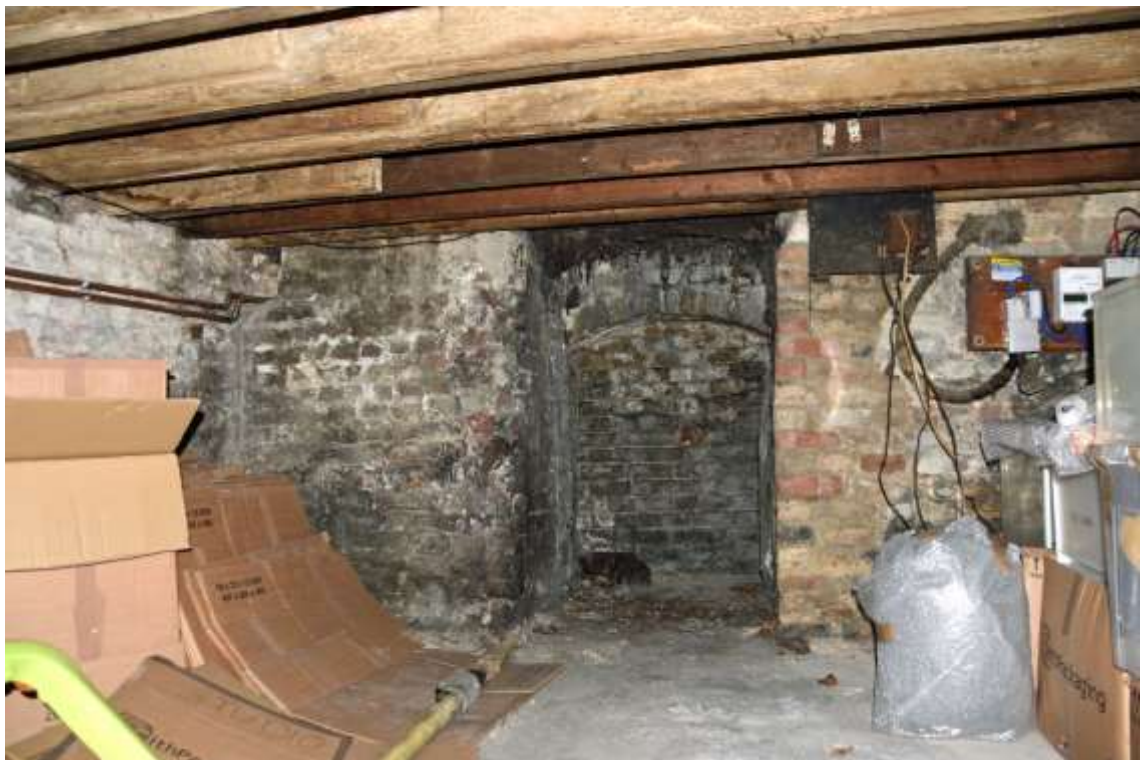
Figure 113: Overview Photograph of Basement, Lightwell feature visible to centre. Taken 22.10.24.
