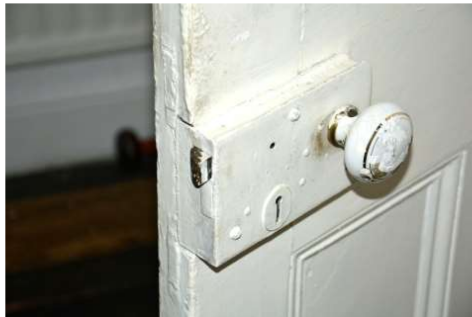
82 Figure 129: Detail of Door hardware in Area C. Taken 11.12.24.
