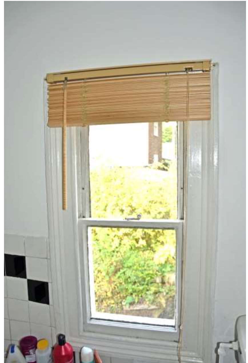
Figure 173: Detail Photograph of window in Area N. Taken 01.11.24.
