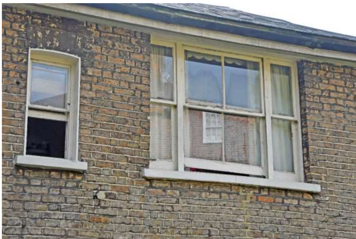
Figure 57: Overview of Upper Central Window (left) on the northern side elevation. Taken 22.10.24.
