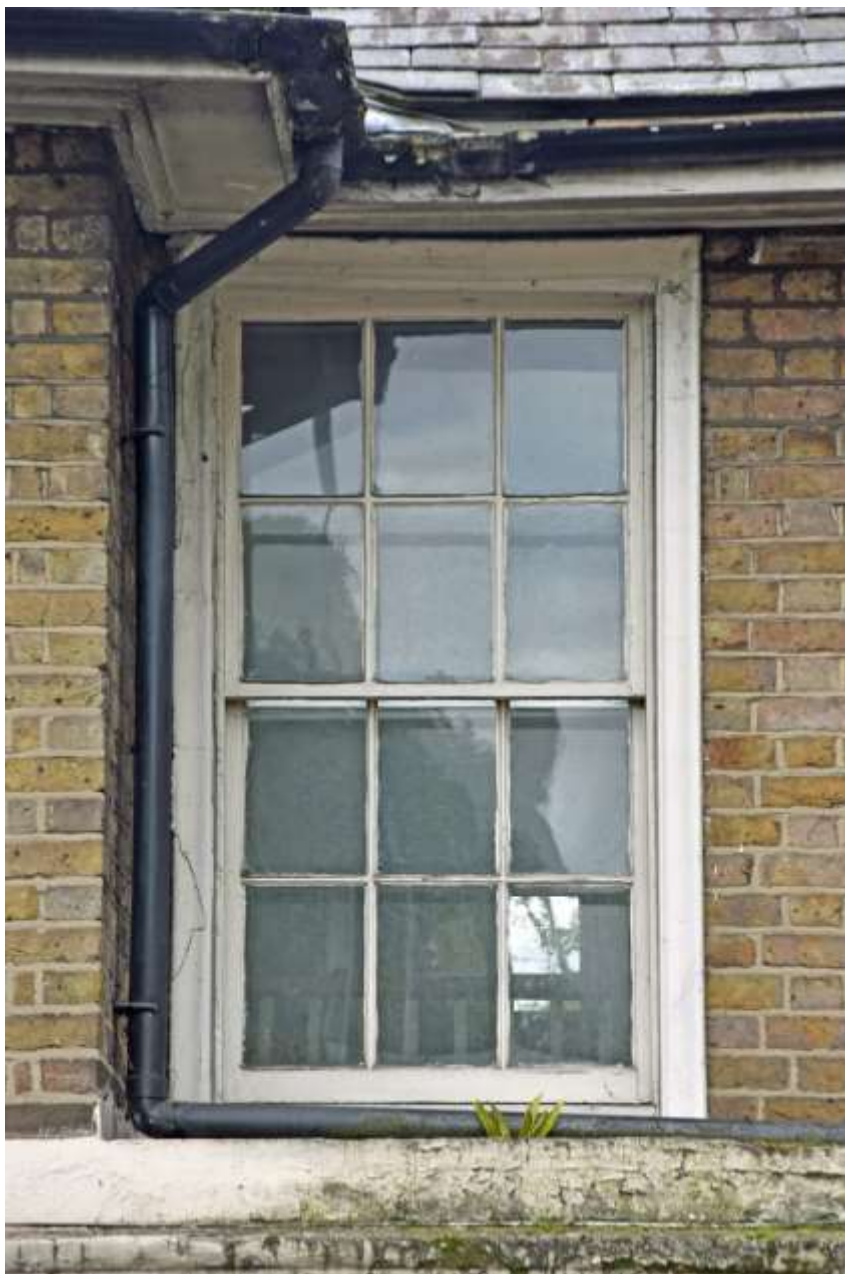
Figure 25: Photograph of the first floor central window on the front façade. Taken 22.10.24.
