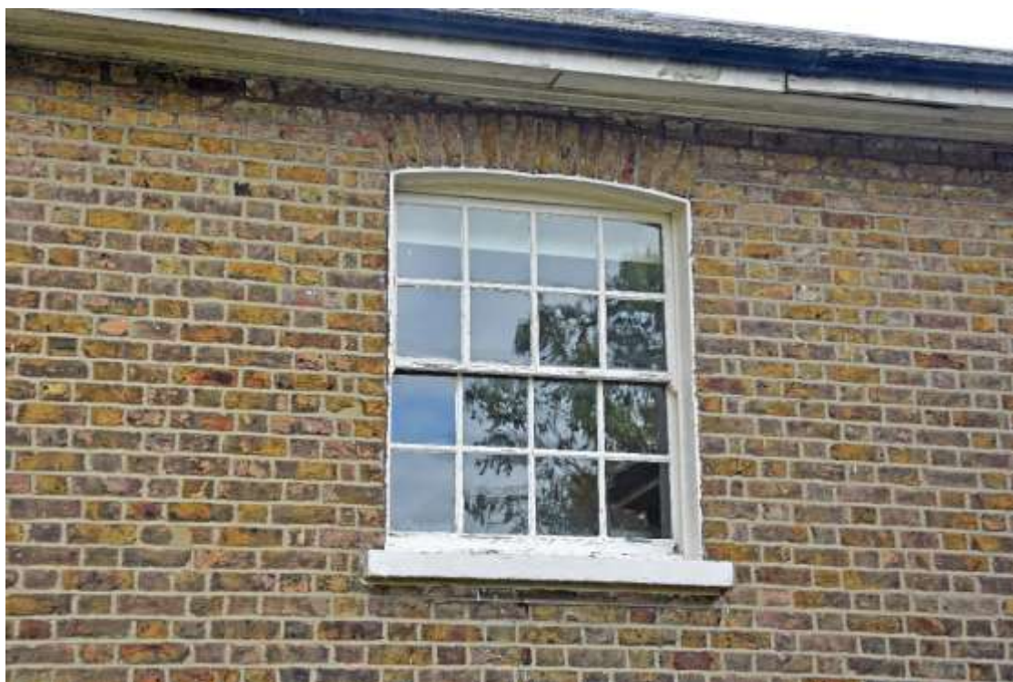
Figure 70: Photograph of Upper left window of rear elevation. Taken 22.10.24.
