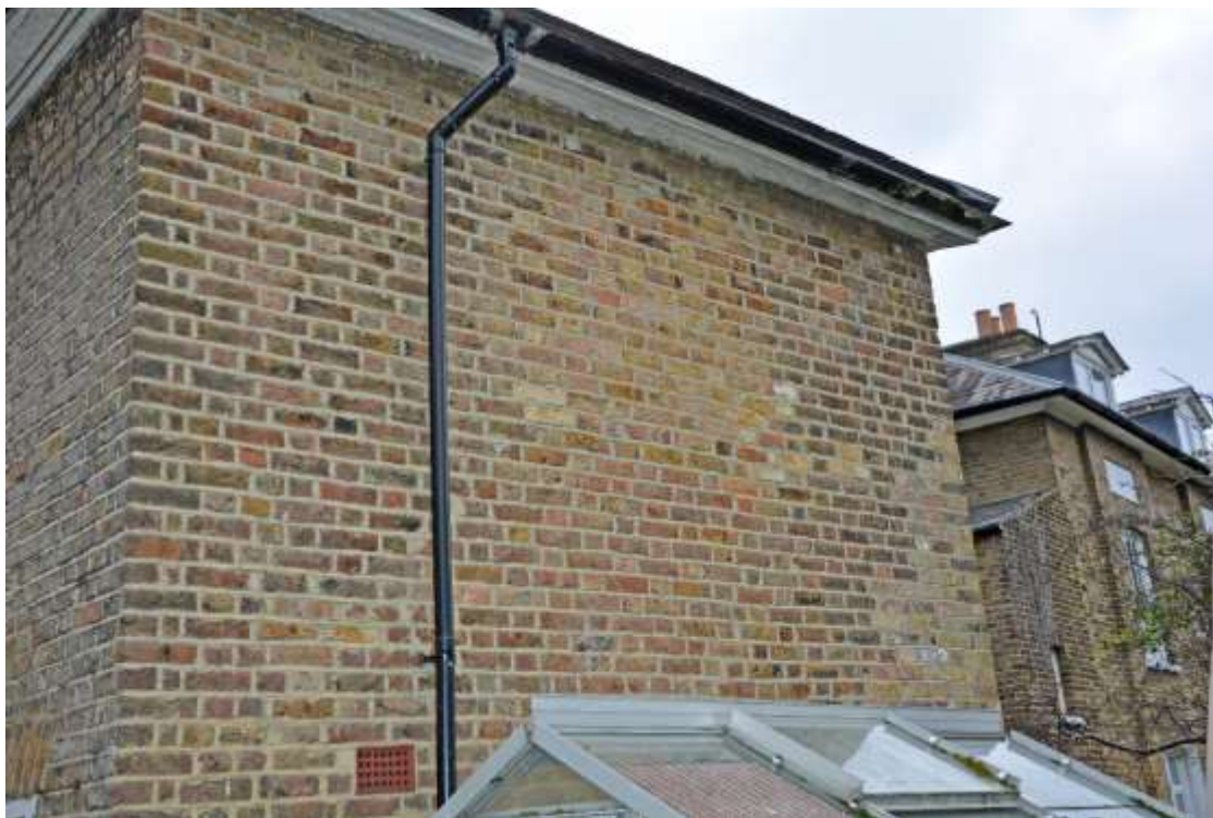
Figure 83: Photograph of the upper part of the rear elevation of the extension, with an area of restored bricks visible in the centre of the first floor. Taken 01.11.24.
