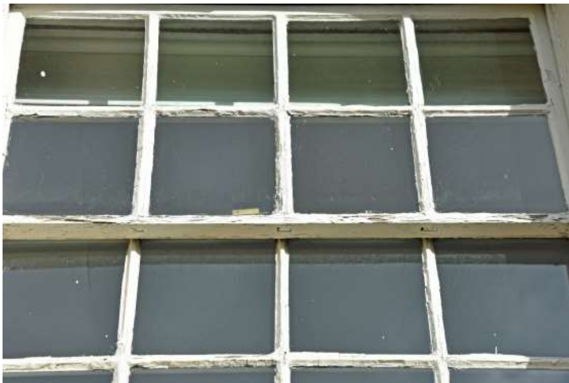
Figure 71: Detail Photograph of Upper Left Window of rear elevation. Taken 22.10.24.
