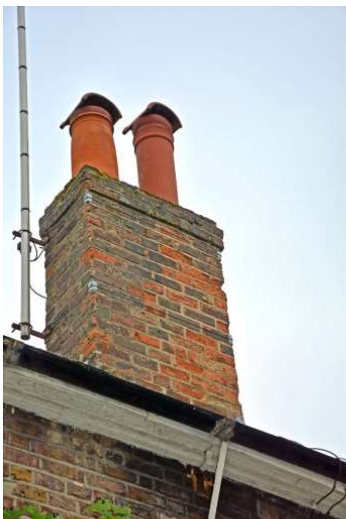
Figure 92: Photograph of the chimney associated with 9a Muswell Hill, southern side elevation. Taken 01.11.24.
