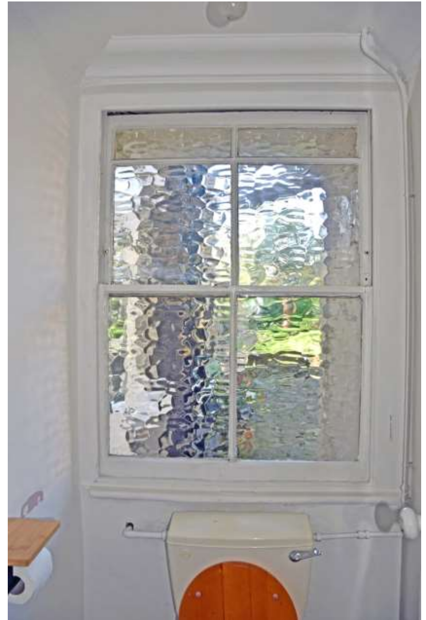
Figure 148b: Detailed photograph of the window in Area F. Taken 22.10.24.
