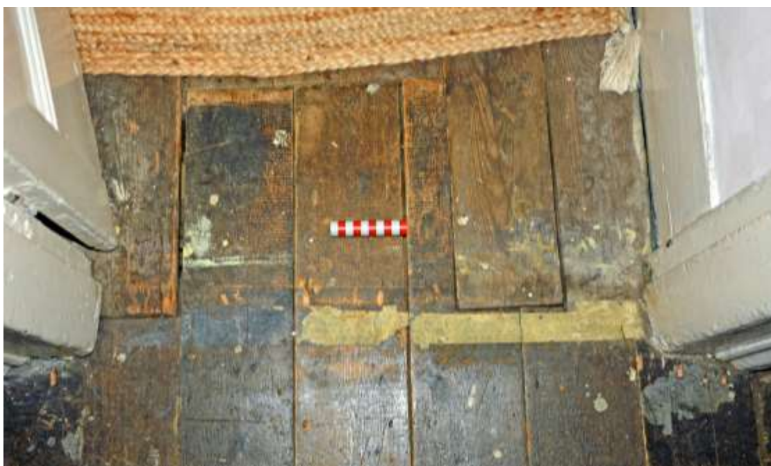
Figure 178: Detail Photograph of flooring within the entrance to Area O. Thinner floorboards visible to the right. Taken 11.12.24.
