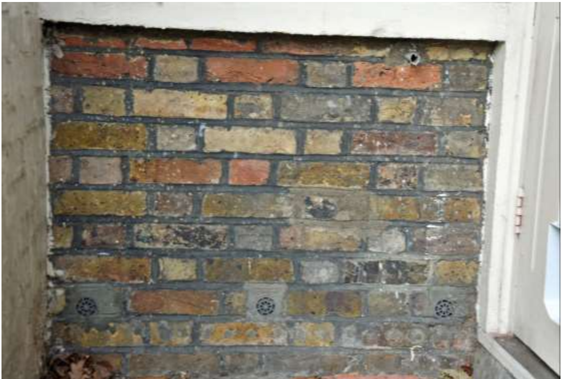
Figure 79: Detail Photograph of the modern brickwork directly underlying the lower central window. Taken 22.10.24.
