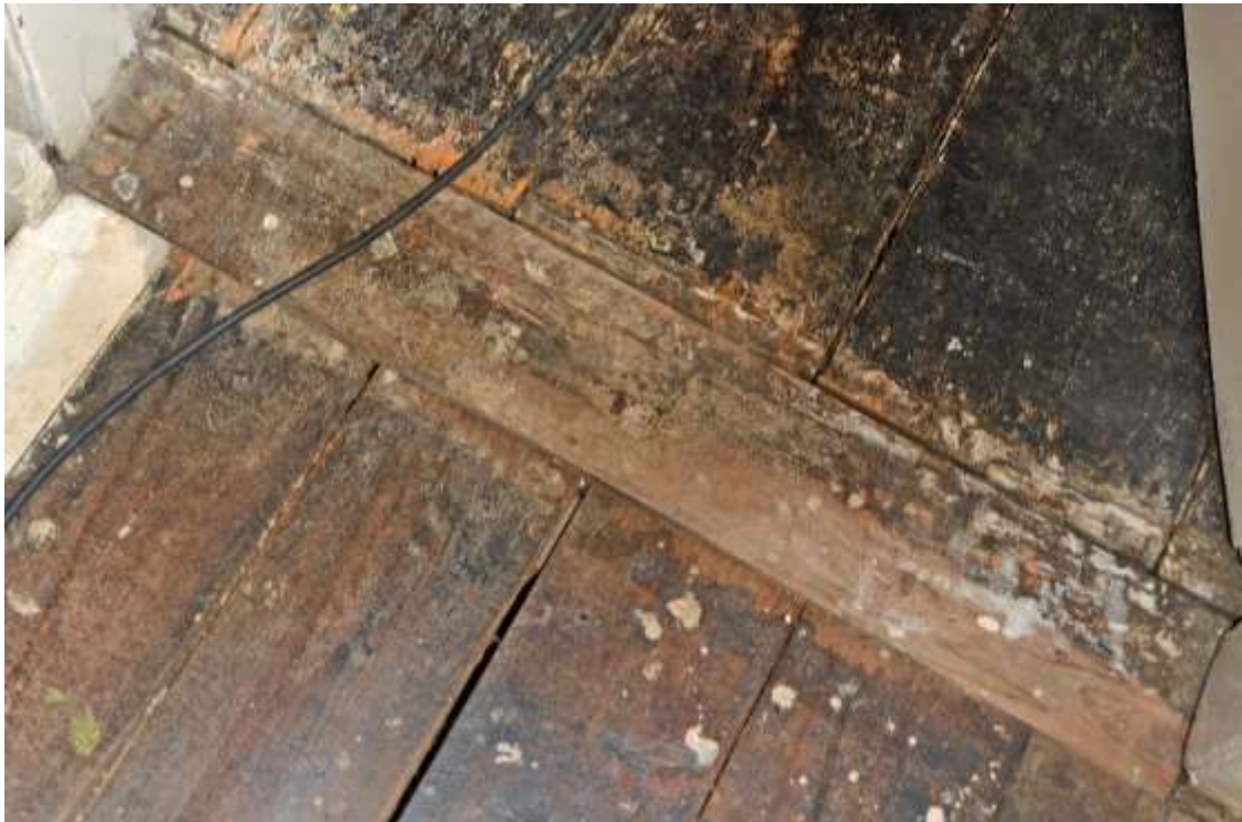
Figure 161: Detail Photograph of entrance to Area L (with wider floorboards top right). Taken 01.11.24.
