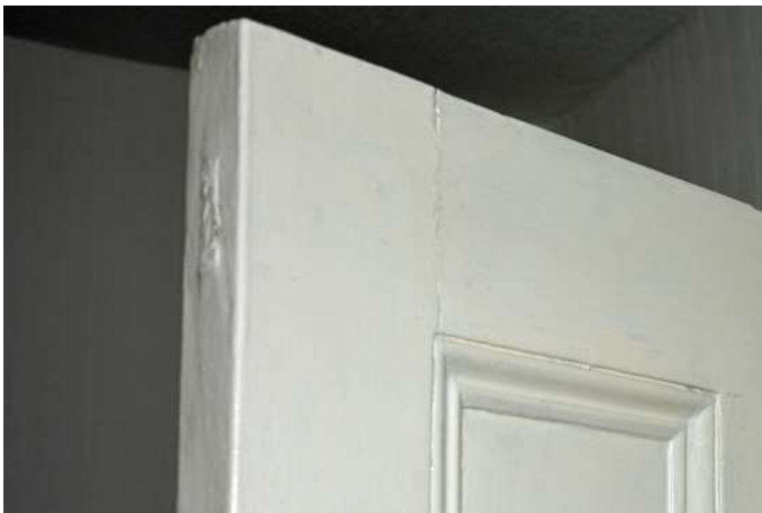
Figure 130: Detail Photograph of mortise and tenon joint within the door of Area C. Taken 11.12.24.
