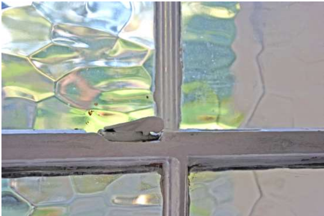
Figure 149: Detail Photograph of 'Fitch' sash fastener in Area F. Taken 22.10.24.
