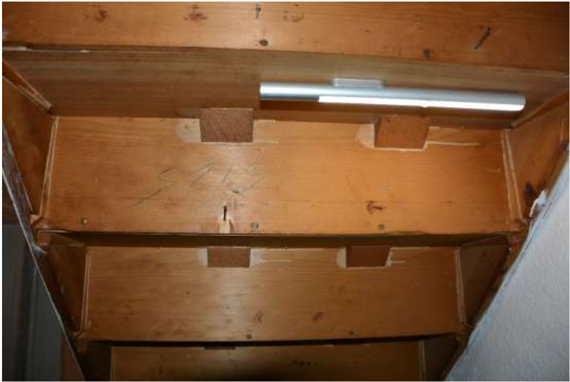
Figure 140: Underside of modern staircase in Area D. Taken 01.11.24.
