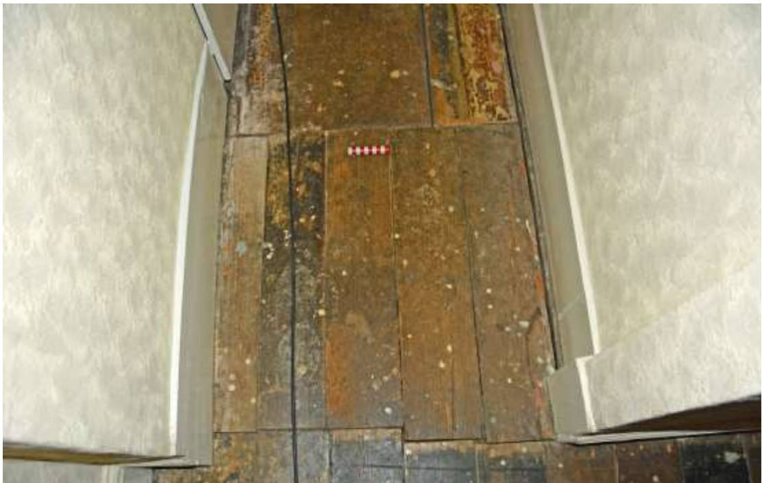
Figure 170: Detail Photograph of flooring in Area M leading to Area N (top). Taken 11.12.24.
