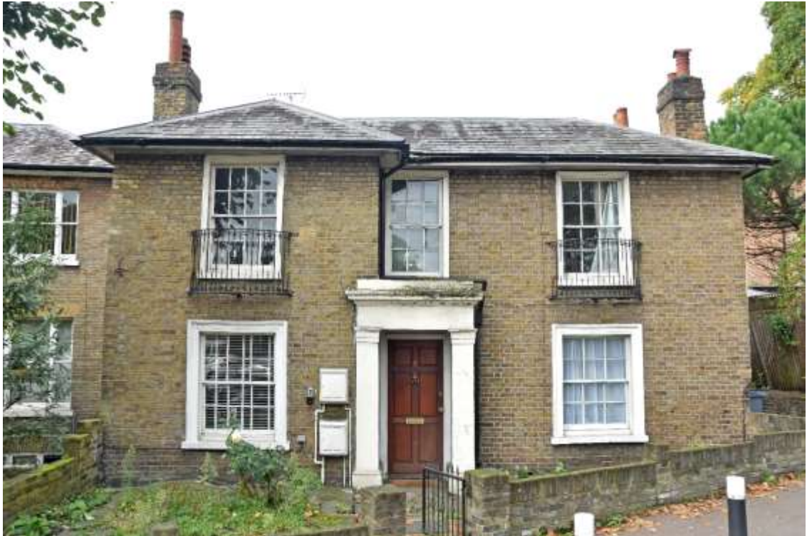
Figure 13: Photograph of Front Elevation of 9 Muswell Hill. Taken 22.10.24. Facing WSW.
