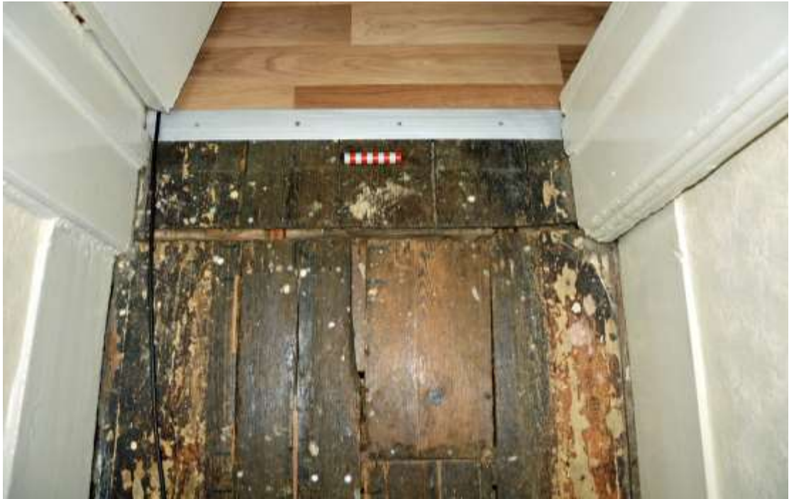
Figure 169: Detail Photograph of flooring between Area M (bottom) and Area N (top). Taken 11.12.24.
