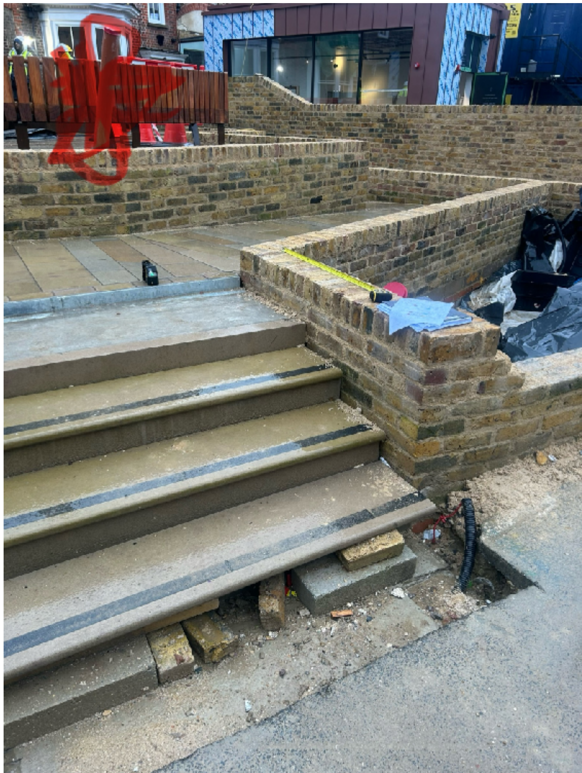
HOLES NOT DRILLED AT TIME OF SURVEY 13/1/26
