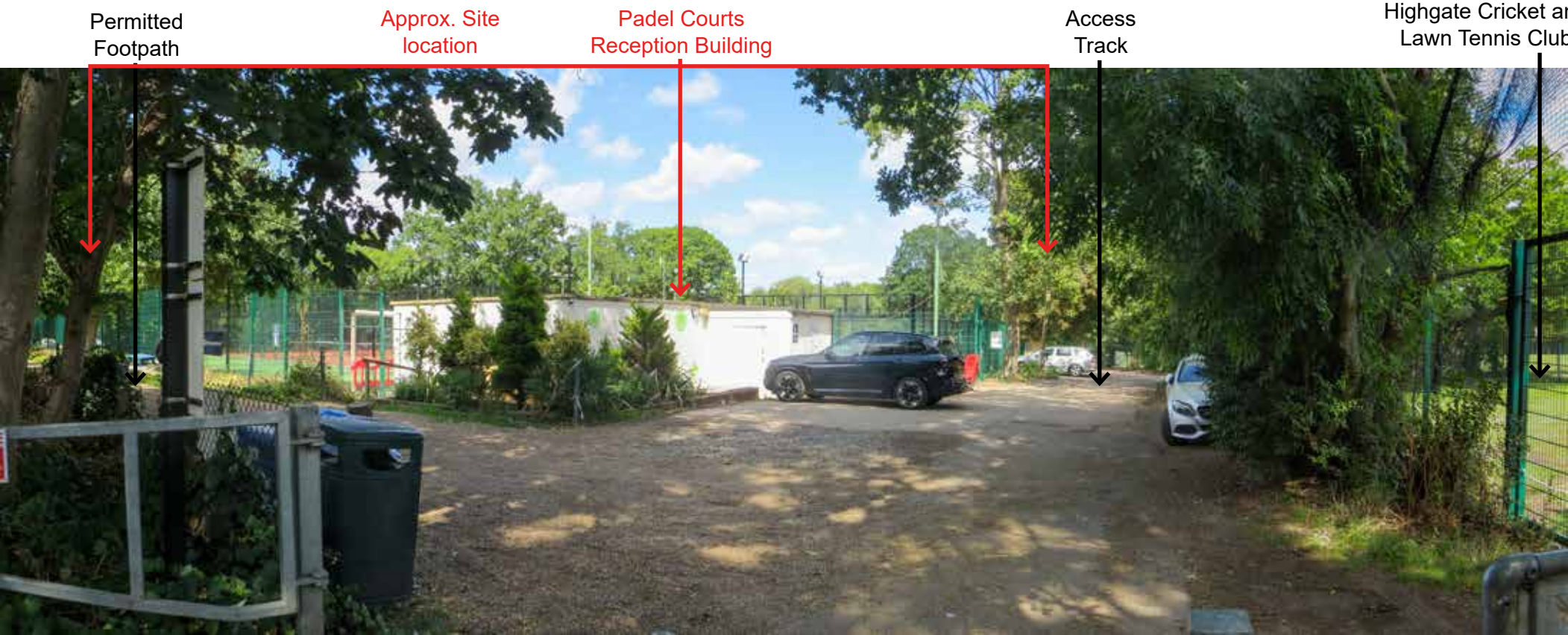
Representative view 2 - taken from Access Track (west)
