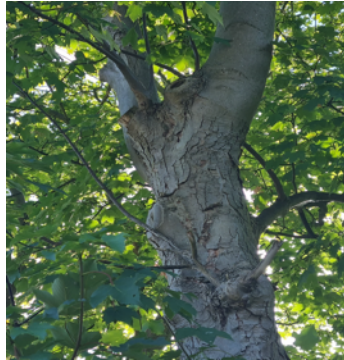
Plate 14: Open and exposed cavity of T2
