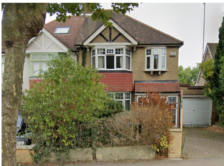
EXISTING SITE PHOTO 16 COPPETTS RD FROM THE ROAD SIDE
