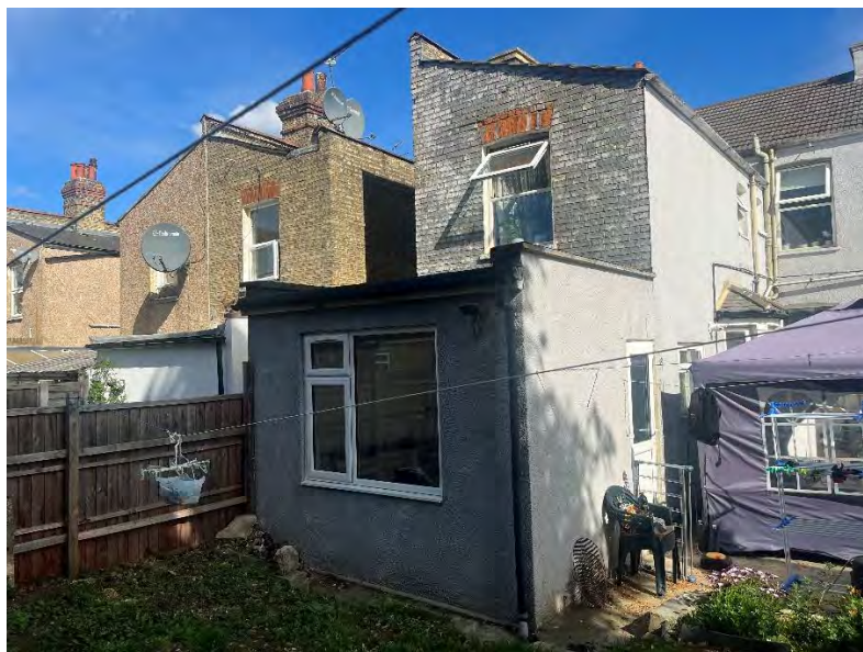
Rear view of nos 1 and 3. The existing single storey rear extension is to be retained.
