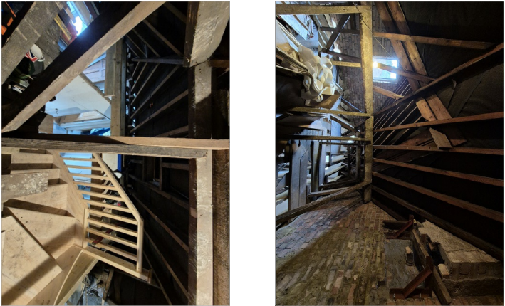
EXISTING ATTIC & STAIRCASE
