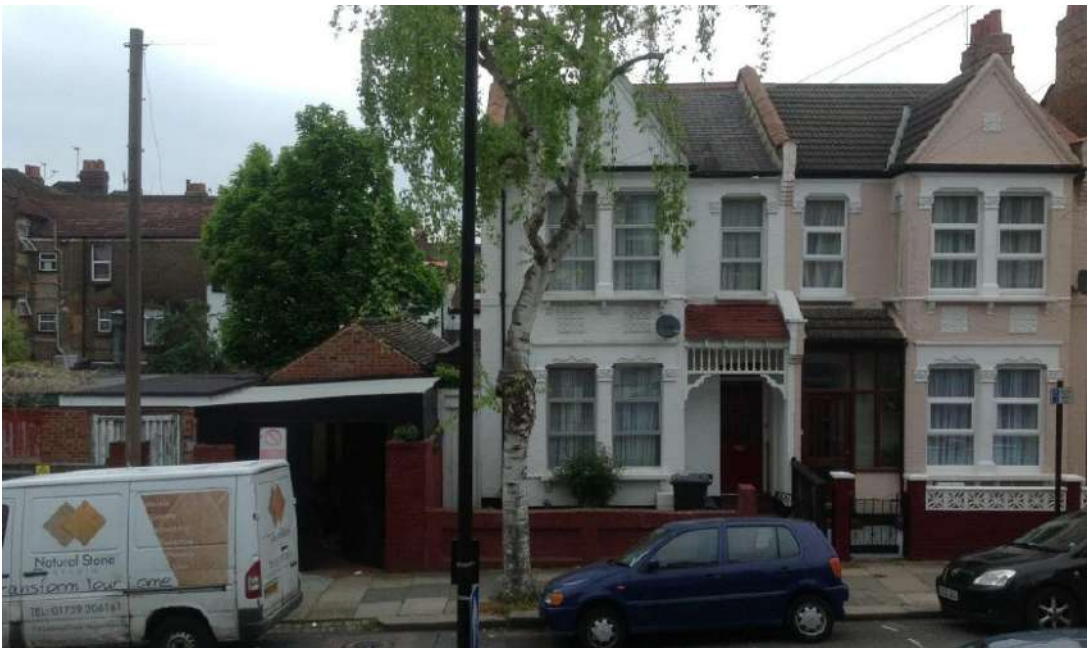
Previous Existing Garages
