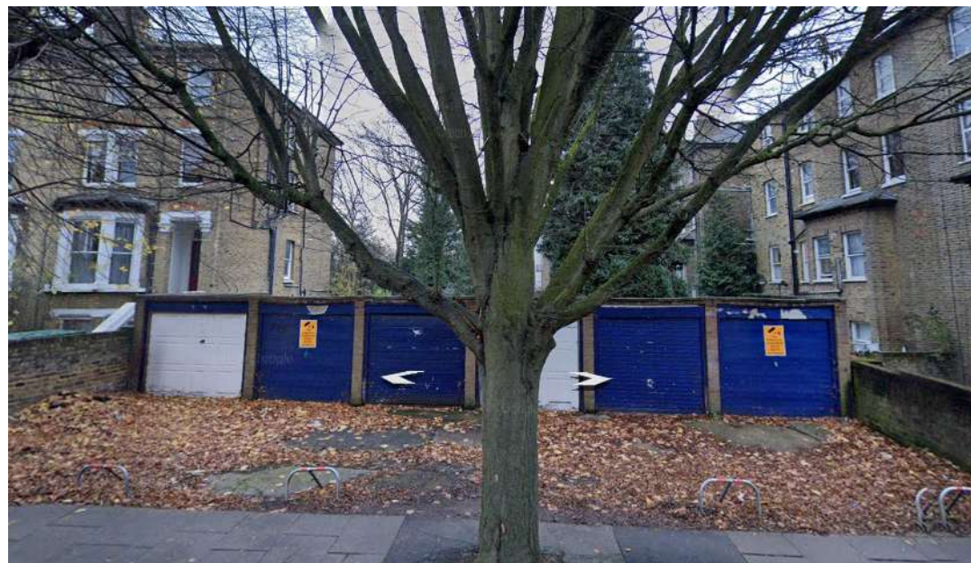
Previous Existing Garages
