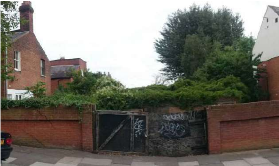
Previous Existing Garages
