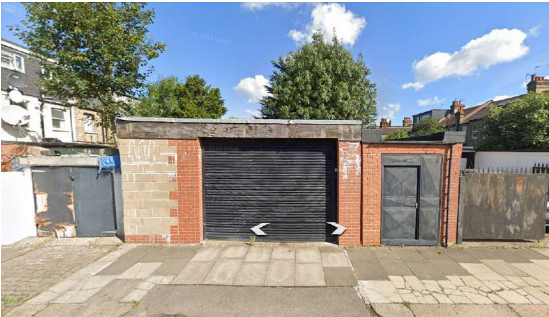
Previous Existing Garages
