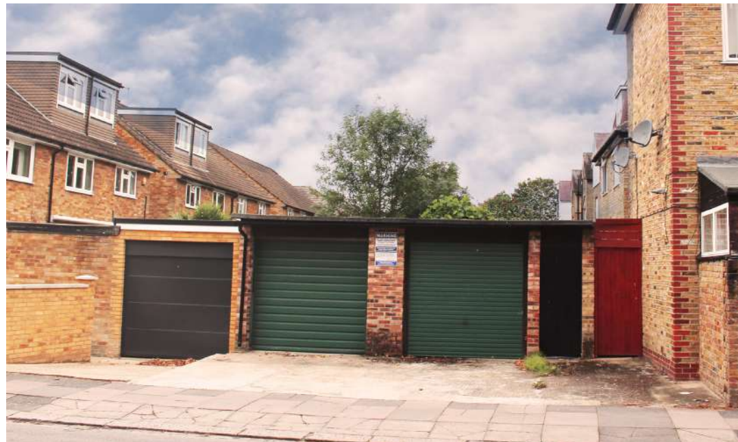
Previous Existing Garages
