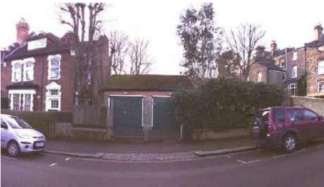
Previous Existing Garages
