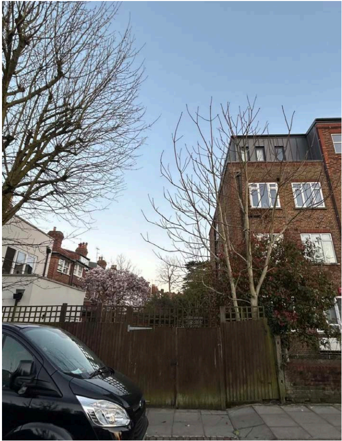
SITE FROM CHURCH ROAD
