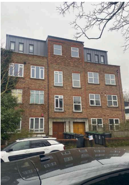
3-5 CHURCH ROAD USE OF FLAT ROOF AND BRICK FACADE NEXT TO SITE
