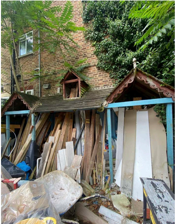
SHED TO BE DEMOLISHED
