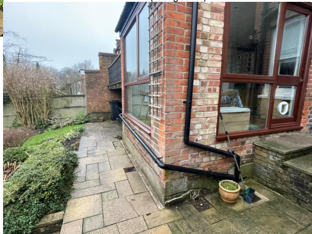
Photograph 6 – Rear Garden (Facing South)
