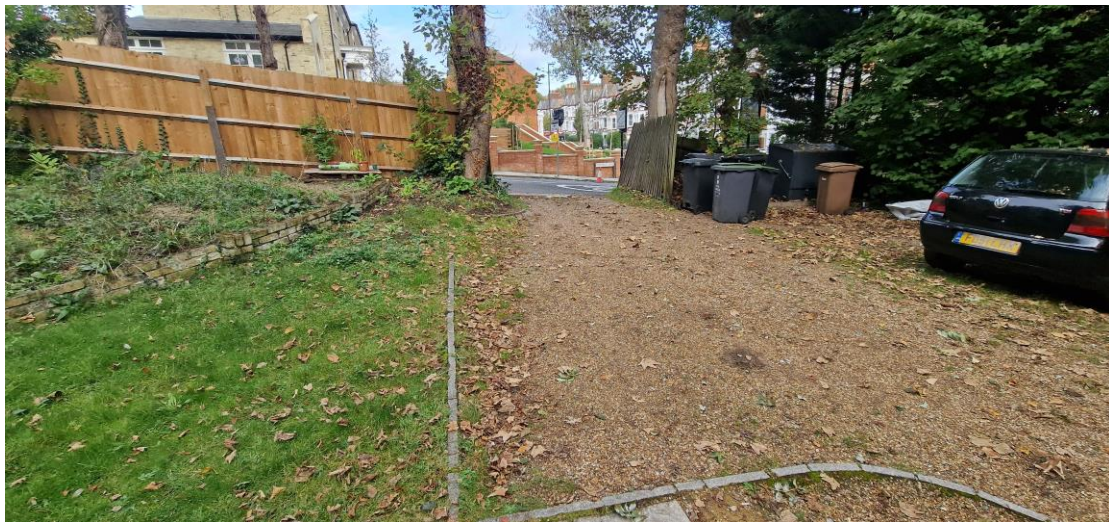
Image of cracked and swollen grounds.
