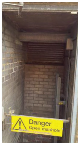
Photo 12 (24/04/2025): Structure 2 access tunnel (Structure 3 had an identical appearance). No bat evidence in above-ground structure.
