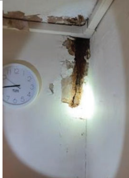
Photo 6 (24/04/2025): Building 1: internal feature - leading to wall cavity. No bat evidence visible within or outside the feature.
