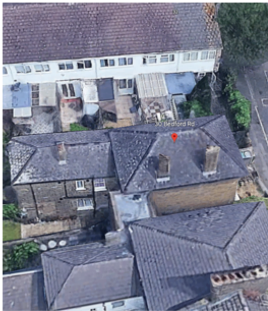
Roof Side Elevation (South)
