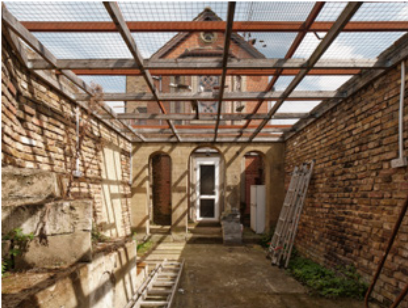
Freestanding arches to be enclosed against
