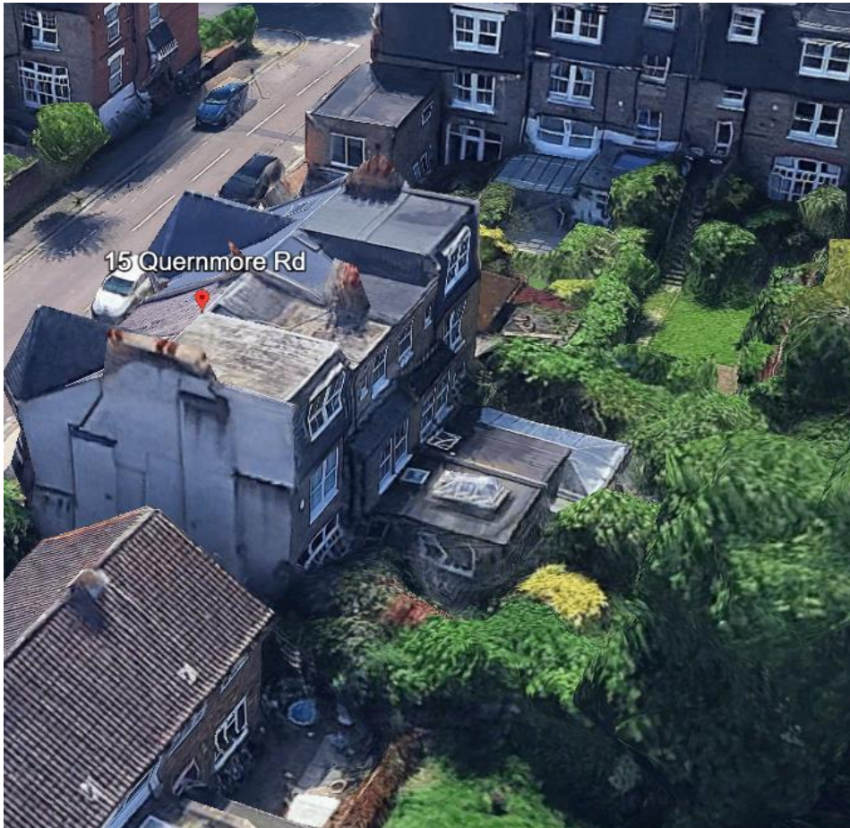
Photograph 2 Showing the existing rear addition to 15 Quernmore Road.
