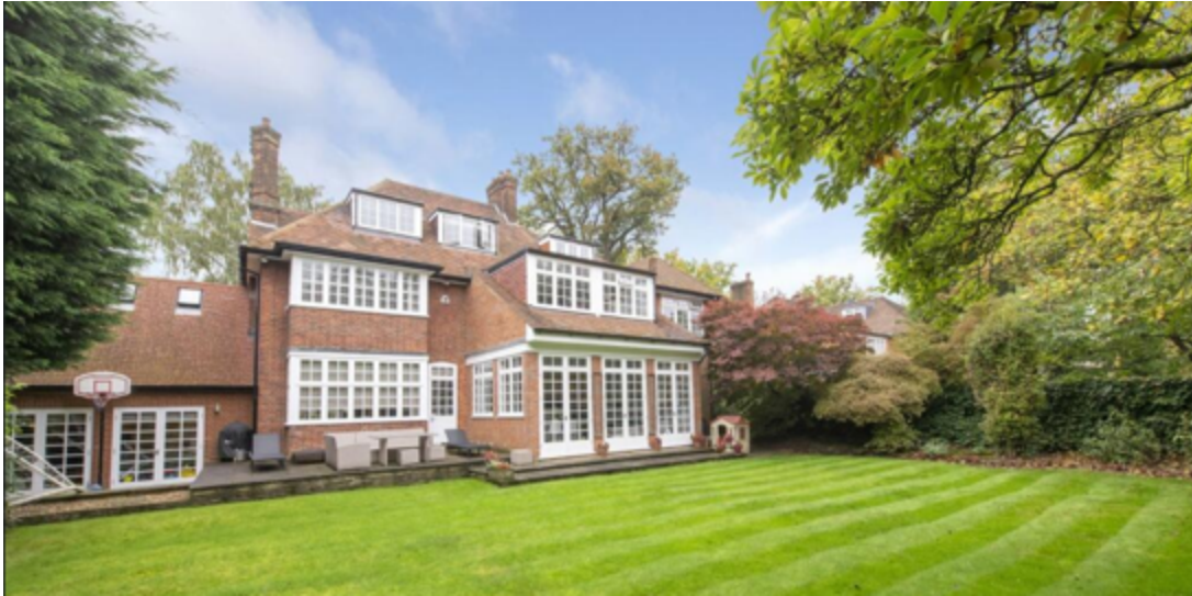
Fig.3 – Image of the rear elevation.
