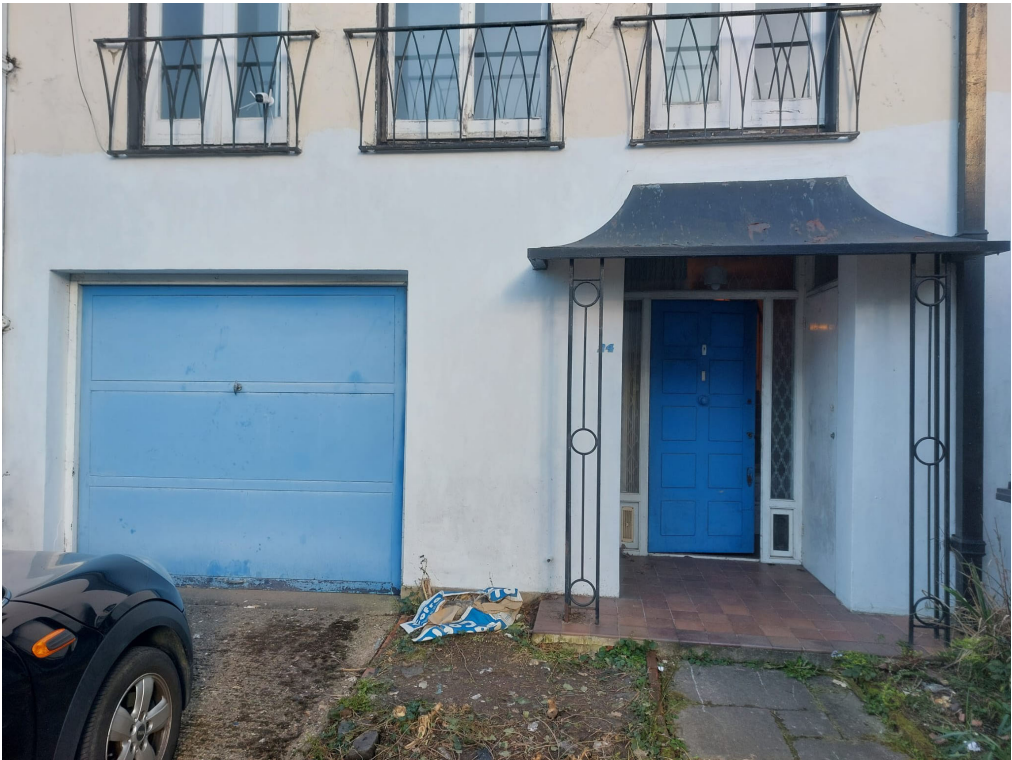
Picture 03: Front View
