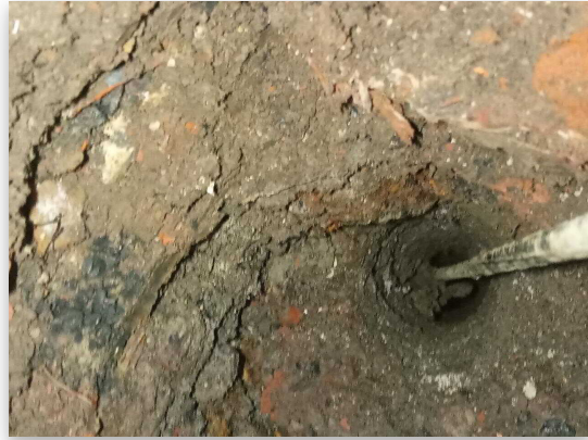
Fig 2.2: Trial Hole 2 Footing
