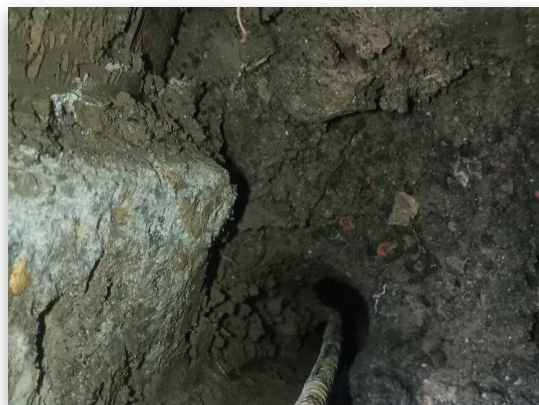
Fig 1.2: Trial Hole 1 Footing
