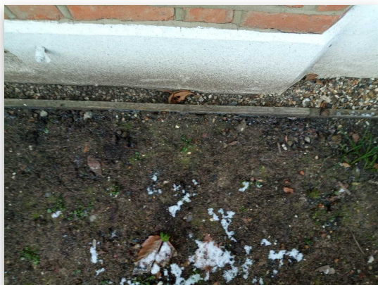
Fig 1.1: Trial Hole 1 Location
