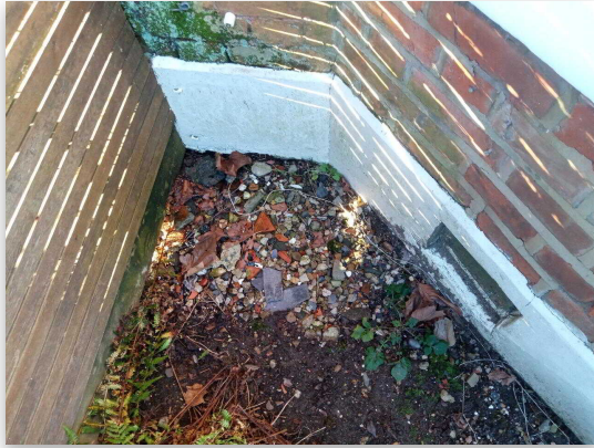
Fig 2.1: Trial Hole 2 Location
