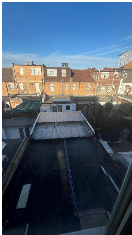
Photos taken in 2026 by the site survey
