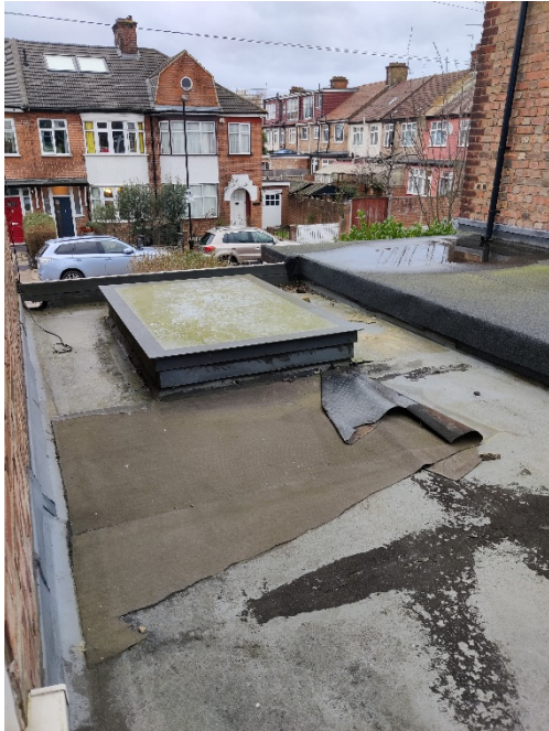
99 Stirling Rd Front Garage roof view from the property. We can see No 97 Garage sits higher
