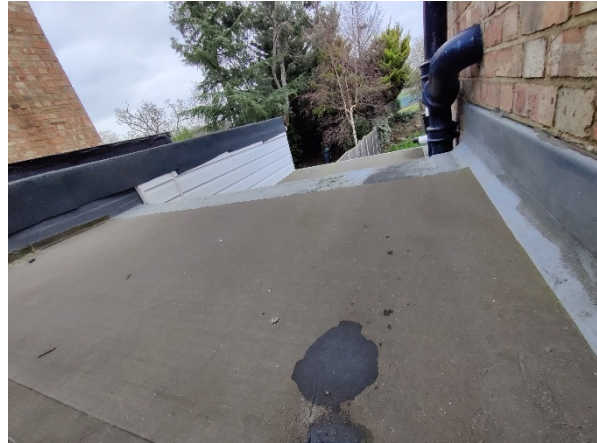
99 Stirling Rd Rear Garage roof view from the property. No 97-roof height is considerably higher due to the reduced height we are trying to mitigate
