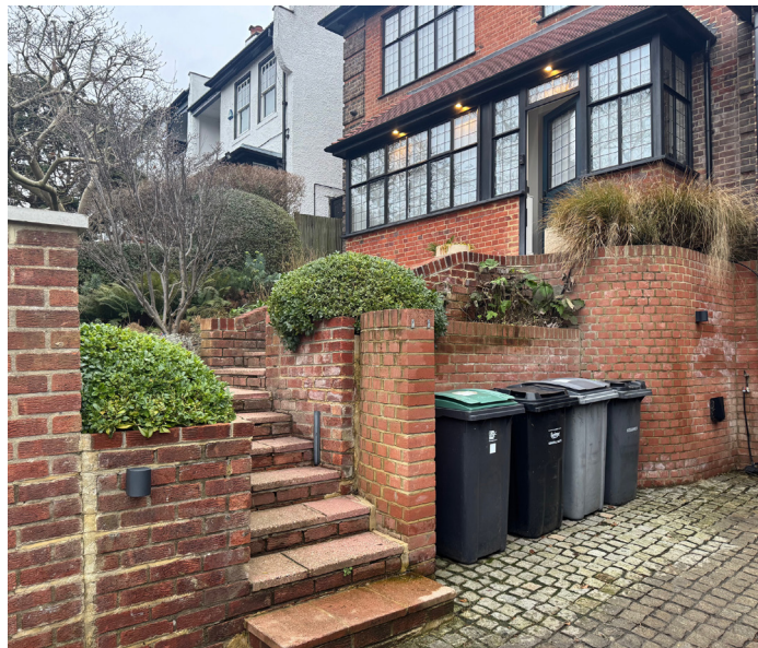
PHOTO 02 - Existing access to the front door, showing entry to steps via the driveway with first steps located on the drive
