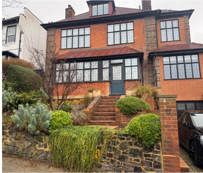
PHOTO 01 - Overall view of the existing front garden at 77 Cholmeley Crescent, N6 5EX
