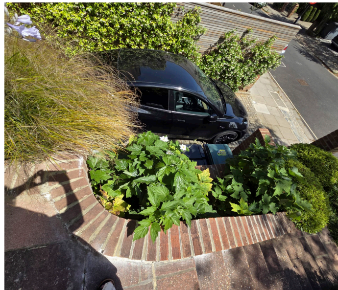
PHOTO 04 - Existing upper landing at top of steps, showing unprotected level change to the driveway below
