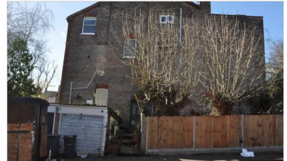
Street Elevation on Clifton Road prior to works
