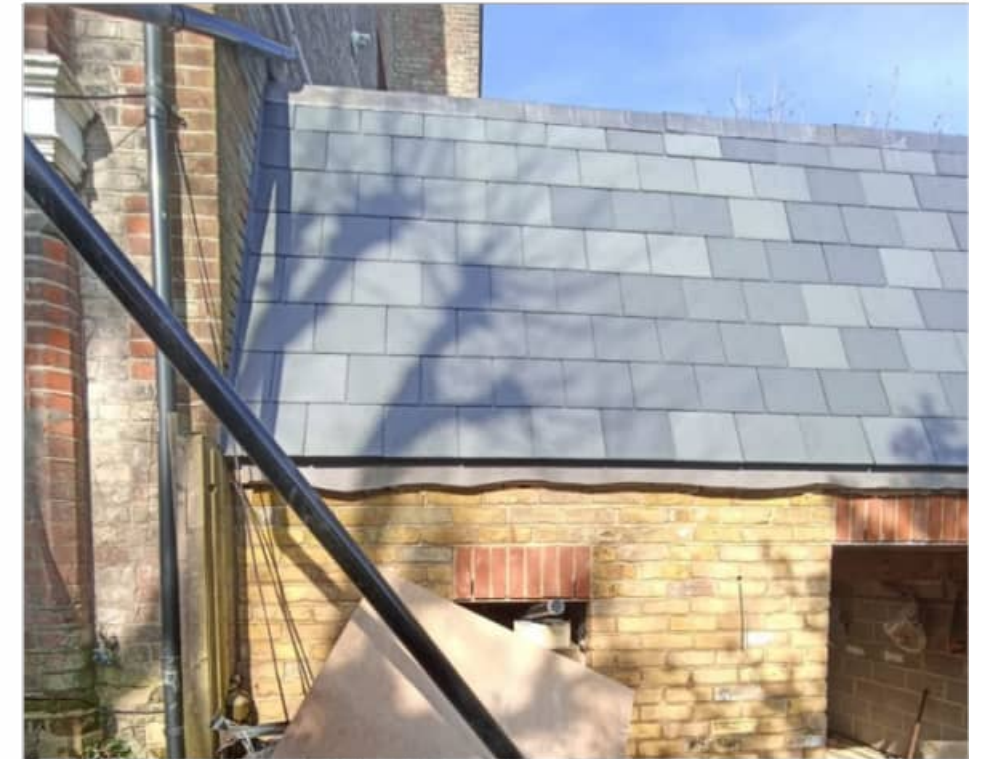
Partially constructed side extension
