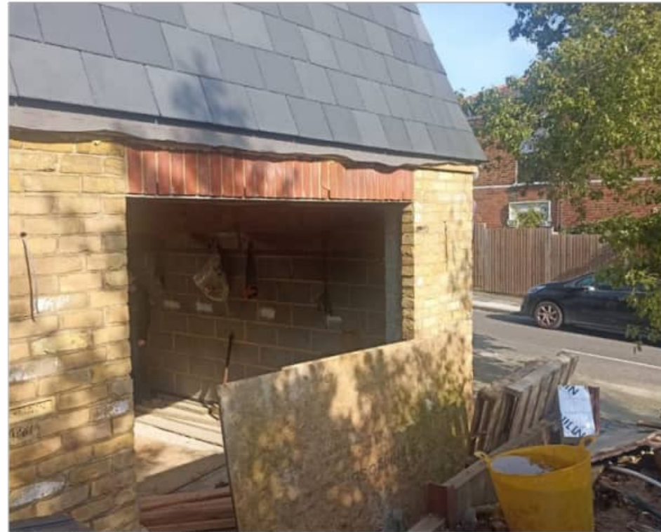
Partially constructed side extension
