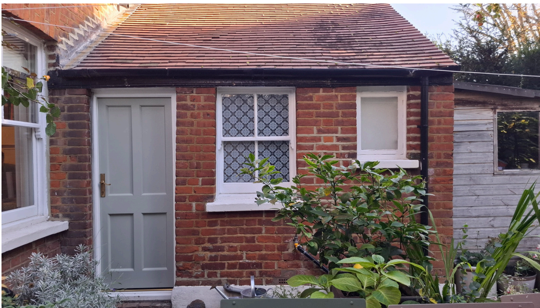
West side facade of existing extension.
