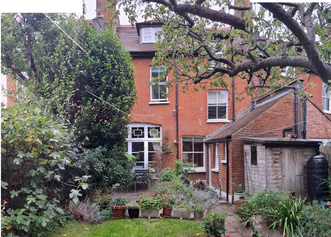
Close-up view of the existing Garden extension. The extension is mirrored on No49 side
