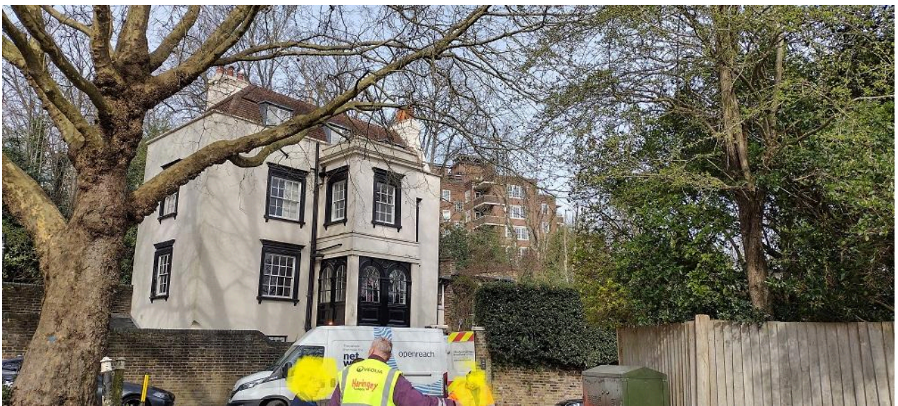
Dowding House viewed from the junction of Jackson's Lane and Southwood Lawn Road, with Bank Point Cottage (Grade: II, List Entry Number: 1189054) and its garden walls (Grade: II, List Entry Number: 1358859) in the foreground.
