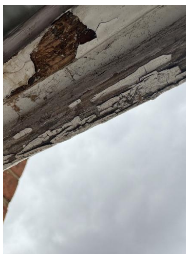
Poor condition of timber double hung sashes
