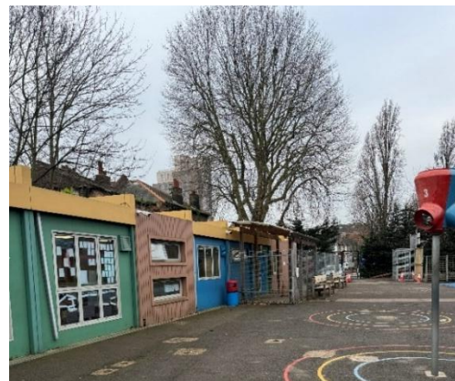
Front Elevation of Block C
