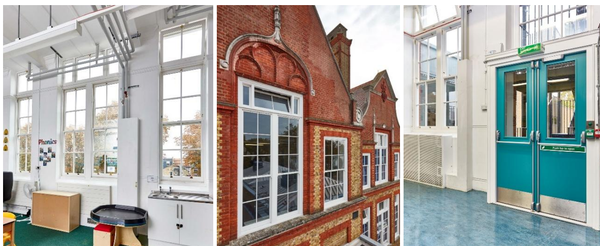
Interior and exterior photos of the double-glazed sash windows at Riversdale Primary
