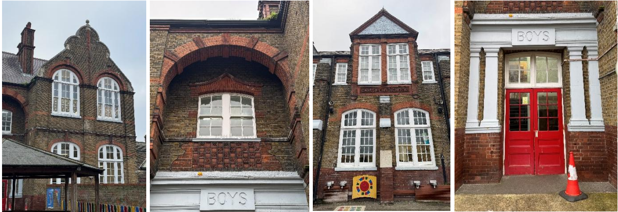
Block Bay 7 gable end, Bay 6 window detail, Bay 4 plaster tympanum and Bay 6 Boys entrance
