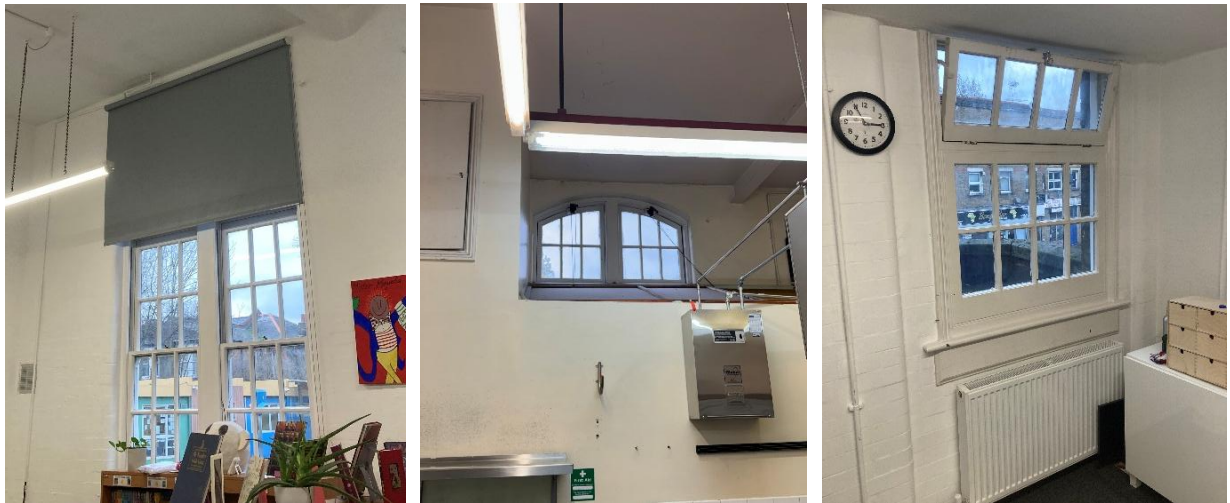
Photos showing bottom hung windows with blinds, high level slopes and opening past reveals.
