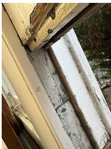
Poor condition of timber double hung sashes
