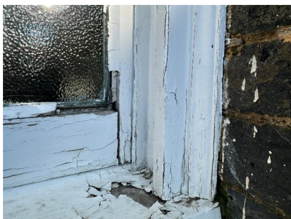
Poor condition of timber double hung sashes
