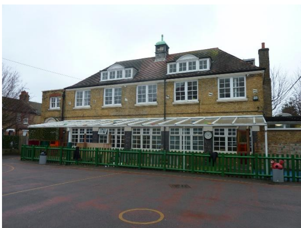
Block C front façade with lean to roof
