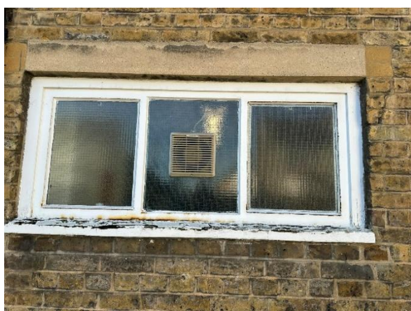
Poor condition of metal casements in timber frames.
