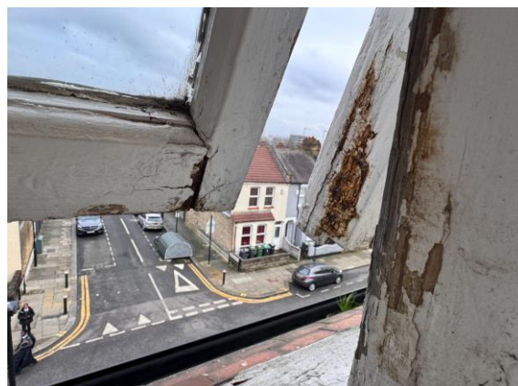
Poor condition of timber casement sashes
