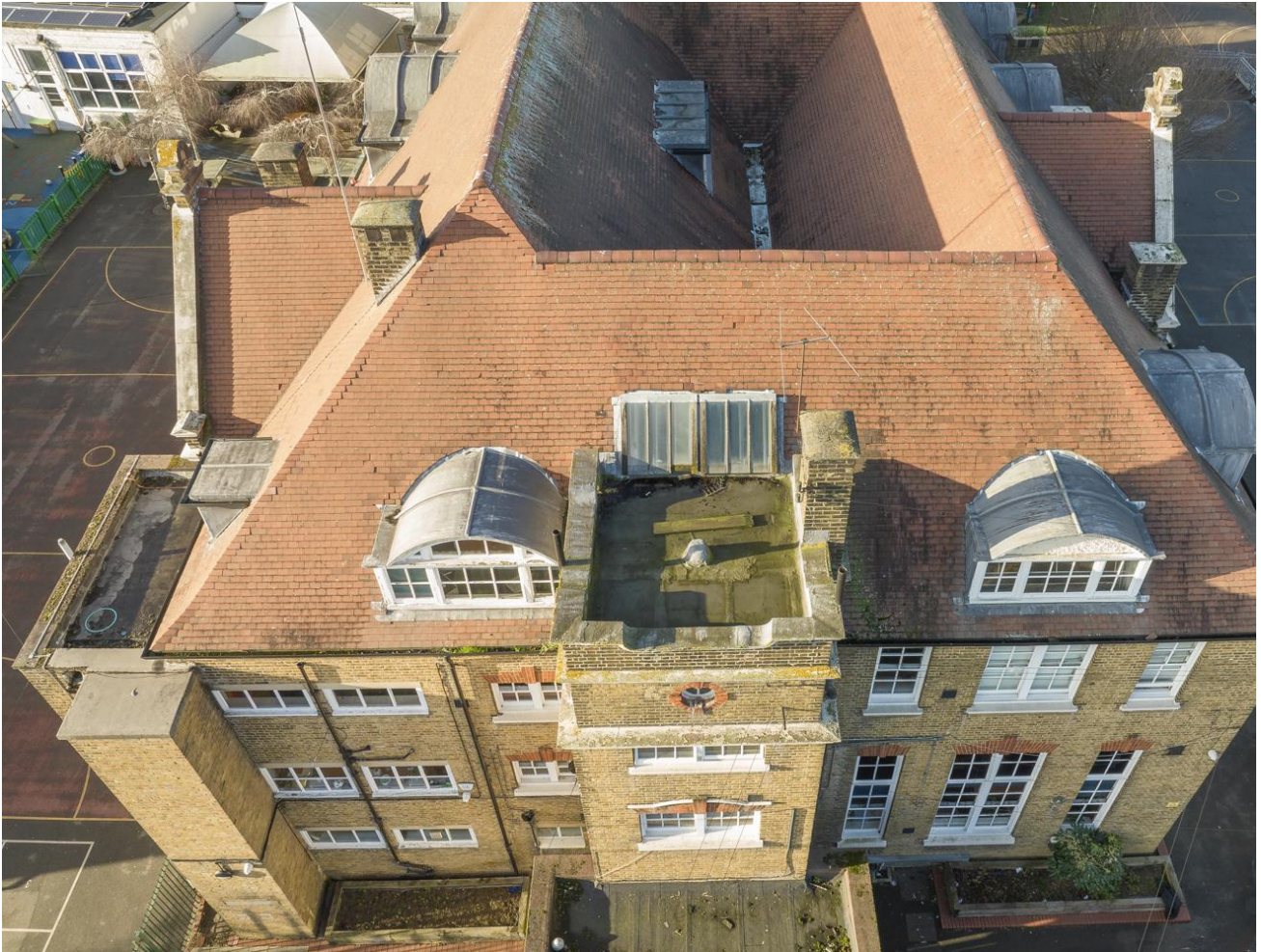
Main roof- Block A
