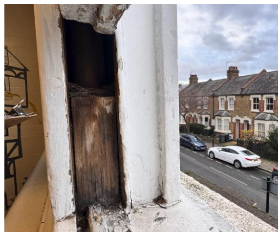
Poor condition of timber casement sashes
