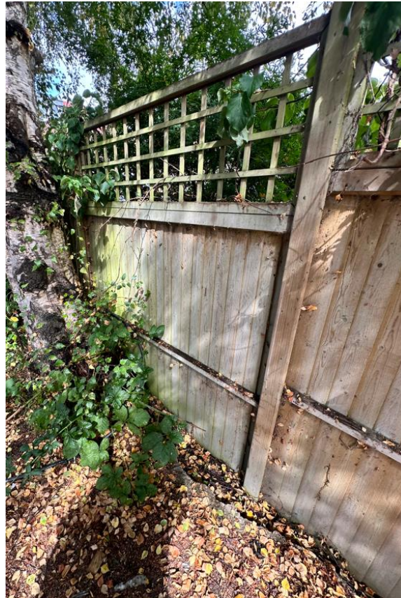
Figure 4: Photo of existing garden fence
