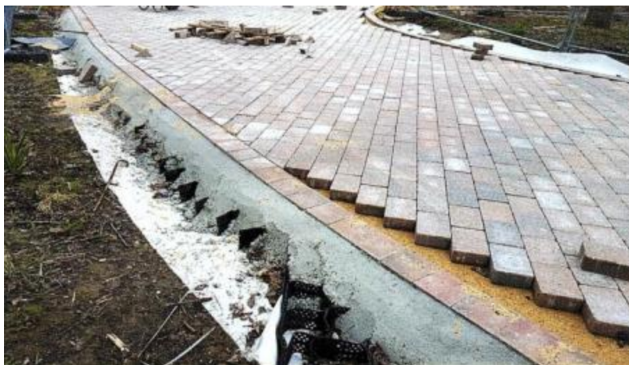
Extract 4. Concrete edge
