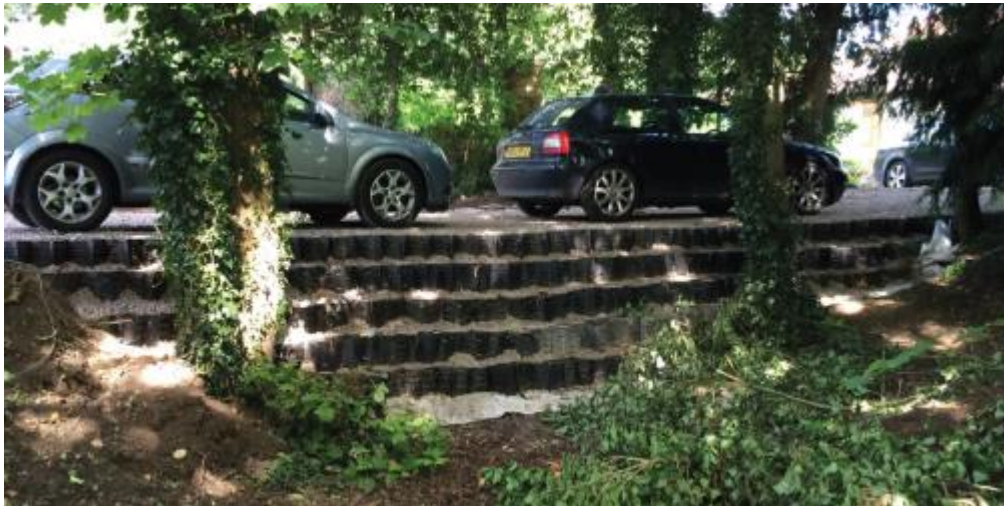
Extract 8 - stacked Cellular Confinement System can be used to increase ground levels
