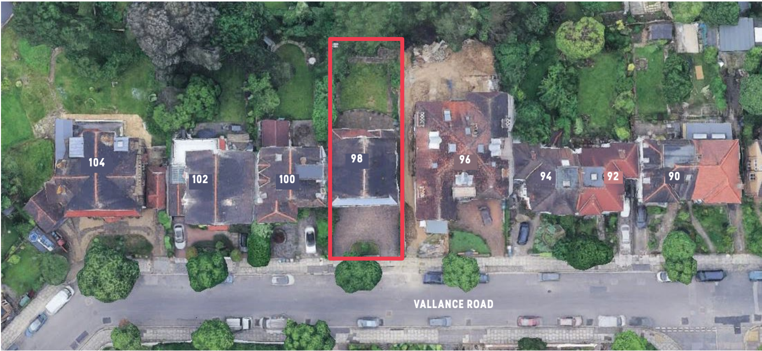
SITE AERIAL Aerial plan view of Vallance Road (outlined in the red). The amount of extension and redevelopment of the neighbouring properties can be observed clearly from this viewpoint.
