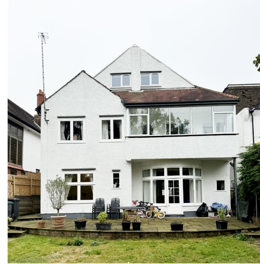
REAR OF PROPERTY North Elevation (facing garden)
