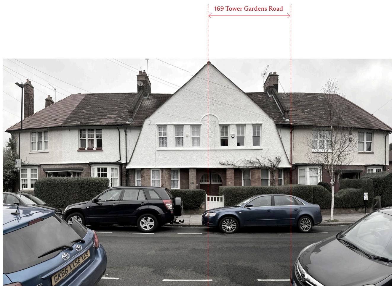
Existing Street View
