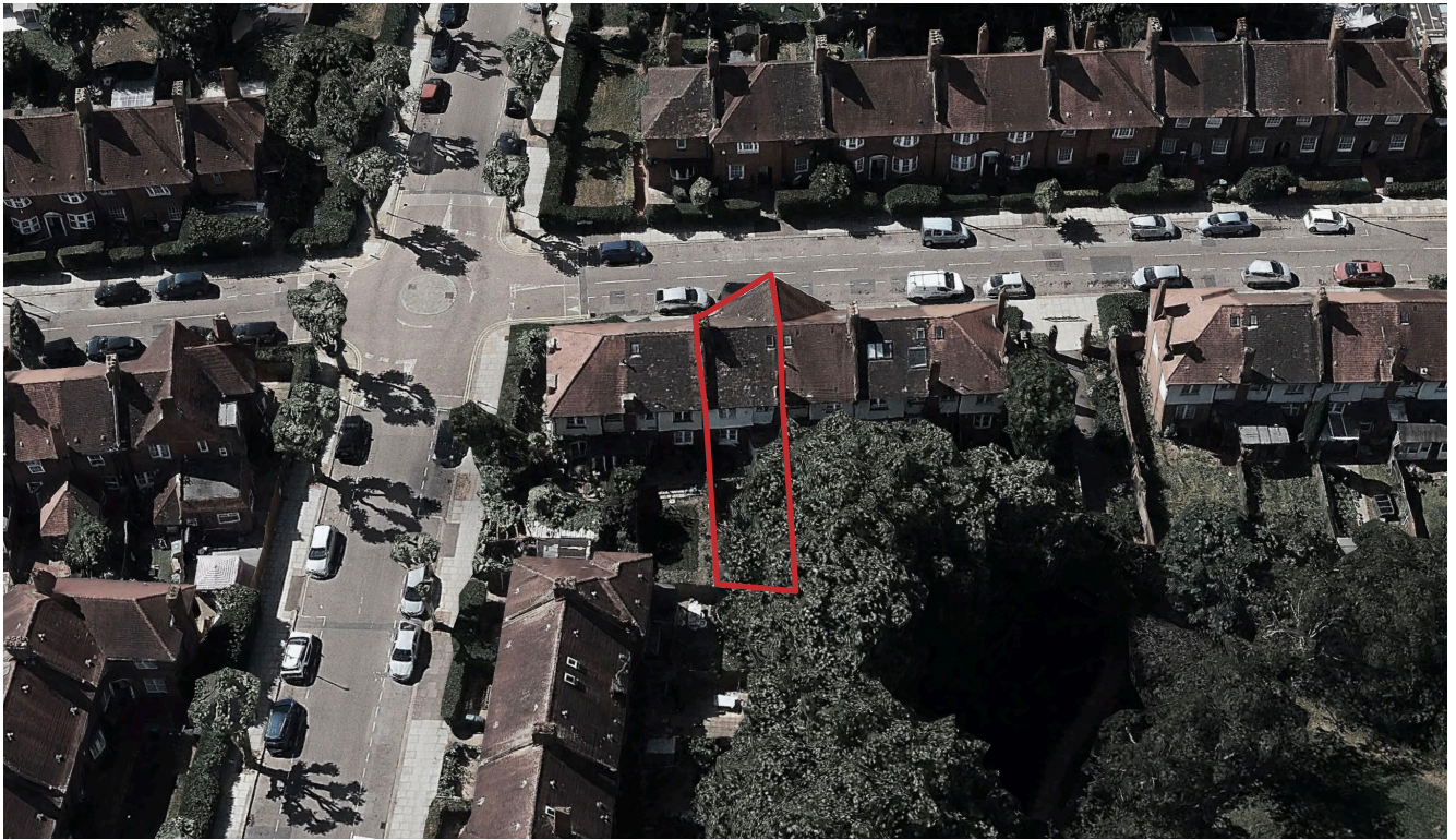
Aerial view from north
