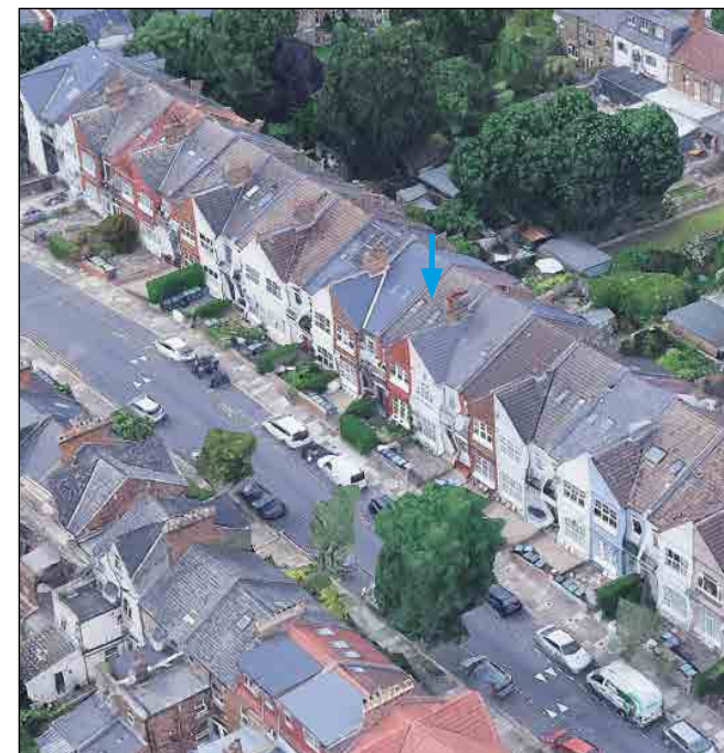
FIGURE 09 Aerial view of existing front facade
