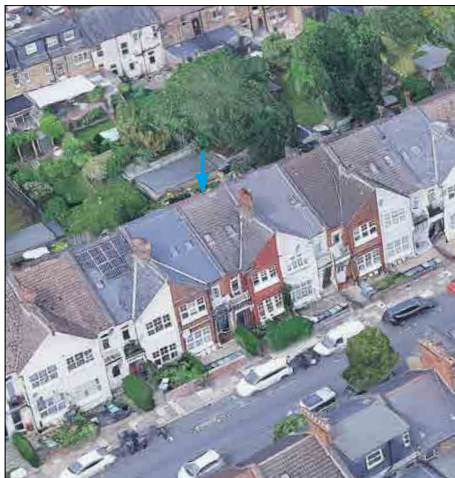
FIGURE 08 Aerial view of existing front facade
