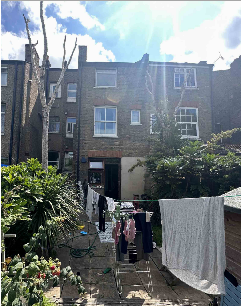
FIGURE 12 Extended view of the existing rear facade from the rear garden.
